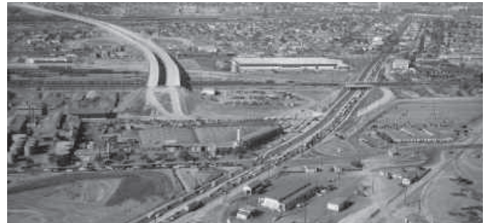
When State Route 7 (I-710) was built in the 1950’s, there was still a great deal of agriculture and open space in the surrounding area.
