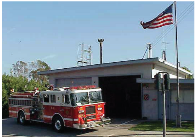
Fire Station No. 4 in the city of Vernon would require relocation under both I-710 build alternatives.
