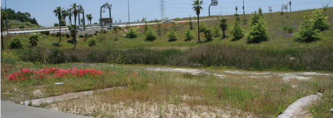
A bioswale storm water runoff treatment feature.
