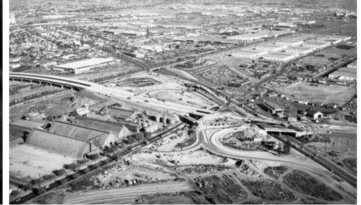
Central Manufacturing District with I-710 under construction in foreground, 1956 (source: Kelly-Holiday Collection of Negatives and Photographs, Los Angeles Public Library)
