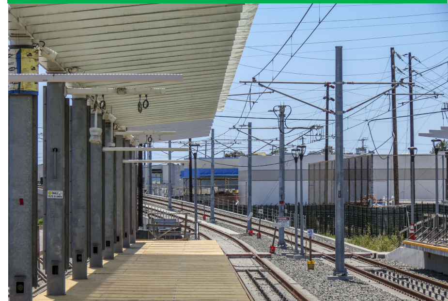
Station platform under construction
