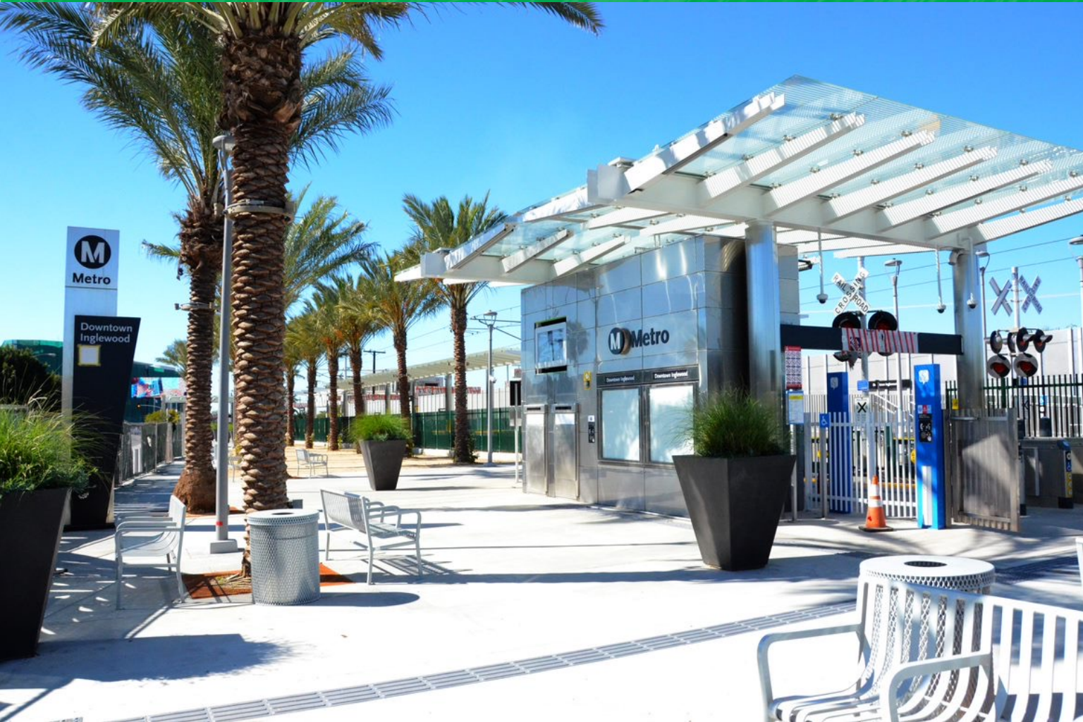
Station pylon, TVM canopy, and plaza
