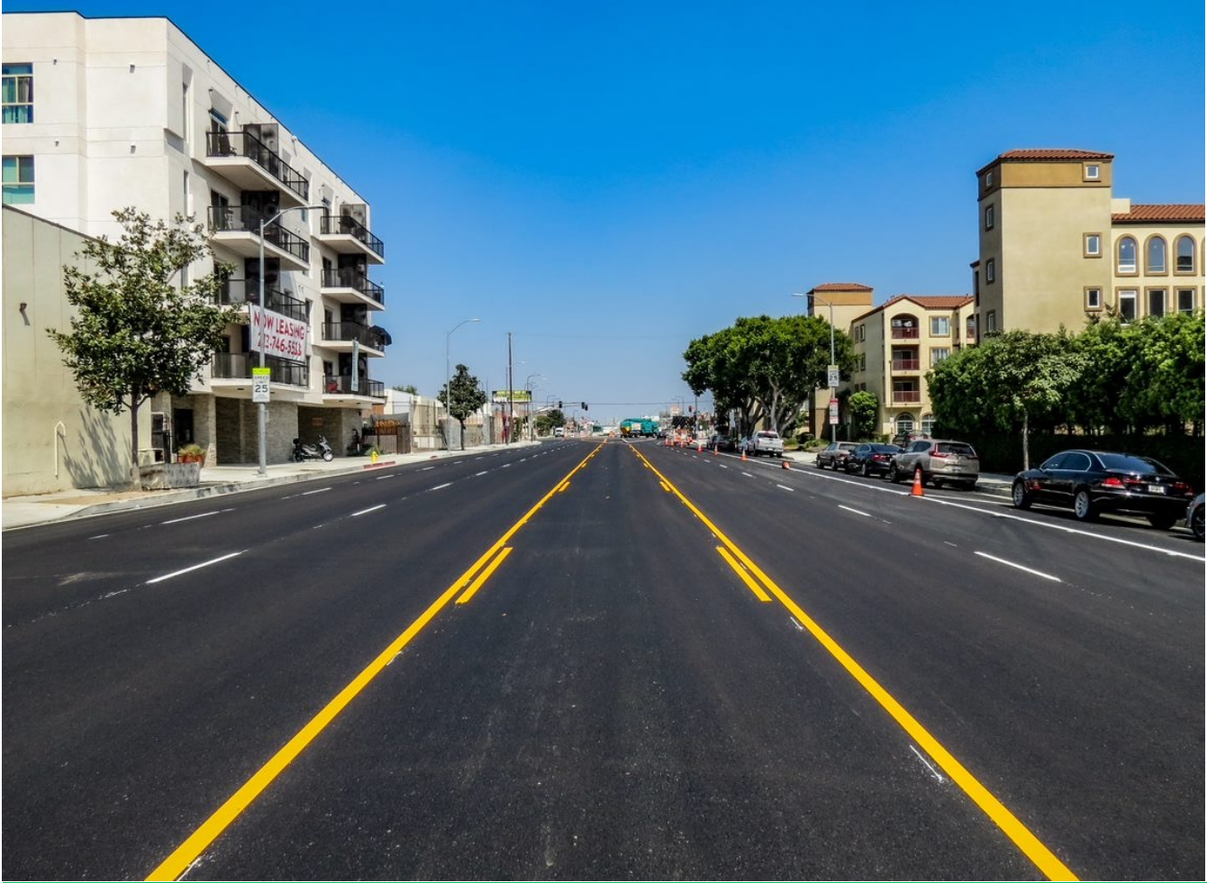
Completed Crenshaw street restoration
