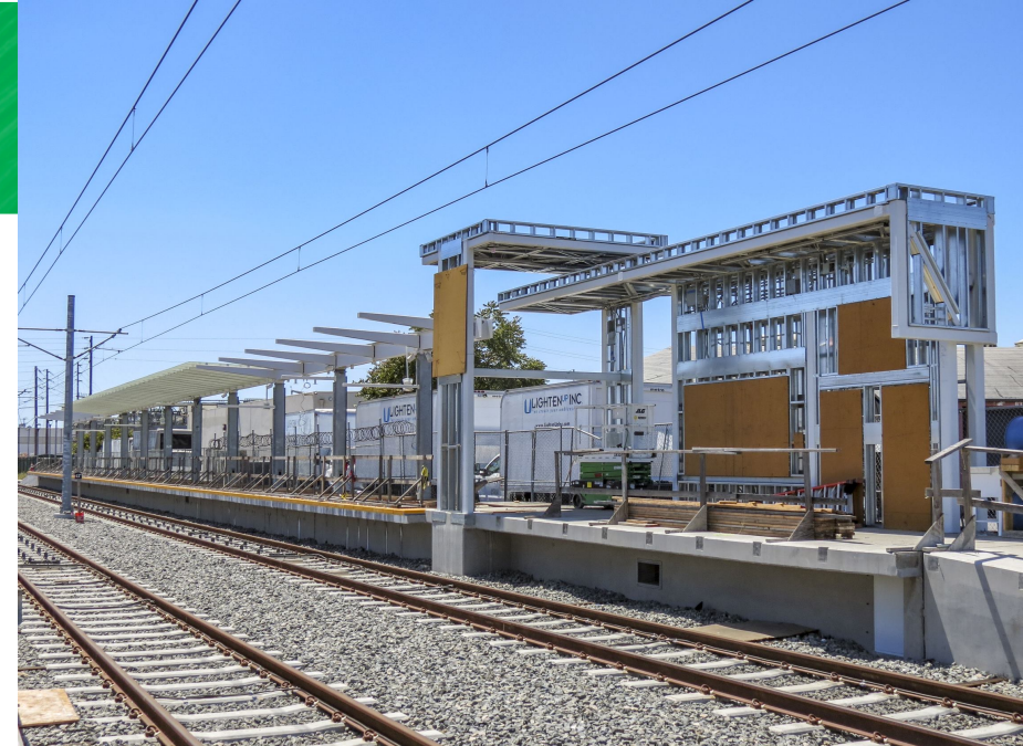
TVM canopy under construction
