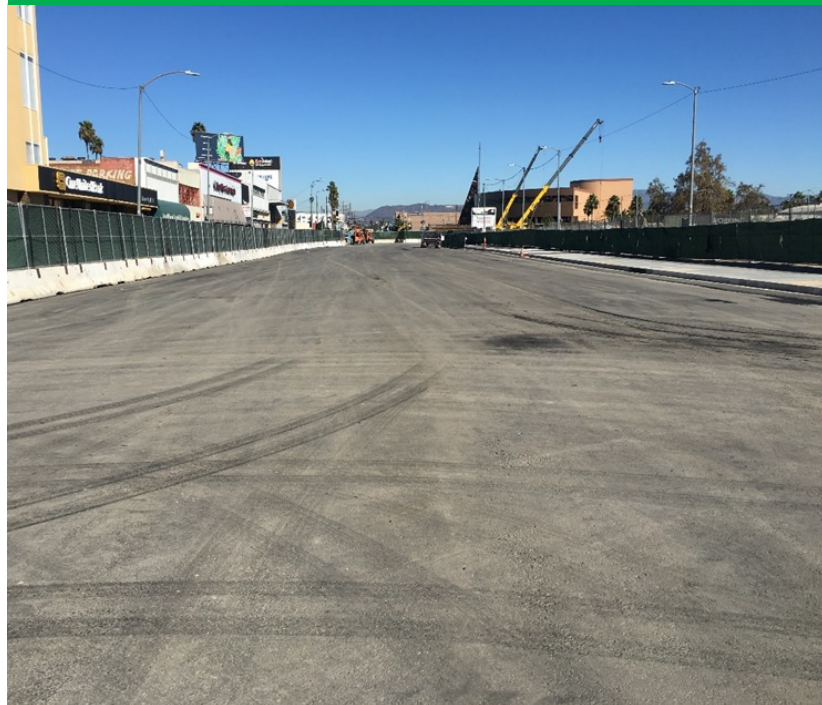
Street restoration of Crenshaw Bl
