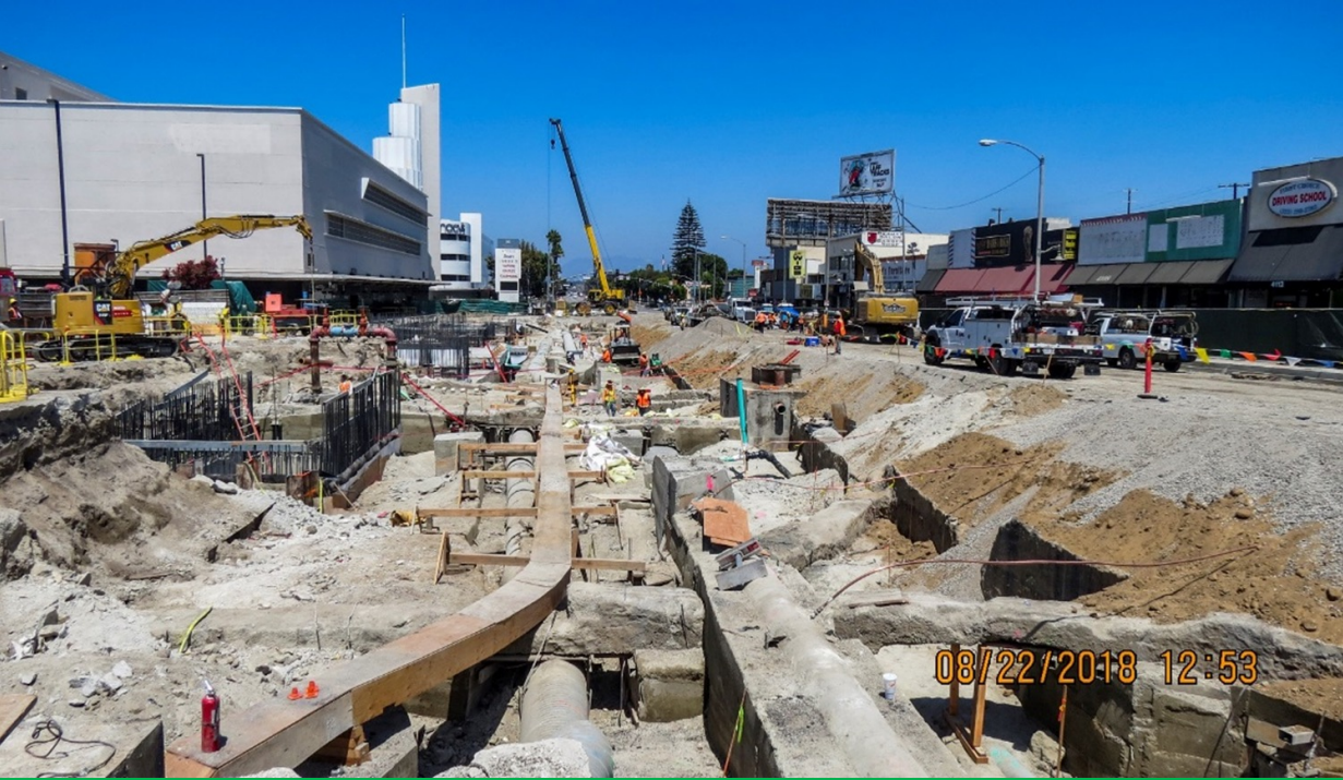
Excavated underground station
