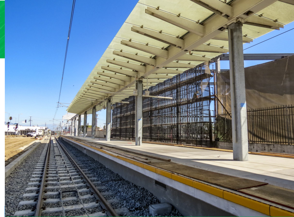
Station platform under construction
