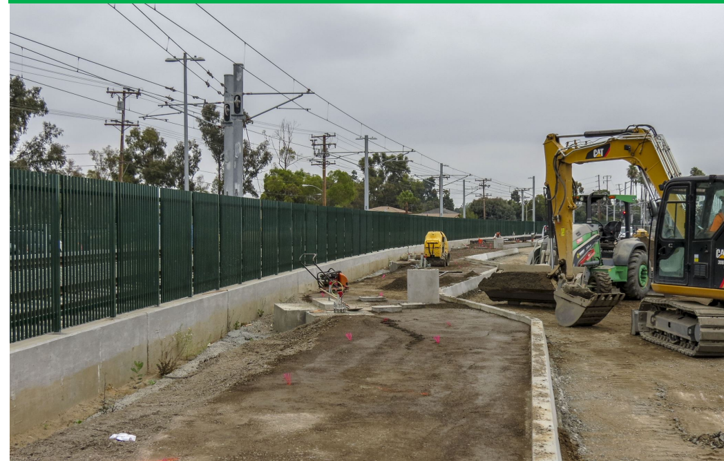
Bus Transfer Facility under construction
