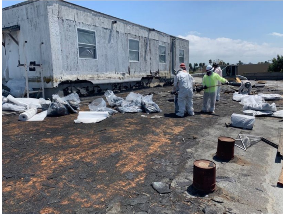
Abatement of roofing material
