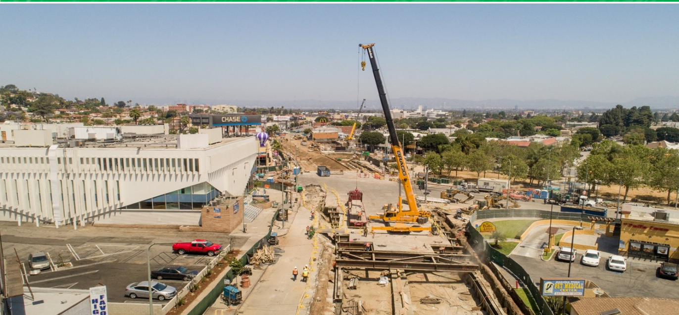
Backfill and decking removal operation at station area
