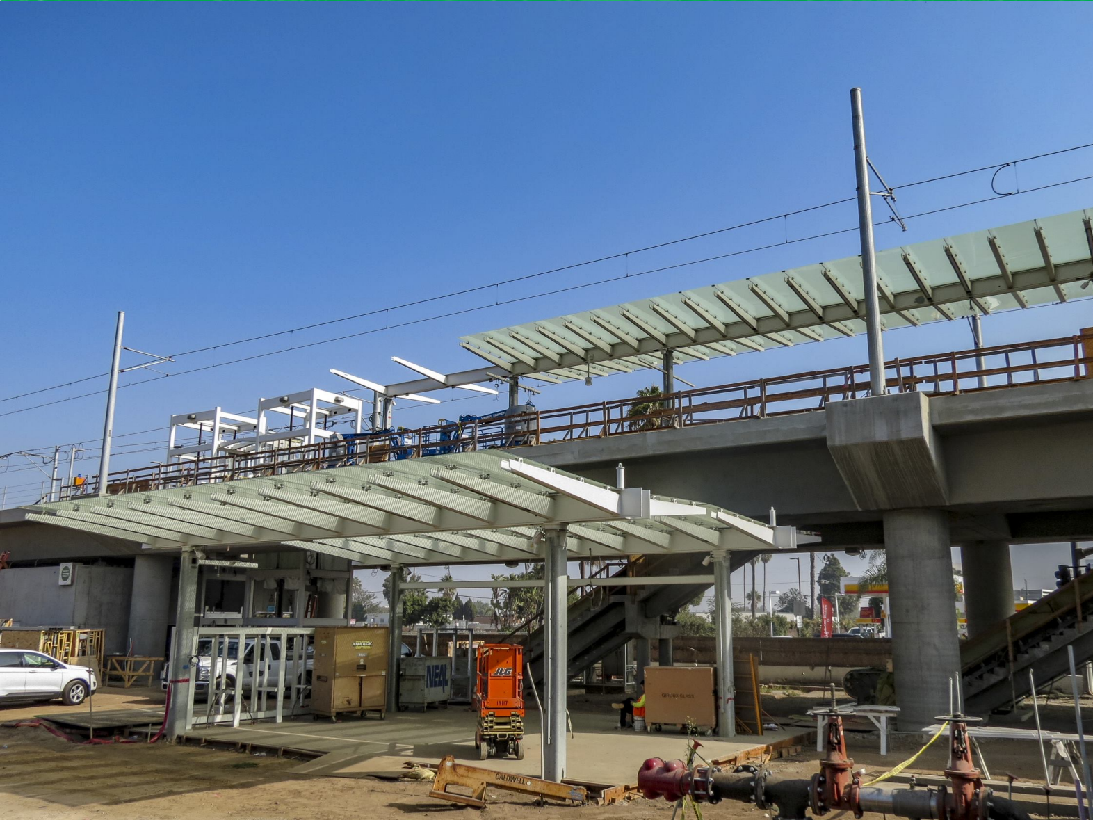
Station canopy and station plaza under construction
