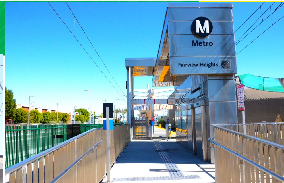
TVM canopy at western end of station
