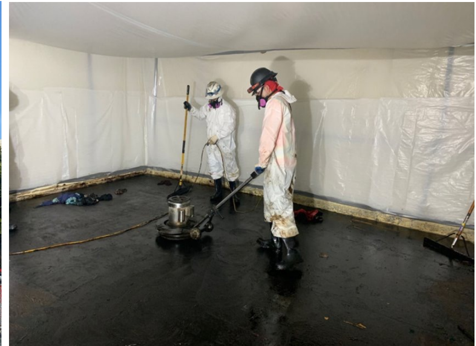
Workers removing glue that held flooring
