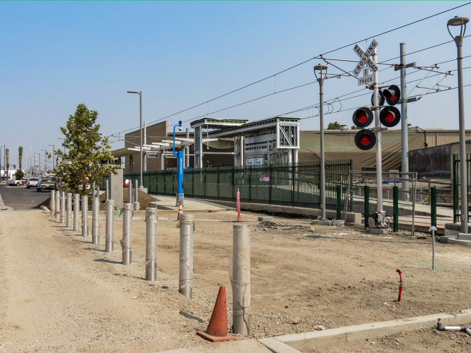
Station parking lot and TVM canopy under construction
