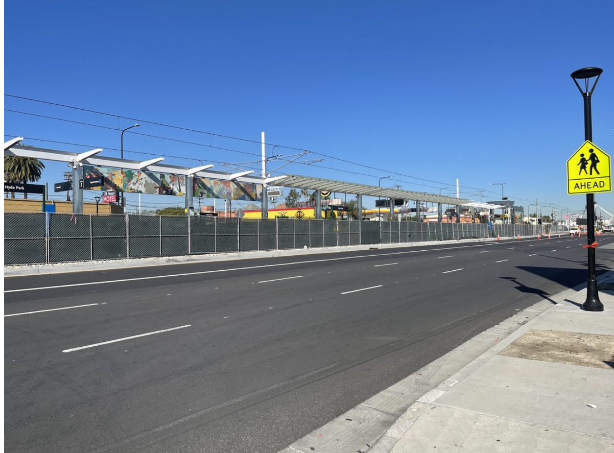
Restored and paved street of Crenshaw Bl near station
