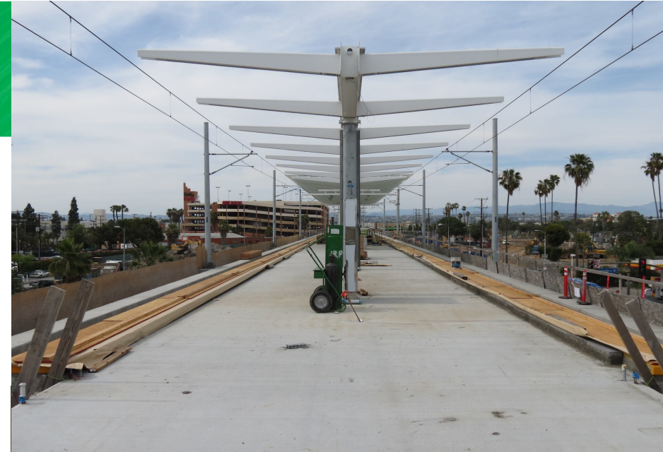
Station platform under construction
