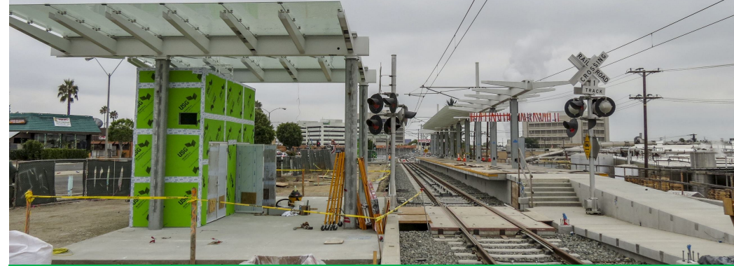
TVM canopy under construction
