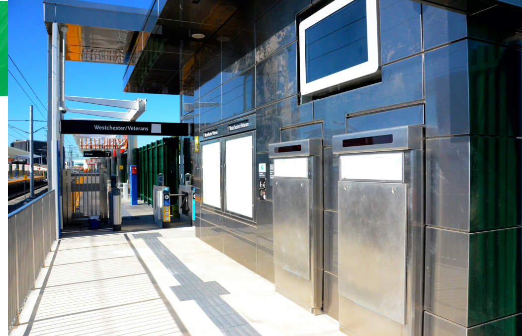
Platform entrance and Ticket Vending Machine
