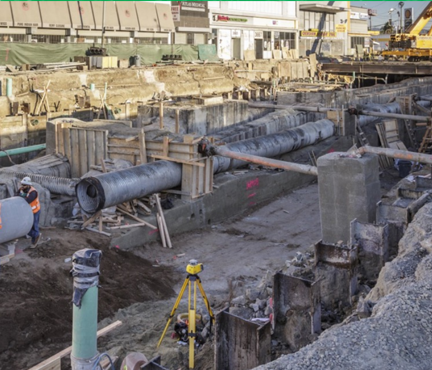
Station backfill and decking removal operation
