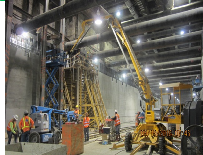
East wall construction
