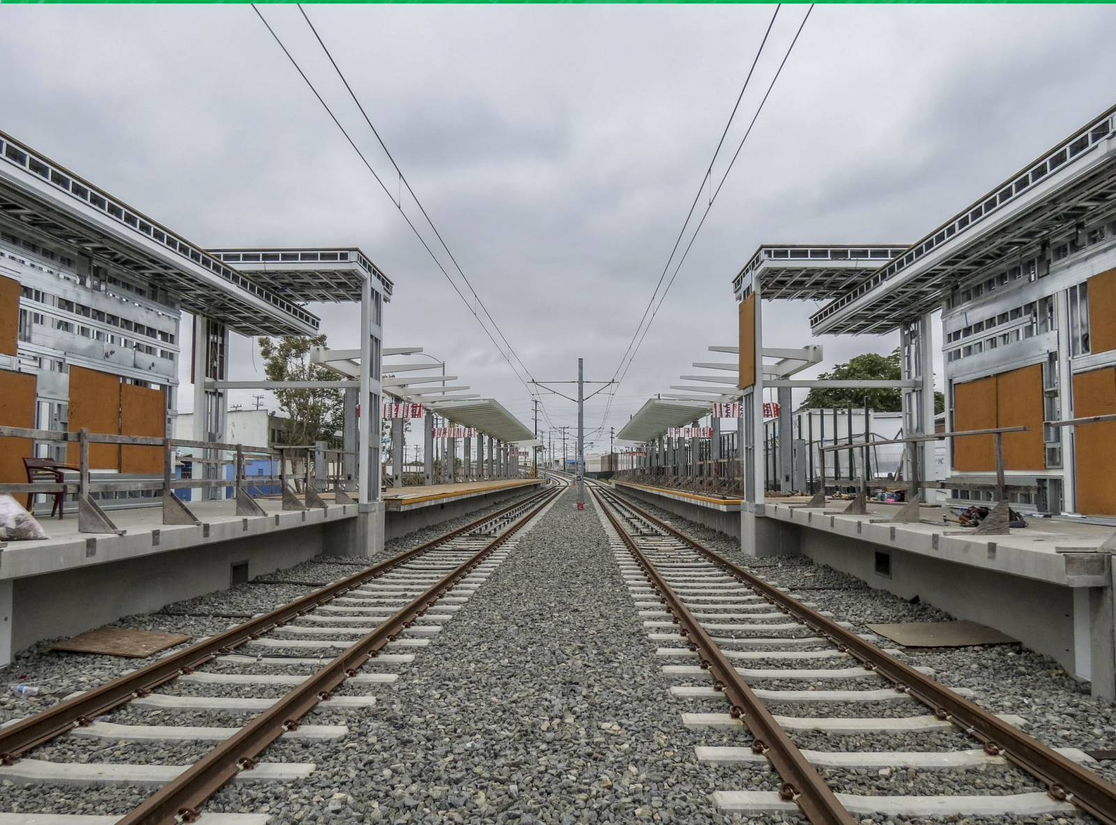
Split-platform station under construction
