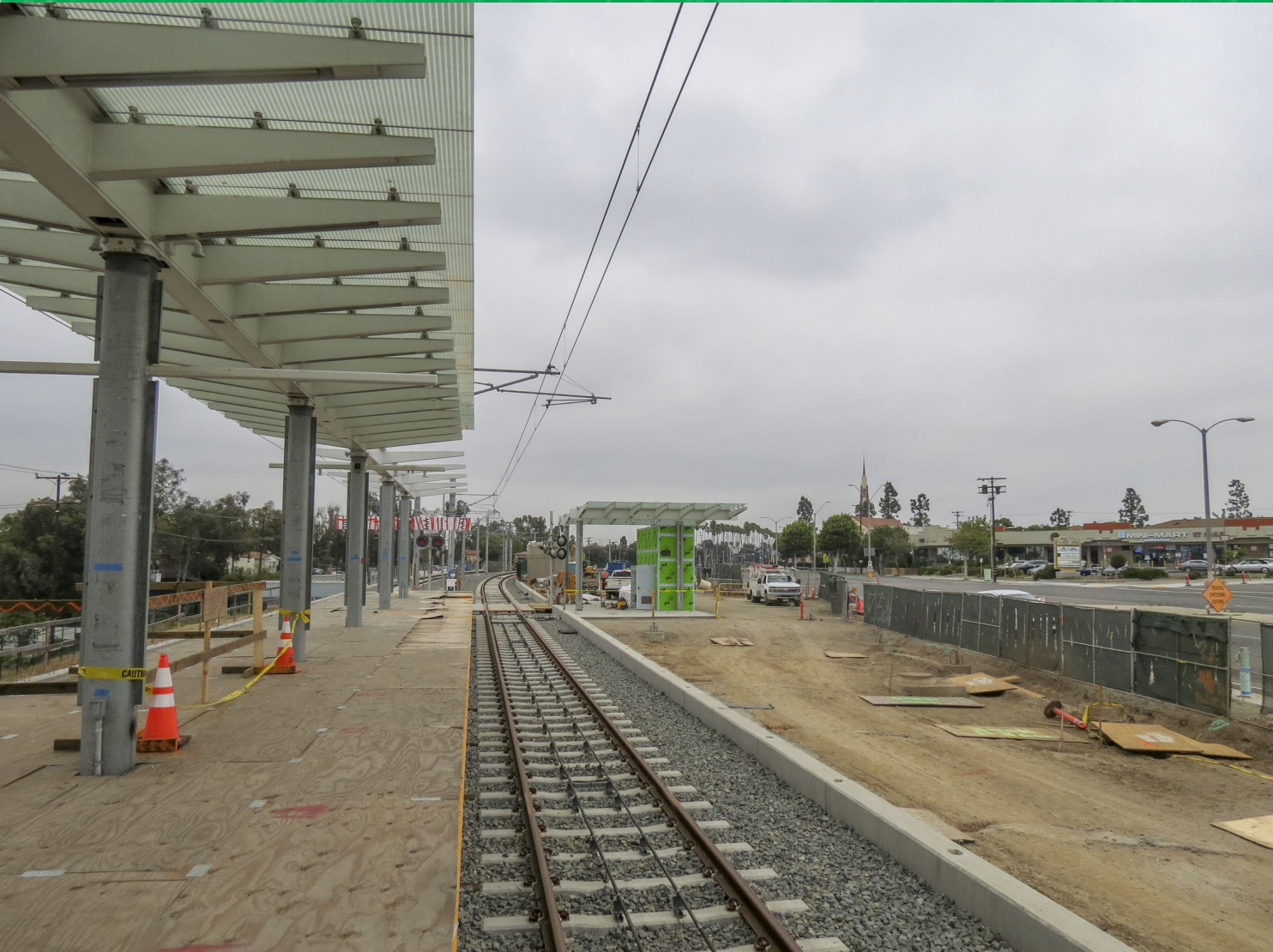
Station platform and plaza under construction
