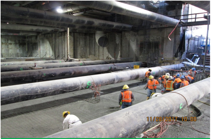
Concrete placement for concourse deck
