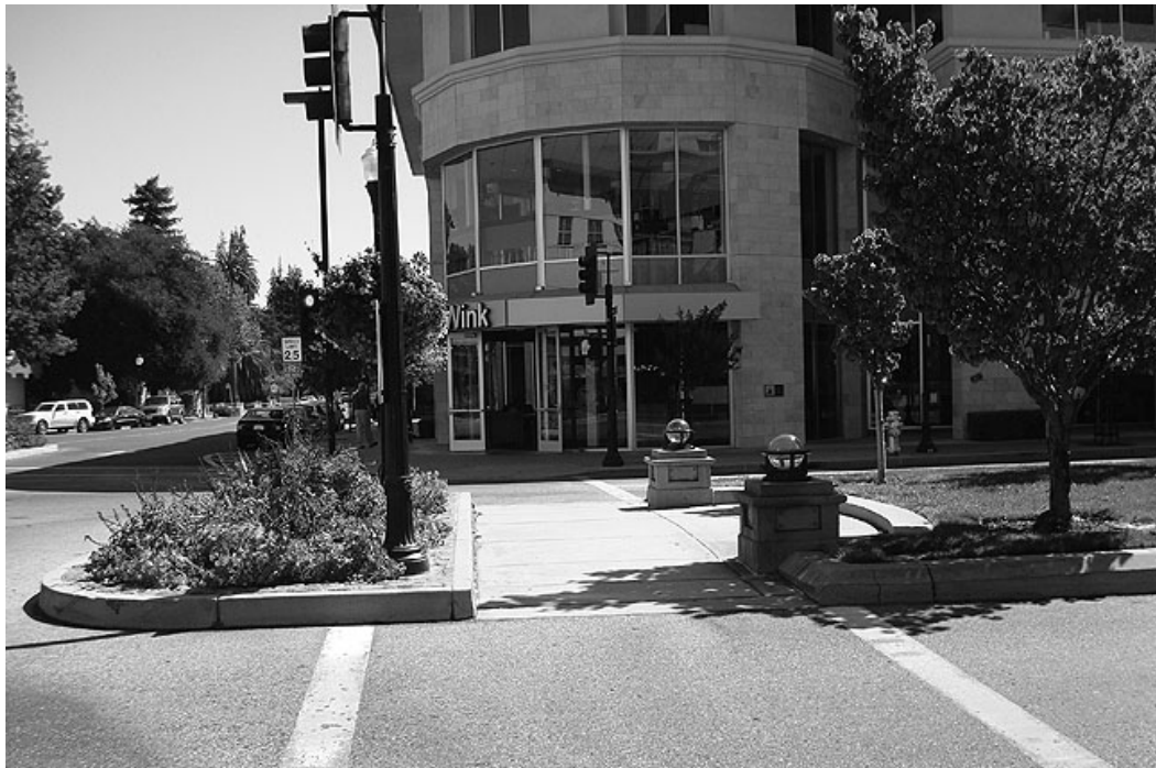
Figure 2-6: Pedestrian Refuge Median
