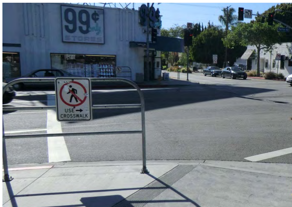
Figure 3-3: Pedestrian No Crossing Barrier
