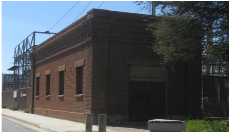
Figure 4-52. Edison Substation – Florence and Fir Avenues
