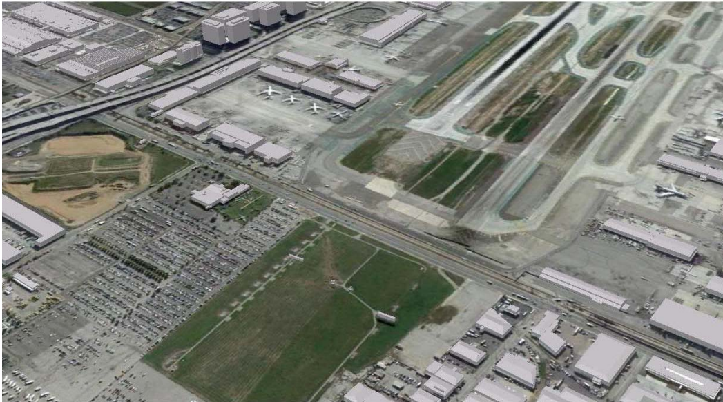
Existing view of Aviation Boulevard in front of the LAX south runways.
