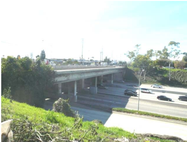
Florence Avenue bridge over I-405 looking northeast.
