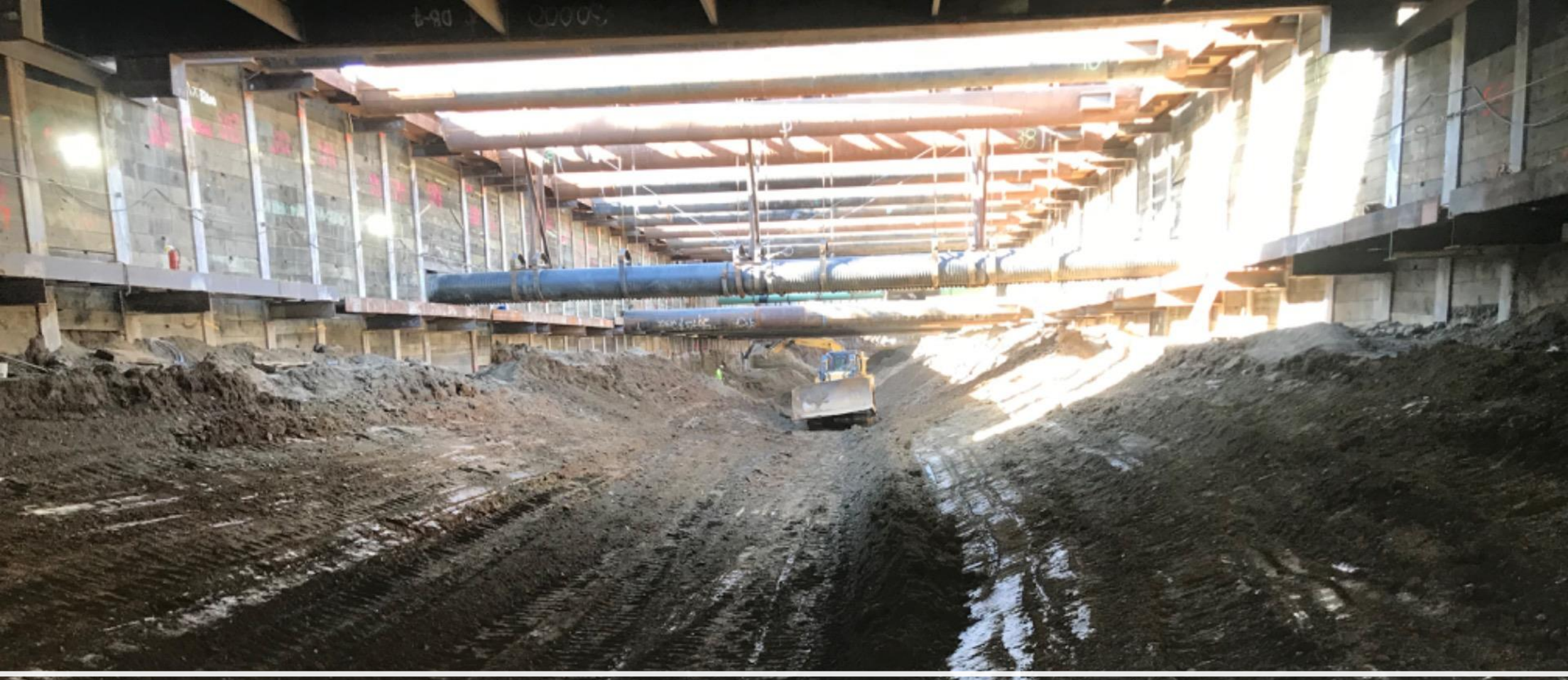
Station Excavation in Progress
