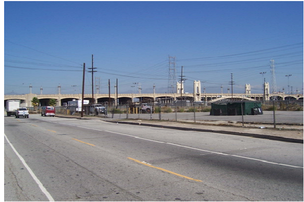
Figure 4-37. View looking north toward the Fourth Street Bridge from Santa Fe Avenue
