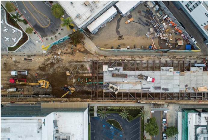
Metro D Line tunneling at the future Wilshire/Rodeo Station
