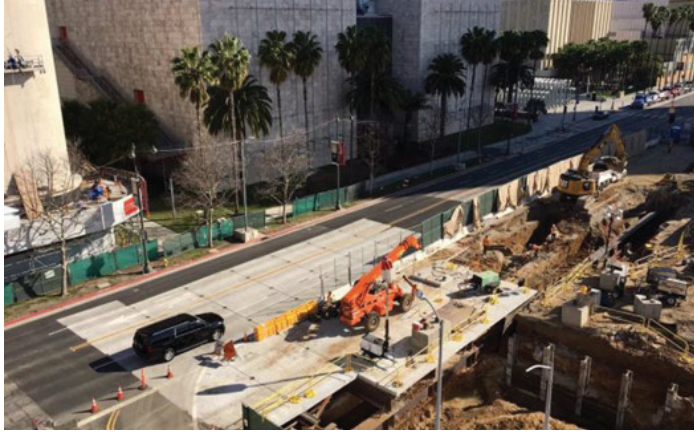
Future Metro D Line tunneling
