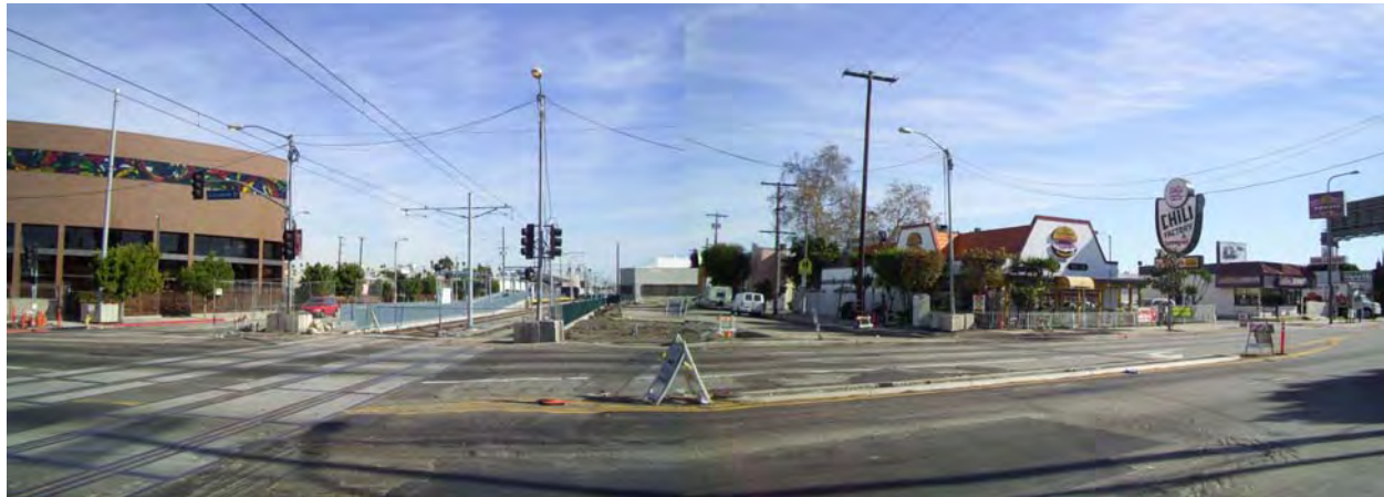
Existing Crenshaw Boulevard and Metro Exposition Line (Under Construction)
