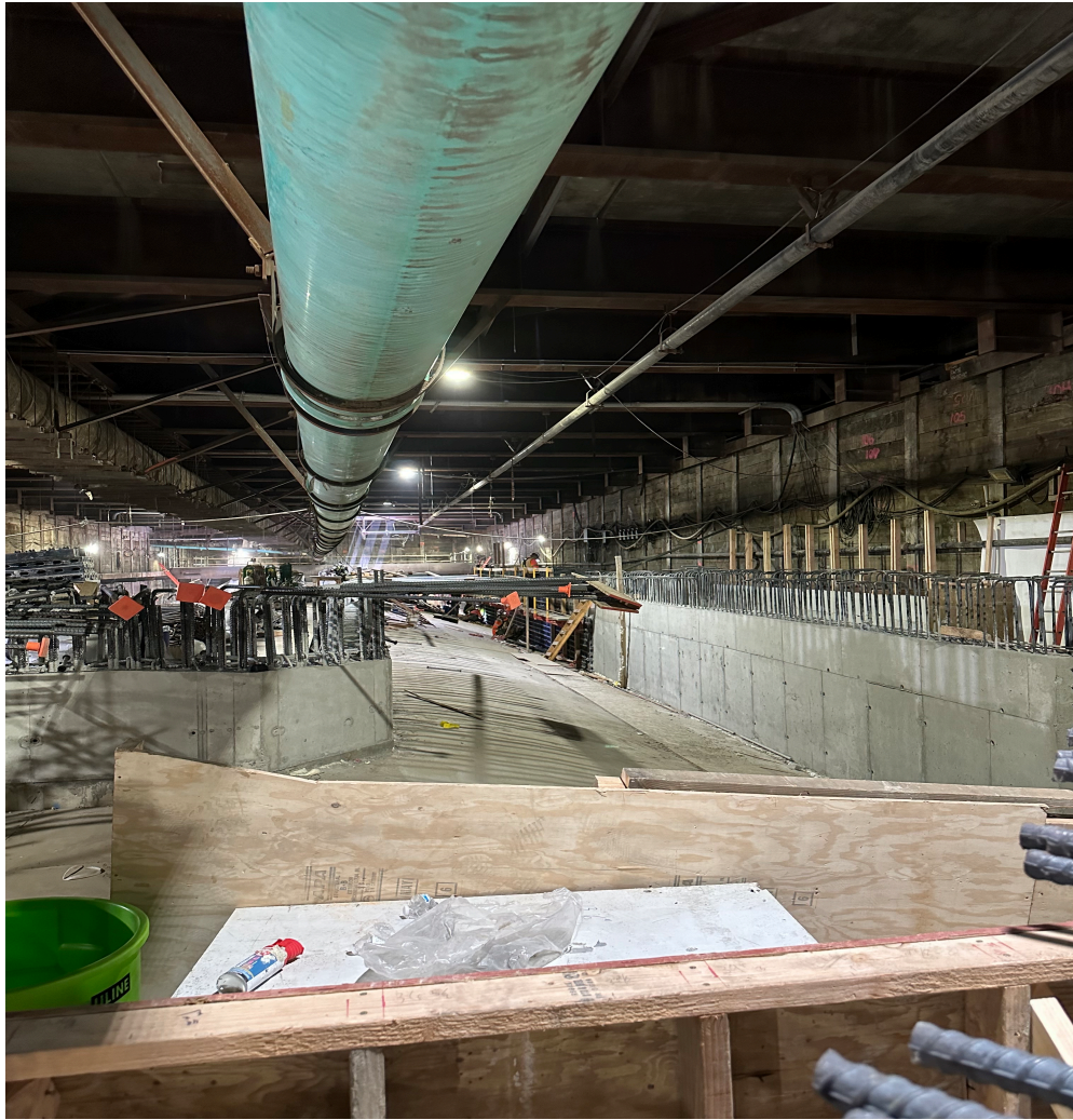
East High Bay Station Roof Progress July/August 2024
