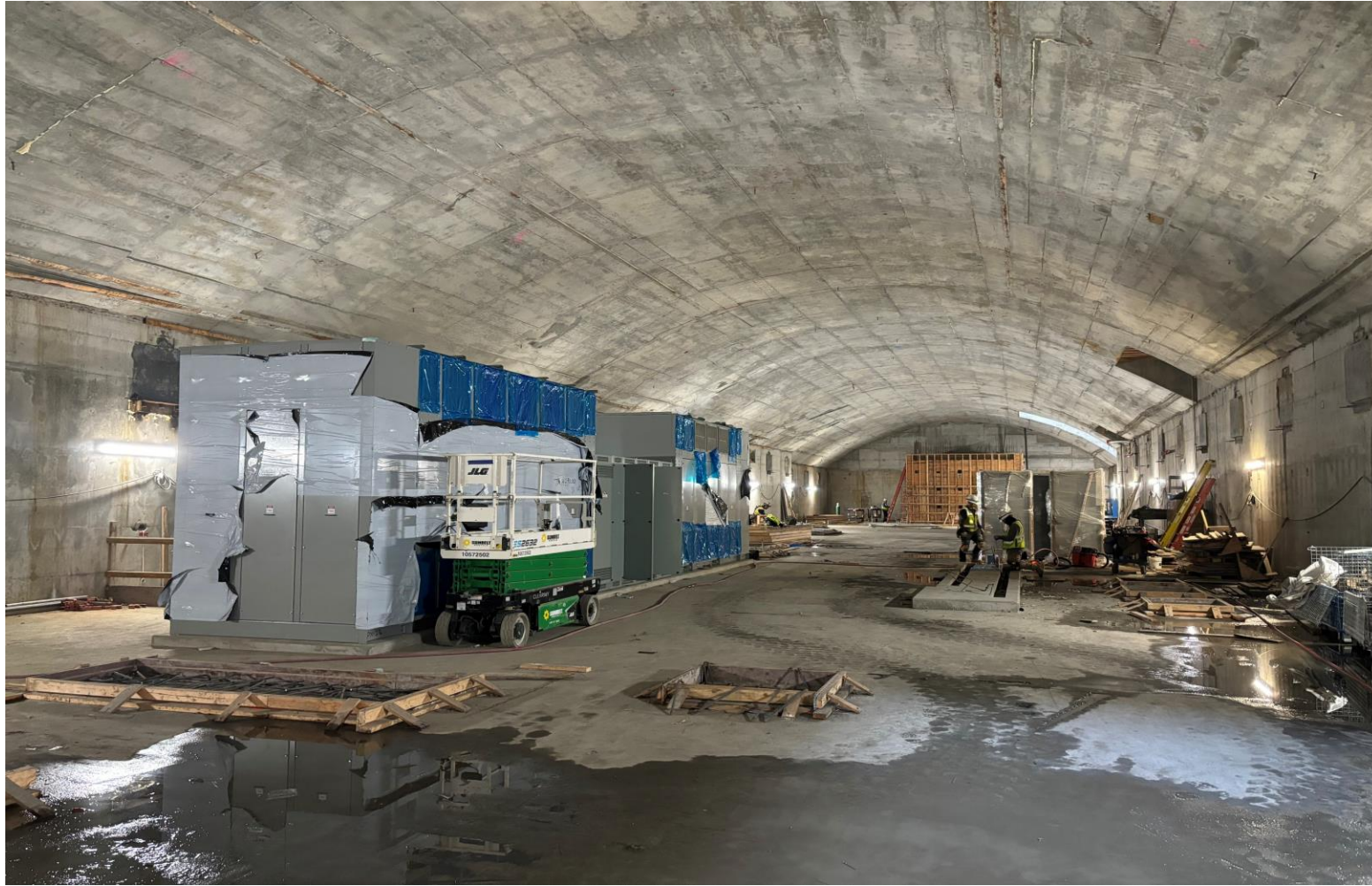
East End of Station Concourse
