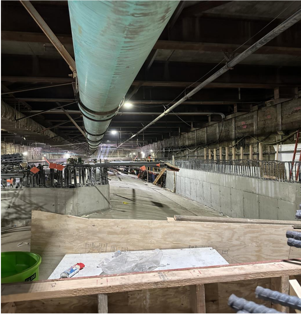
East High Bay Station Roof Progress July/August 2024
