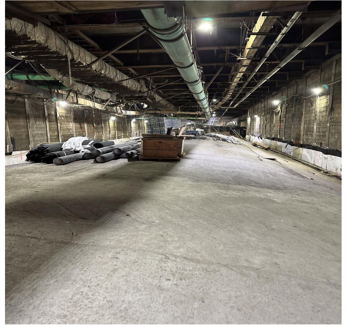
West High Bay Station Roof Progress July/August 2024
