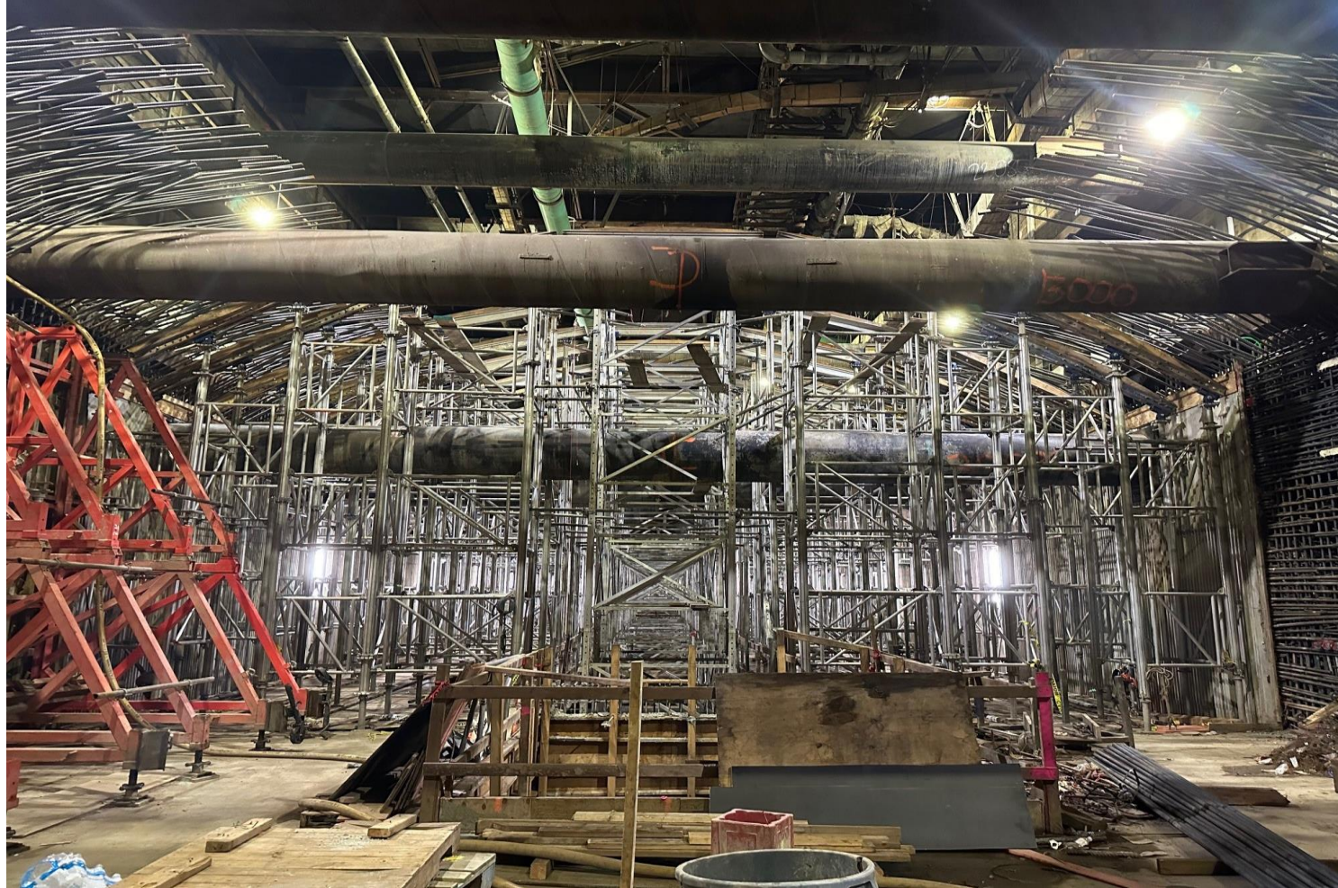
Station Roof Falsework Towers May 2024
