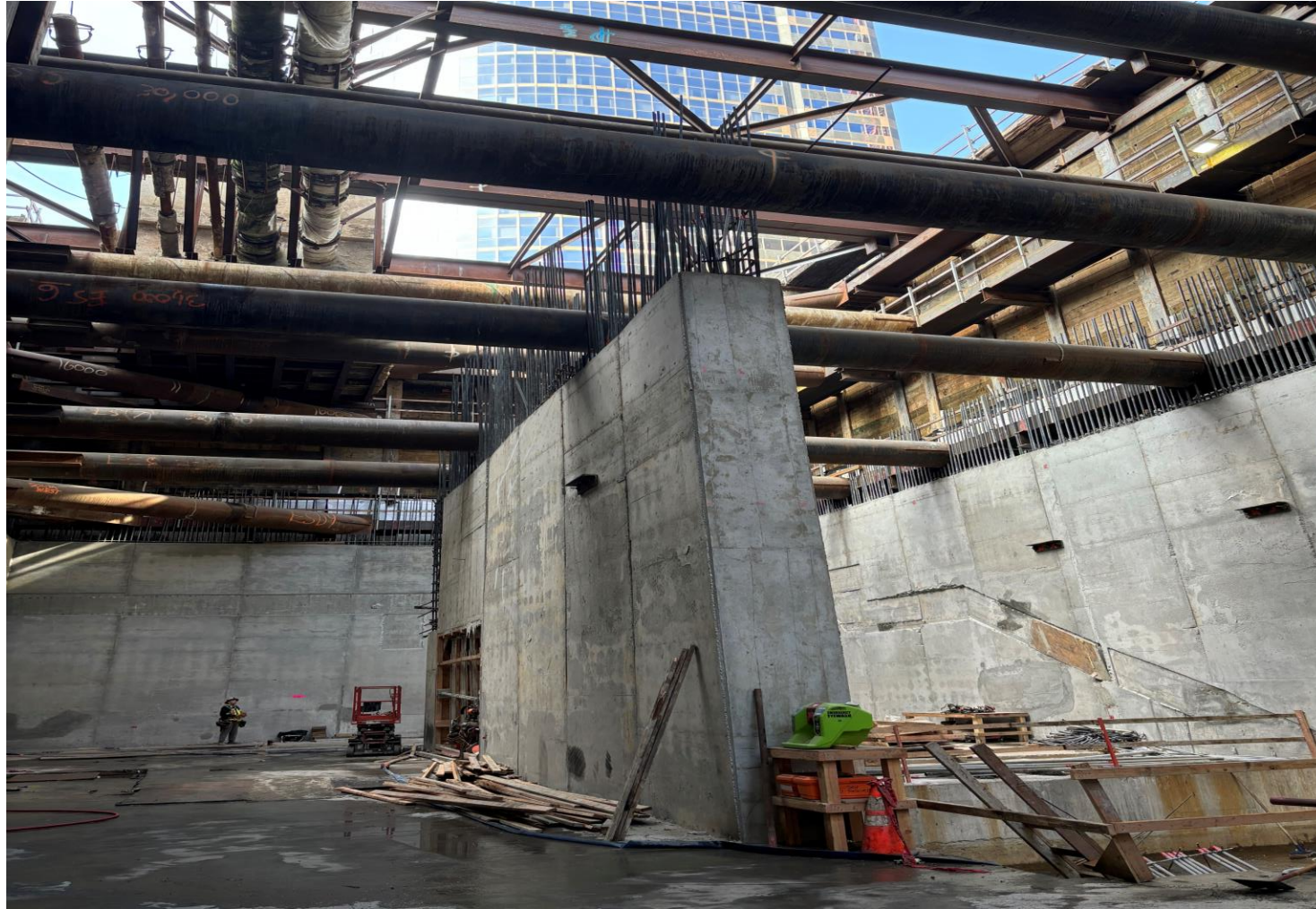
Concourse Entrance Interior Walls at Future Escalators
