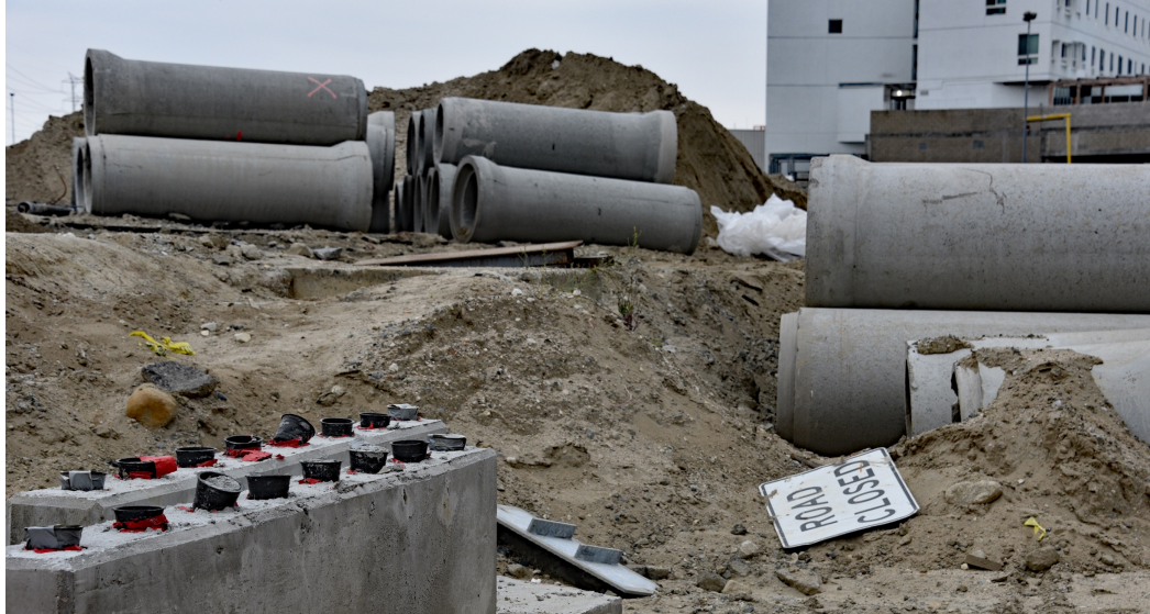
Storm drain segments buried in the south yard.
