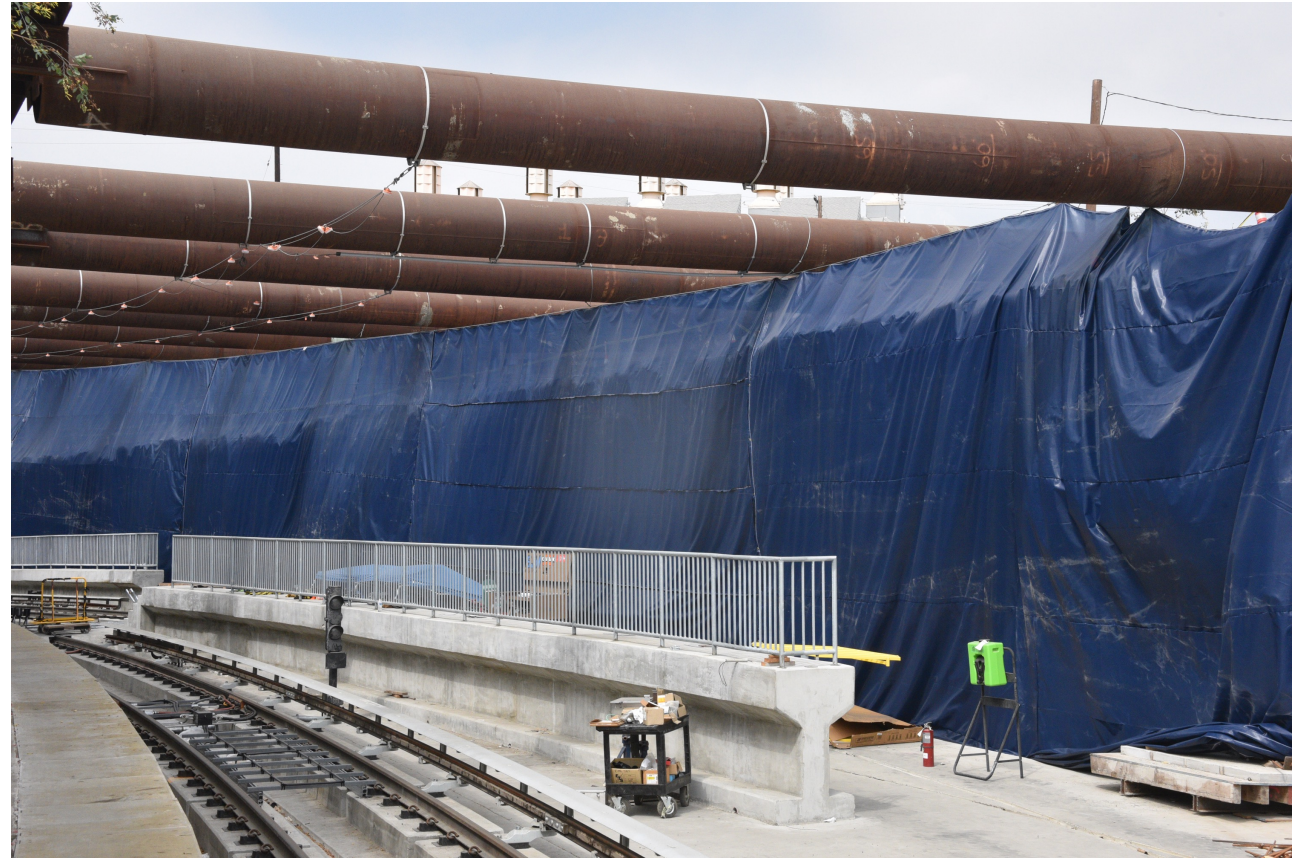
West portal. Blanket protects from flying objects during demolition
