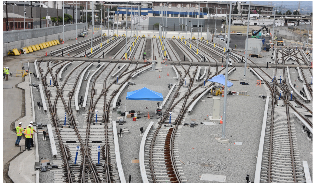
North Yard looking north
