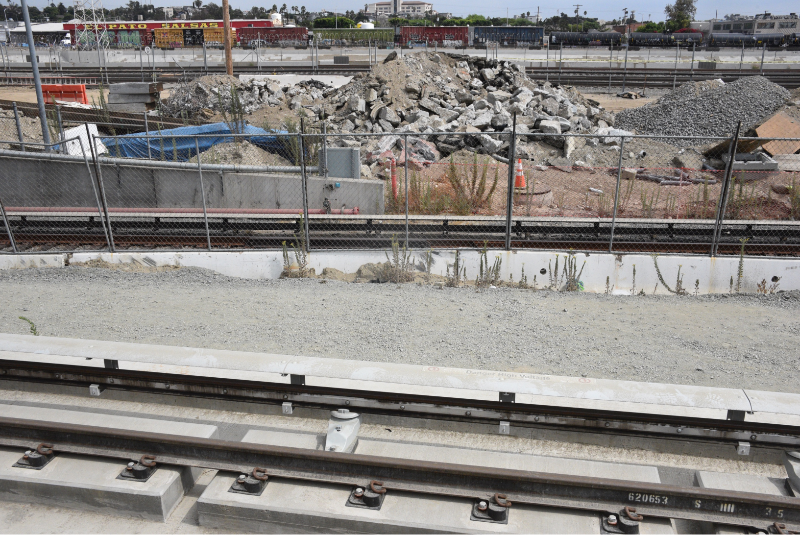
Demolition continues near east portal site.
