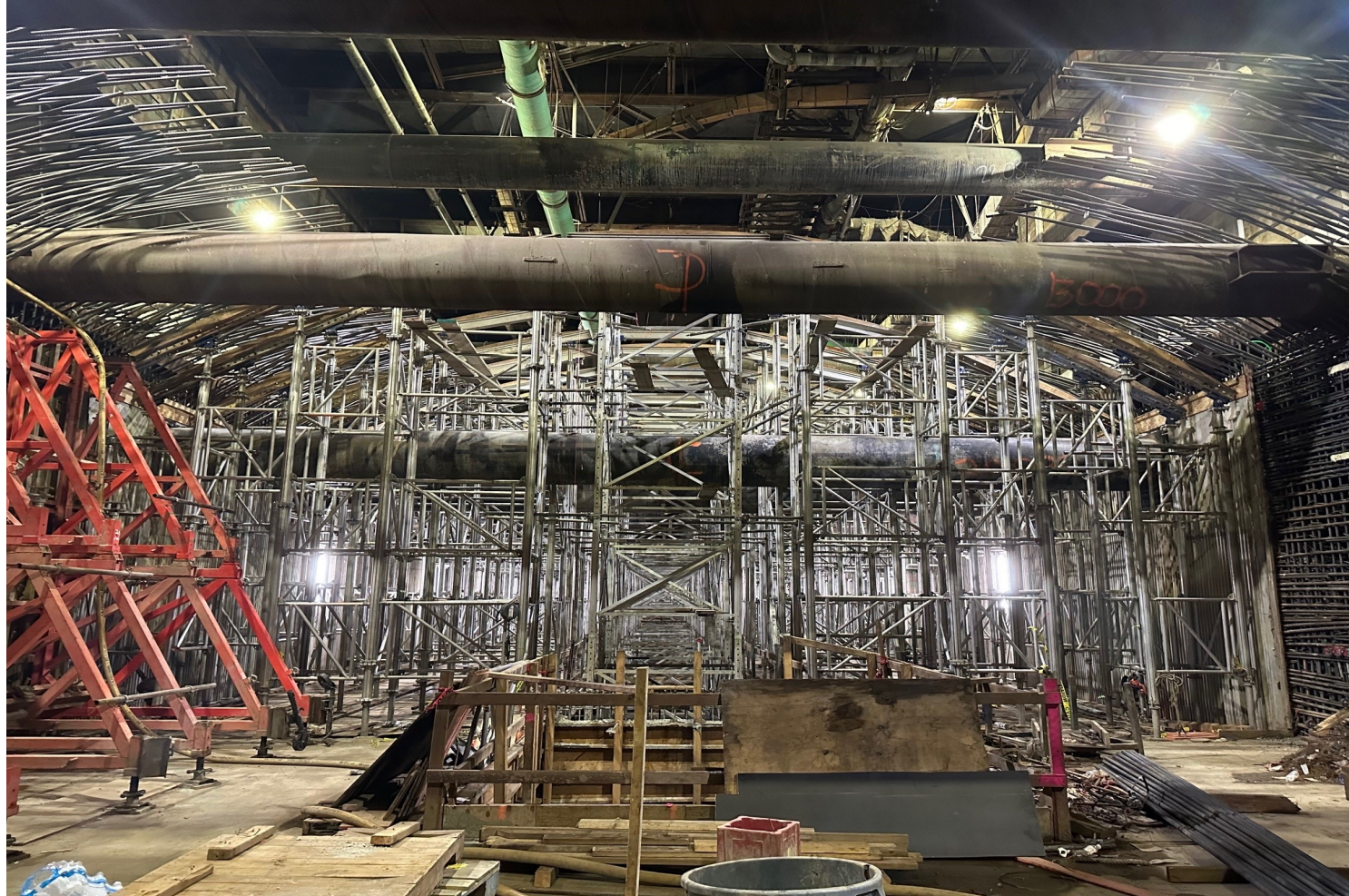
Station Roof Falsework Towers May 2024
