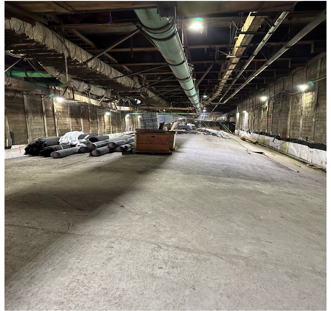
West High Bay Station Roof Progress July/August 2024
