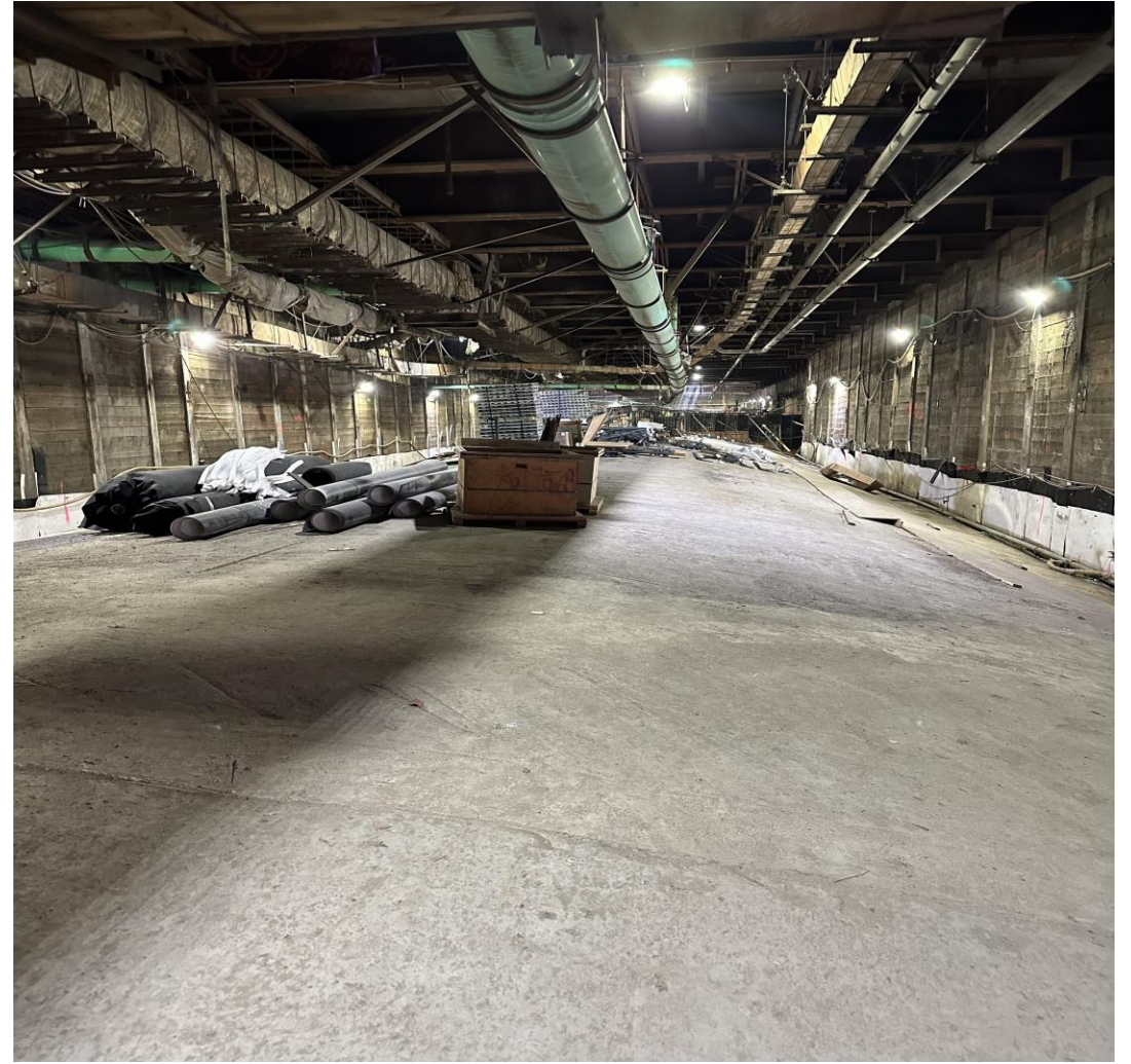
West High Bay Station Roof Progress
