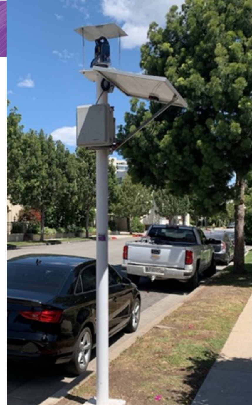
Example of 10-foot geotechnical instrumentation pole.
