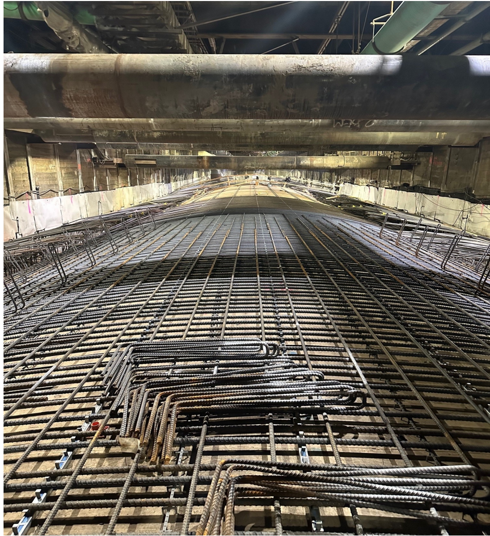
East High Bay Station Roof Progress
