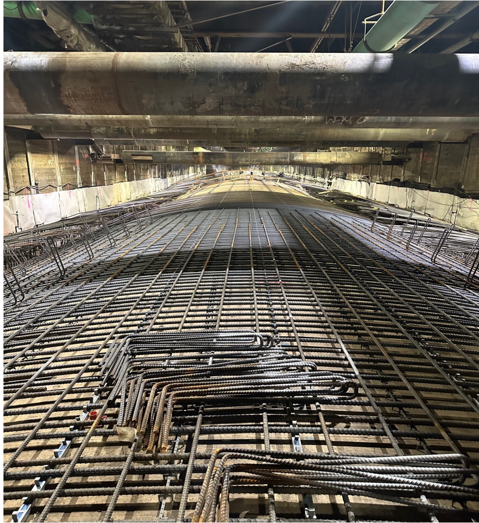
East High Bay Station Roof Progress
