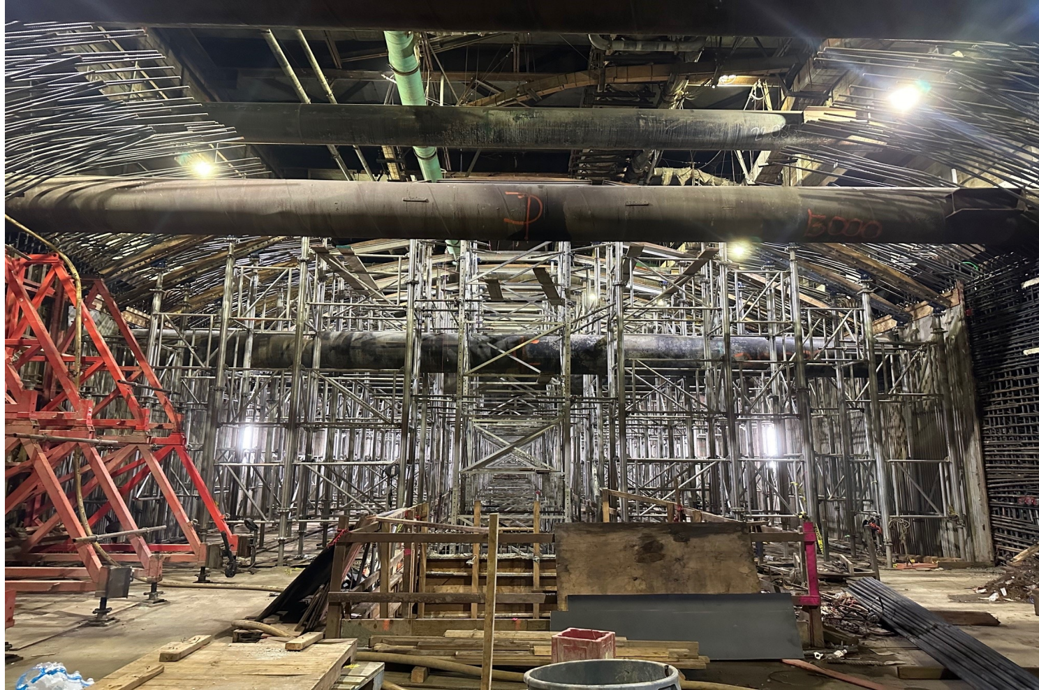
Station Roof Falsework Towers
