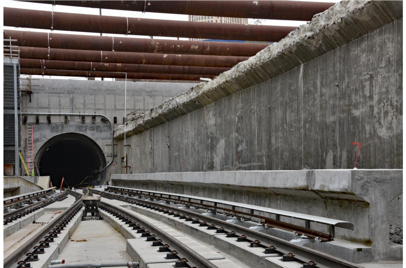
West portal nearing completion. Notice the contact rail cover.
