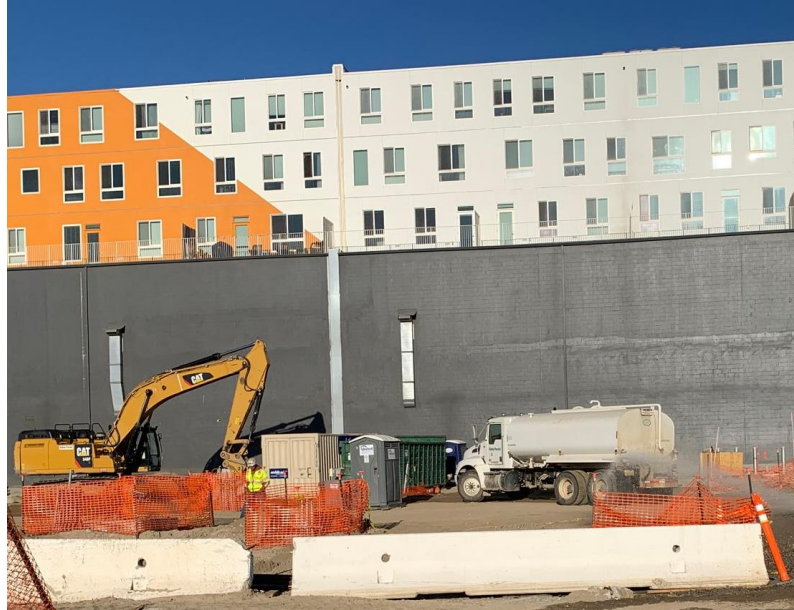
Watering truck east of One Santa Fe reduces dust.
