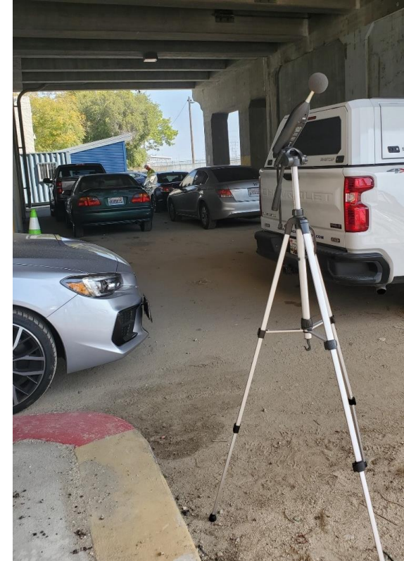
Workers monitor noise as excavation in the south yard continues.
