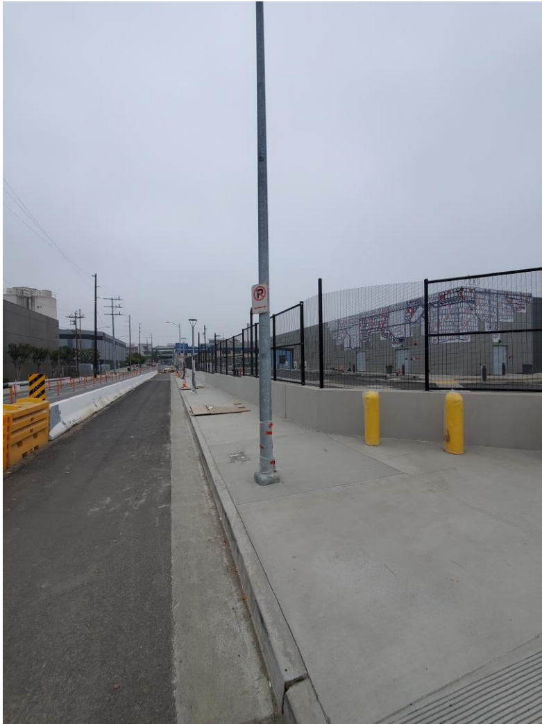
Center St: Civil improvements nearing completion
