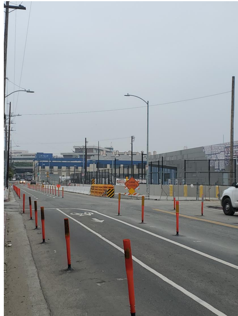
Center St: Temporary traffic lane reconfiguration to be removed June 3rd
