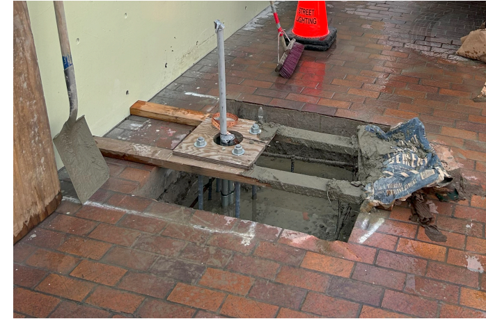
Building the foundation of one of the two new streetlights on Azusa St
