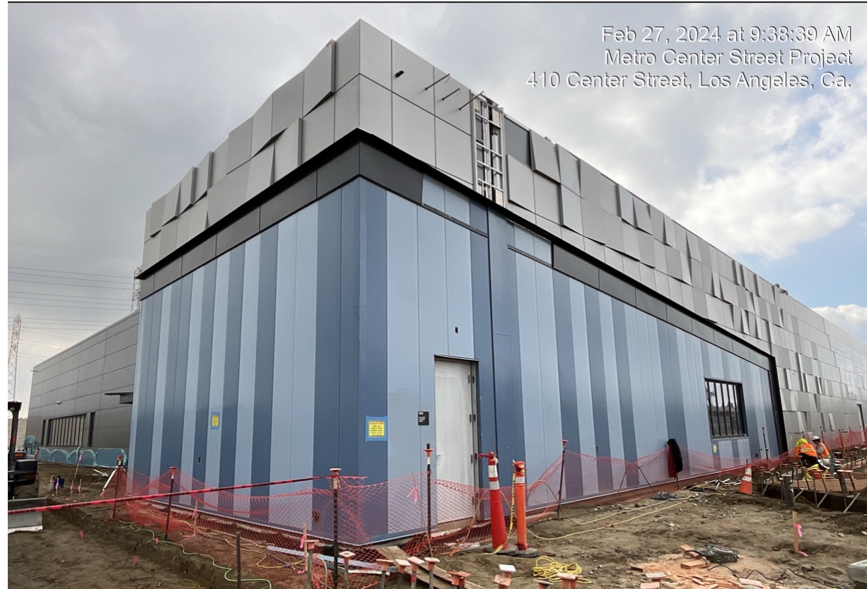
Northwest corner of building (view looking southeast)
