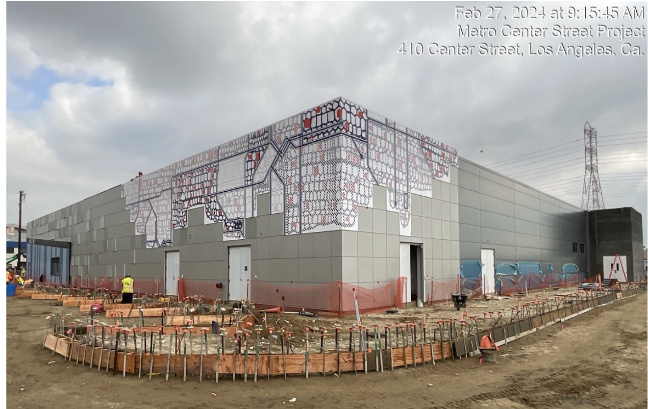
Southwest elevation of building (view looking northeast)
