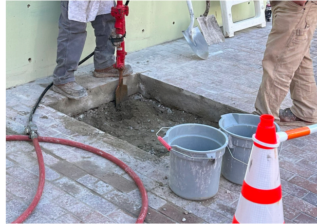
Building the foundation of one of the two new streetlights on Azusa St
