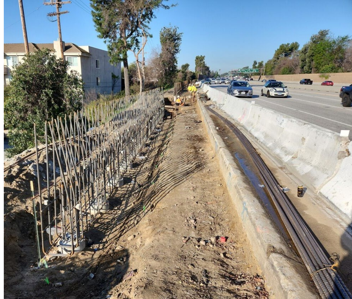
SR-134 west view of rebar iron work.
