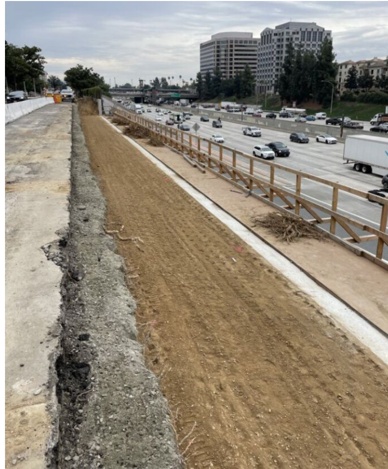
Demo, grading, and form work.
