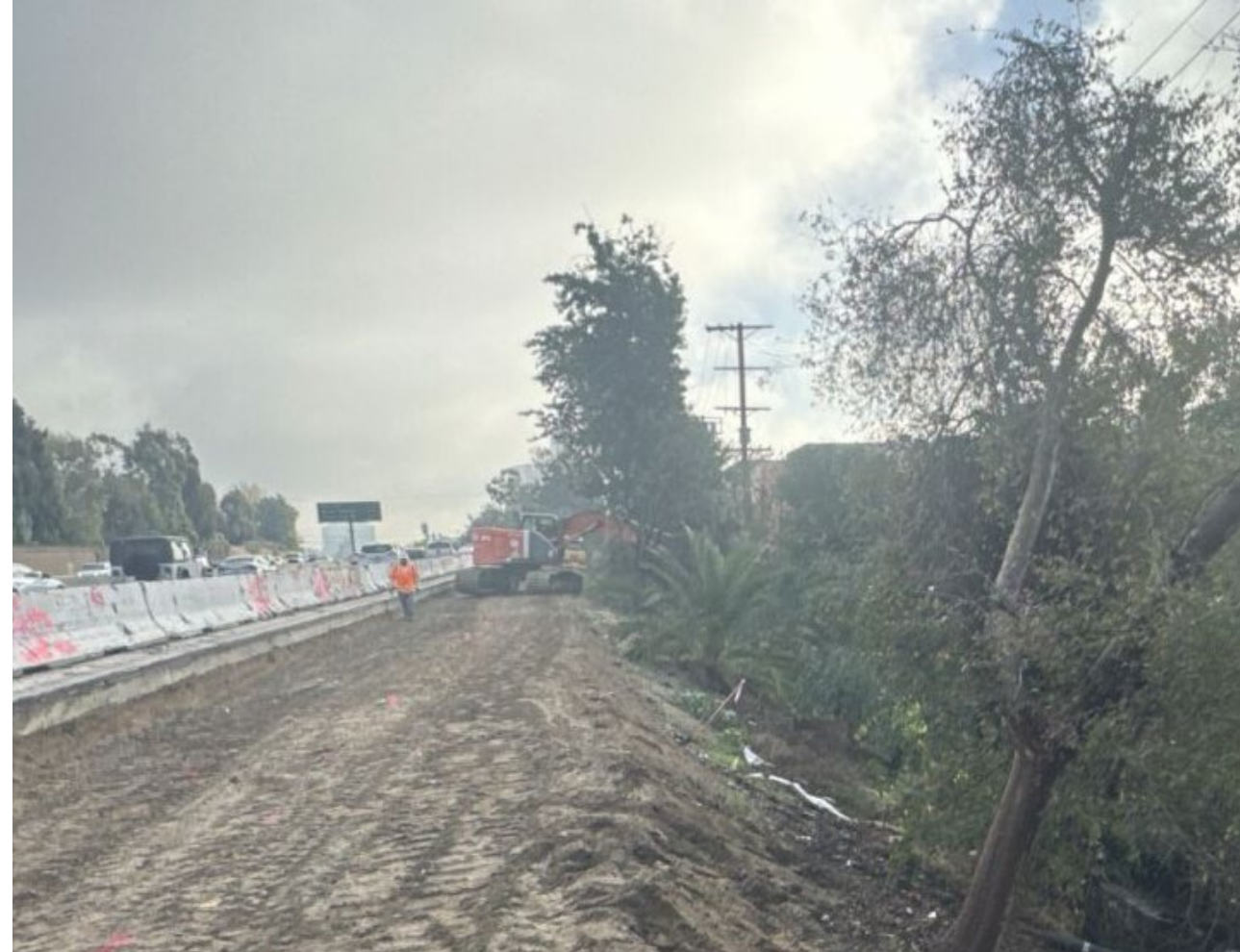
East view after clear, grub, demo operations.
