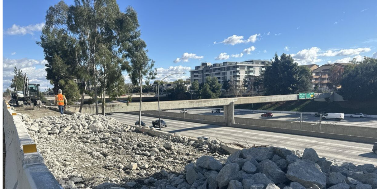
East view of I-210 clearing and demo operations
