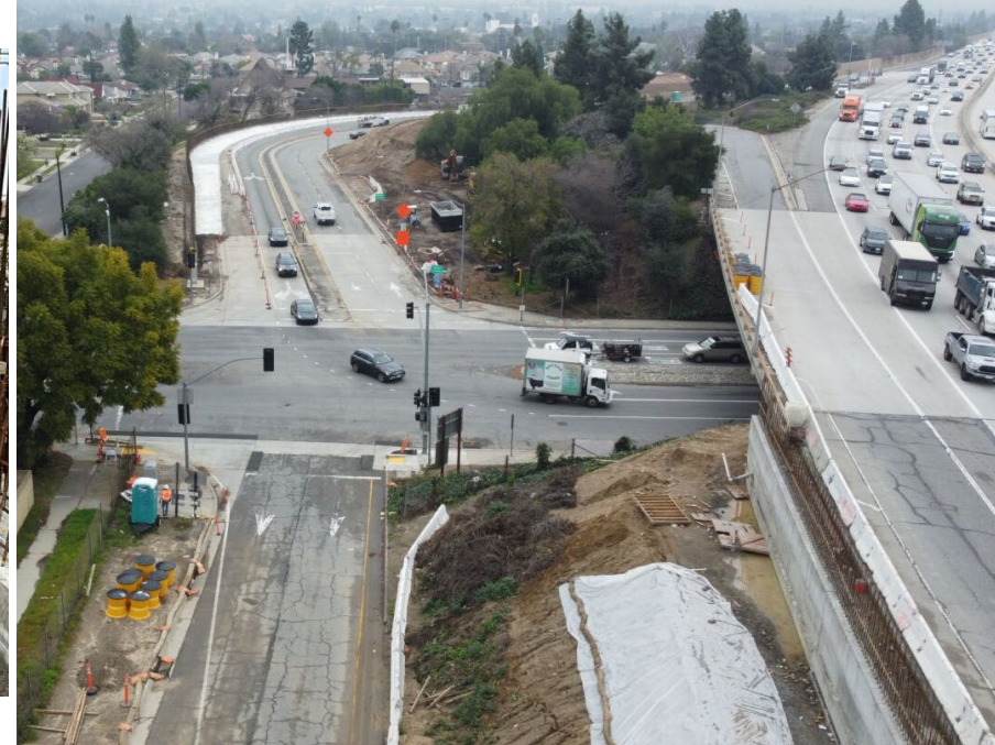
Concrete and rebar for concrete barrier.
