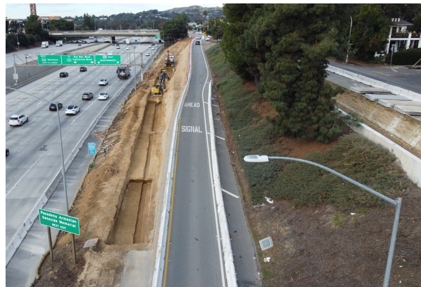
West view of I-210 Marengo Av off-ramp retaining wall excavation.
