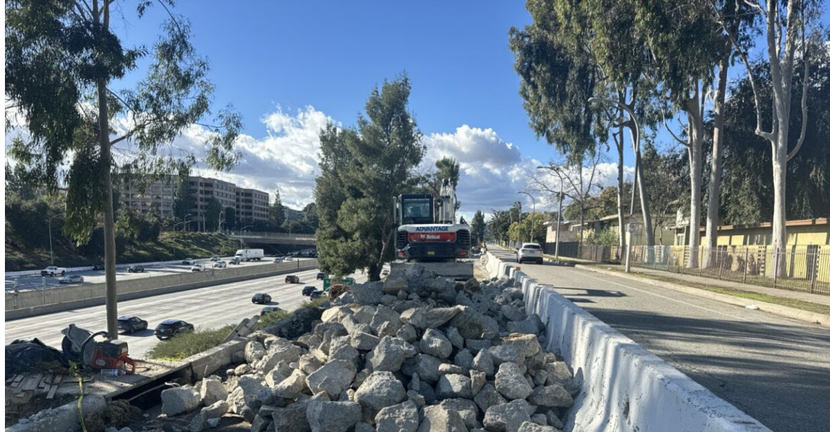
West view of I-210 demo operations along Maple St
