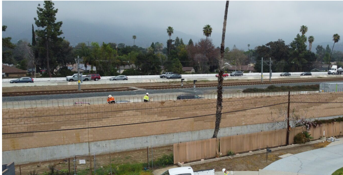
Soundwall lower barrier complete masonry work advancing.
