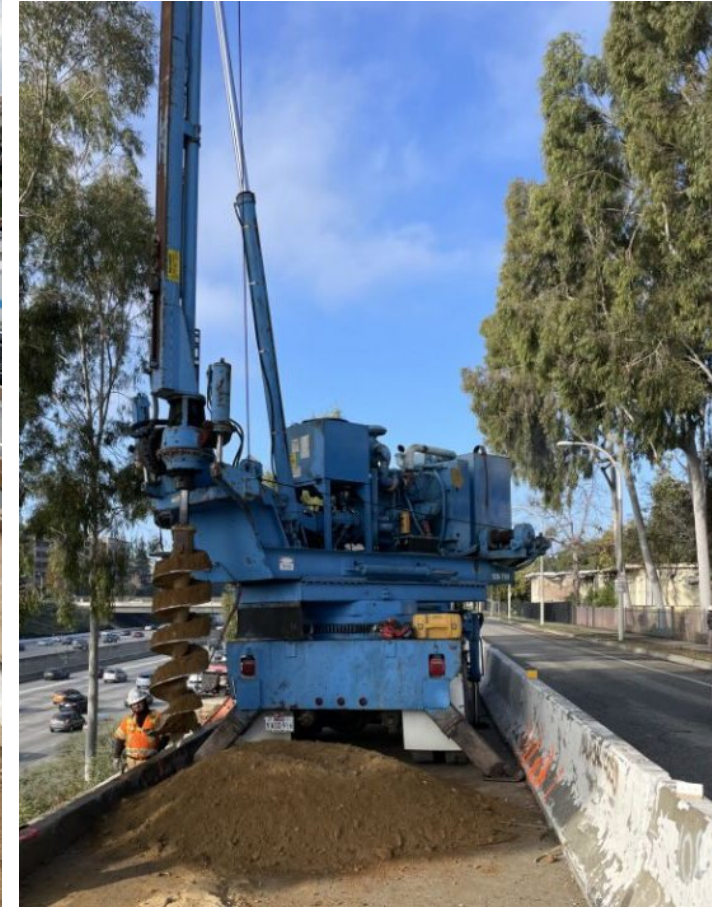
Pile drill and placement along Maple St.
