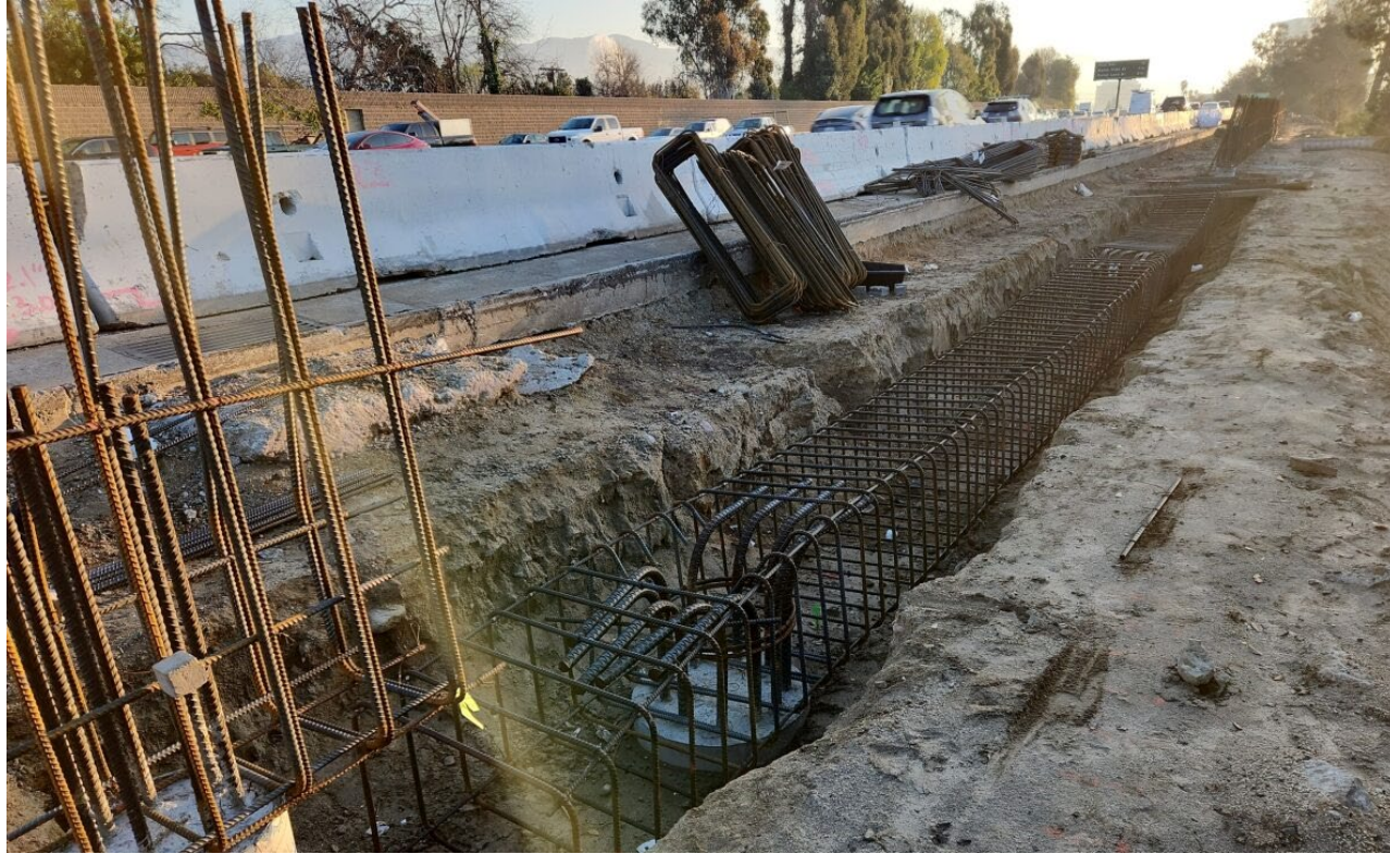
Rebar placement in preparation of pile cap concrete placement.
