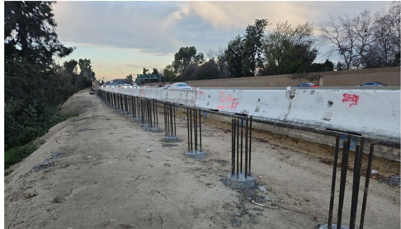
Pile installation completed with rebar/concrete ready for pile cap.
