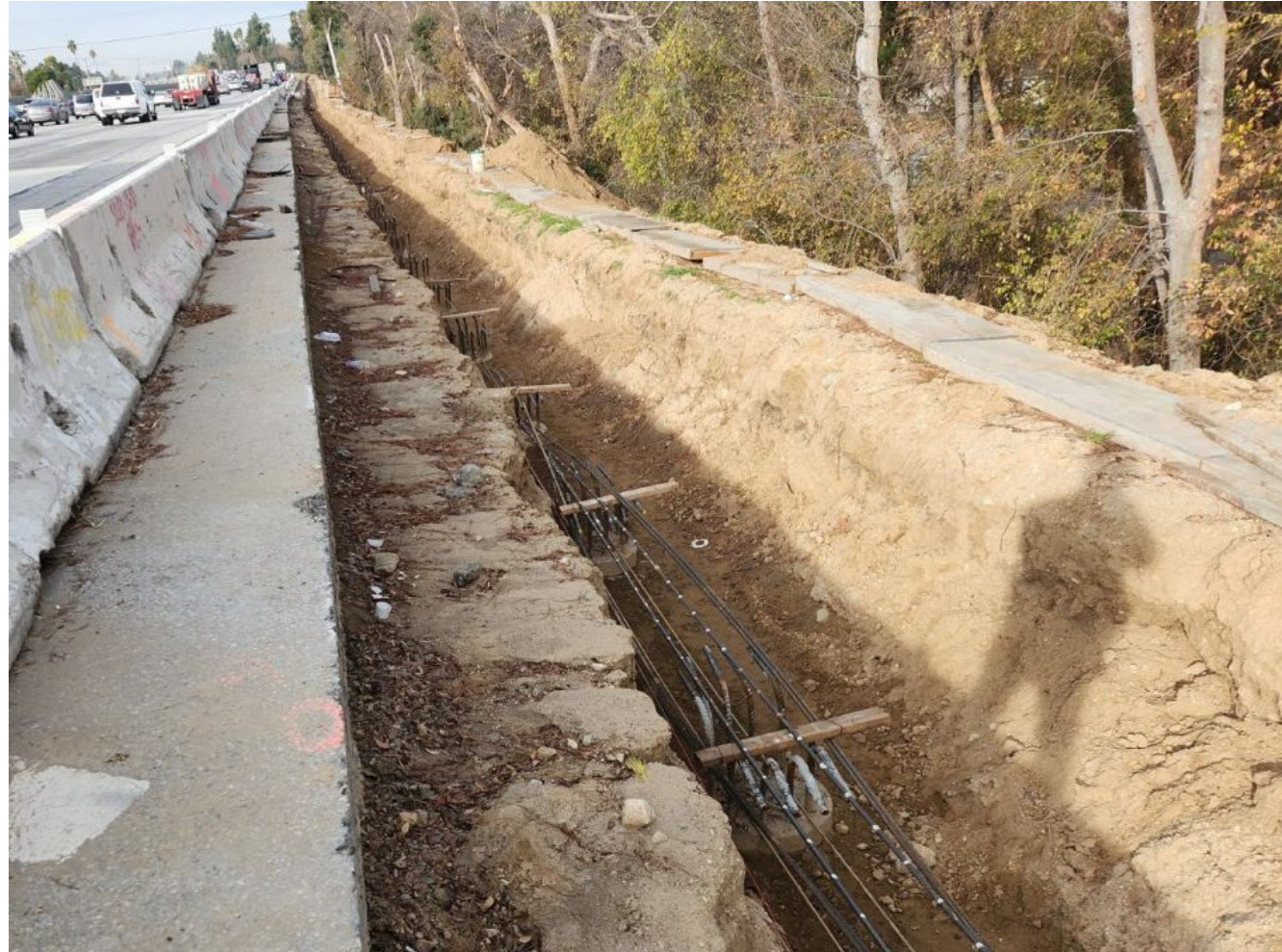
Completed piles, grading, and preparation for pile cap/rebar.
