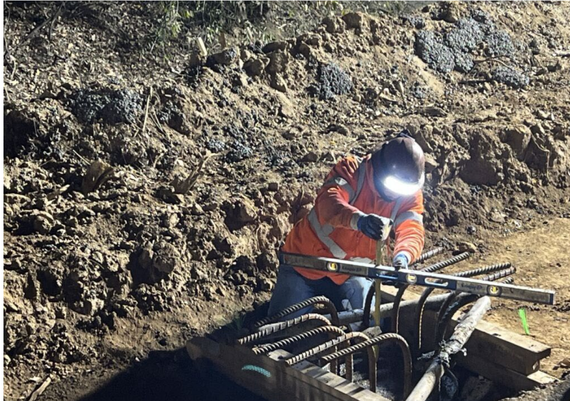
Iron worker adjusting rebar.
