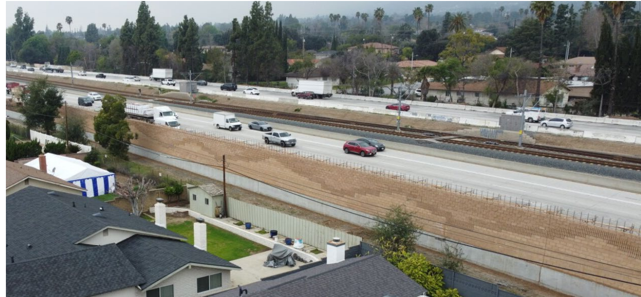
West view of masonry soundwall segment.
