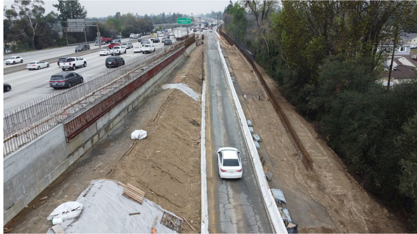
After pile install, rebar, concrete barrier.
