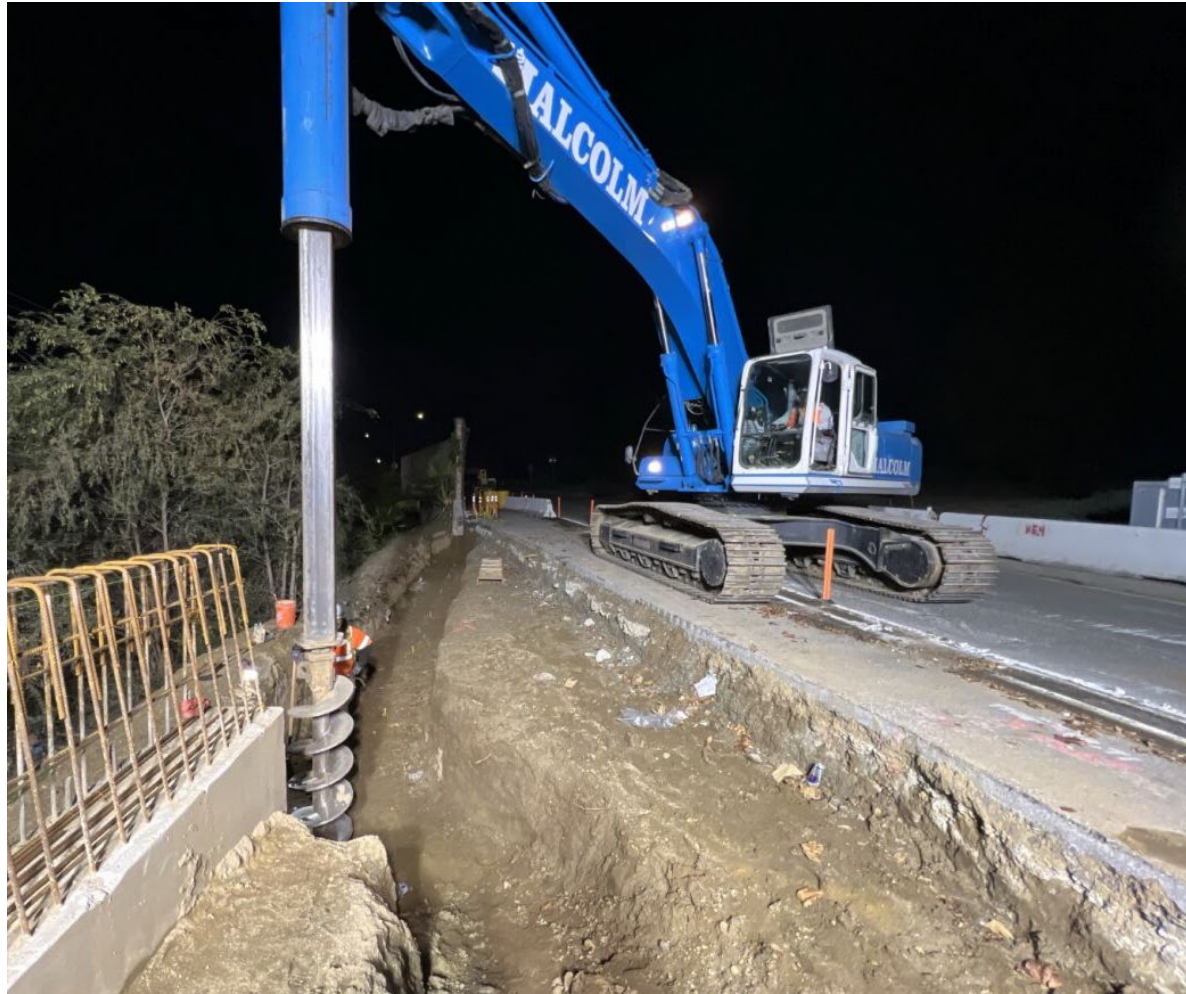
Pile drill along eastbound SR-134.
