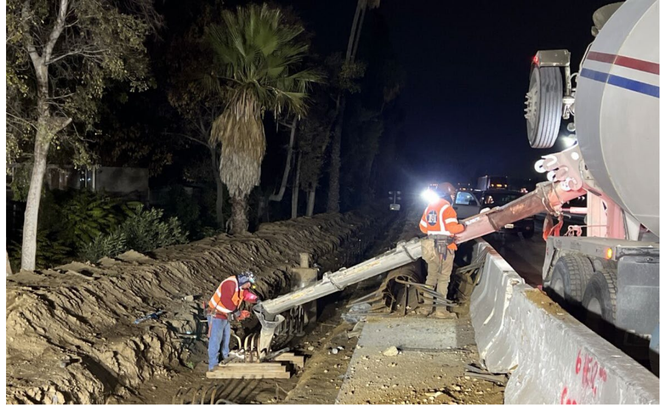
Pile rebar cages and concrete placement.
