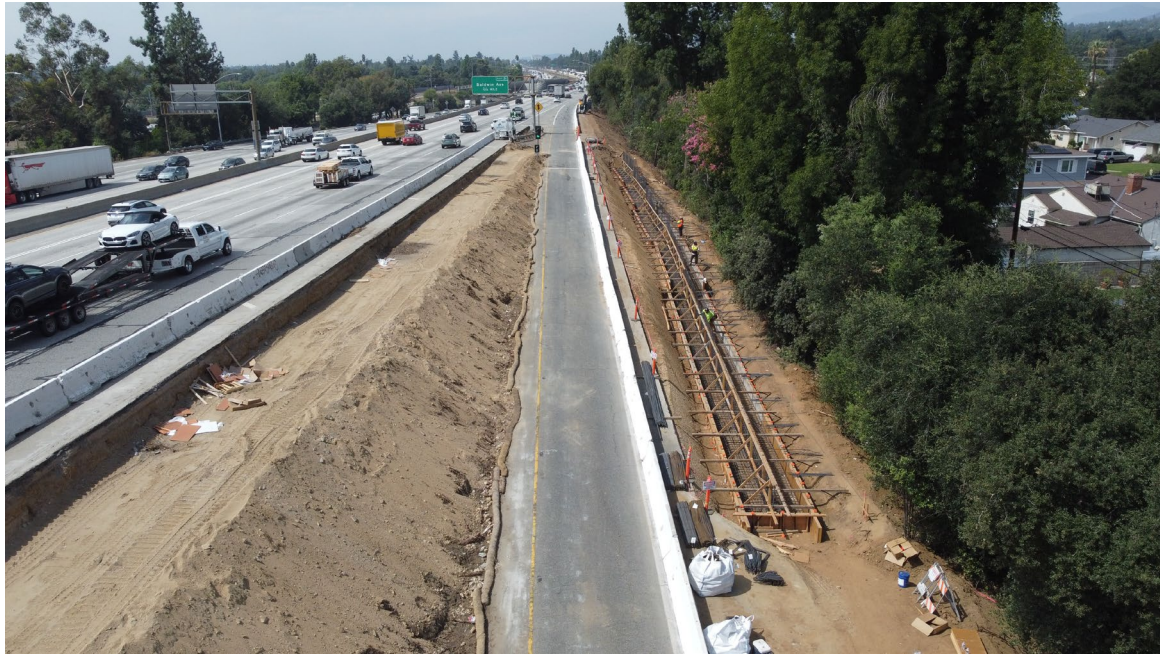
Before pile install, rebar, concrete barrier placement.
