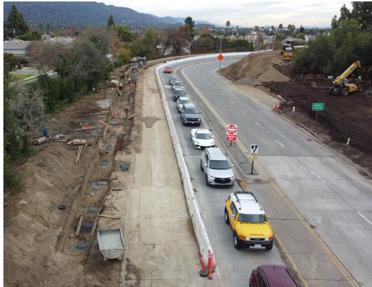
Pile installation at WB Santa Anita Av.
