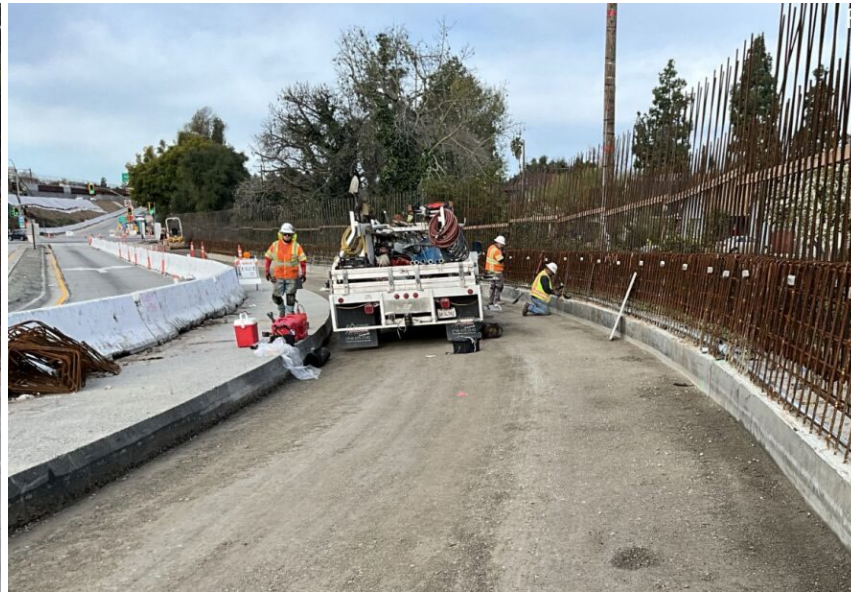
Grading, concrete, rebar work.
