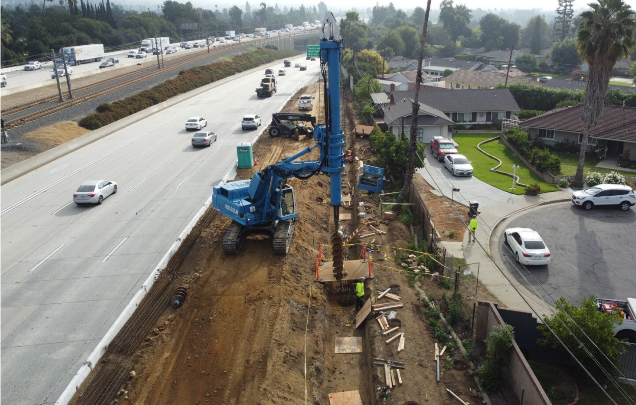
East view of pile installation from 2023.
