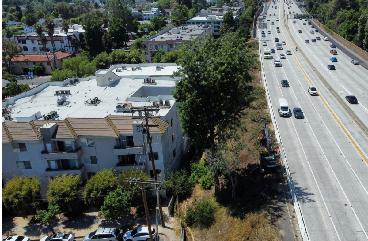
West view of SR-134 before clear, grub, demo operations.
