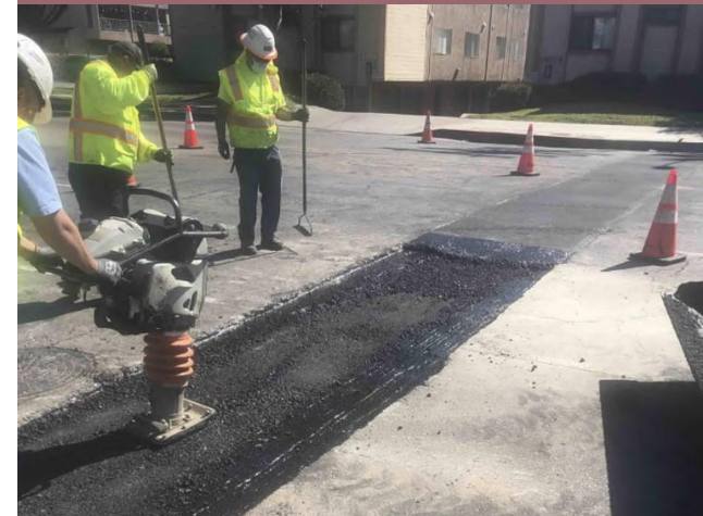
Street pavement restoration near Van Nuys Bl & Arleta Av
