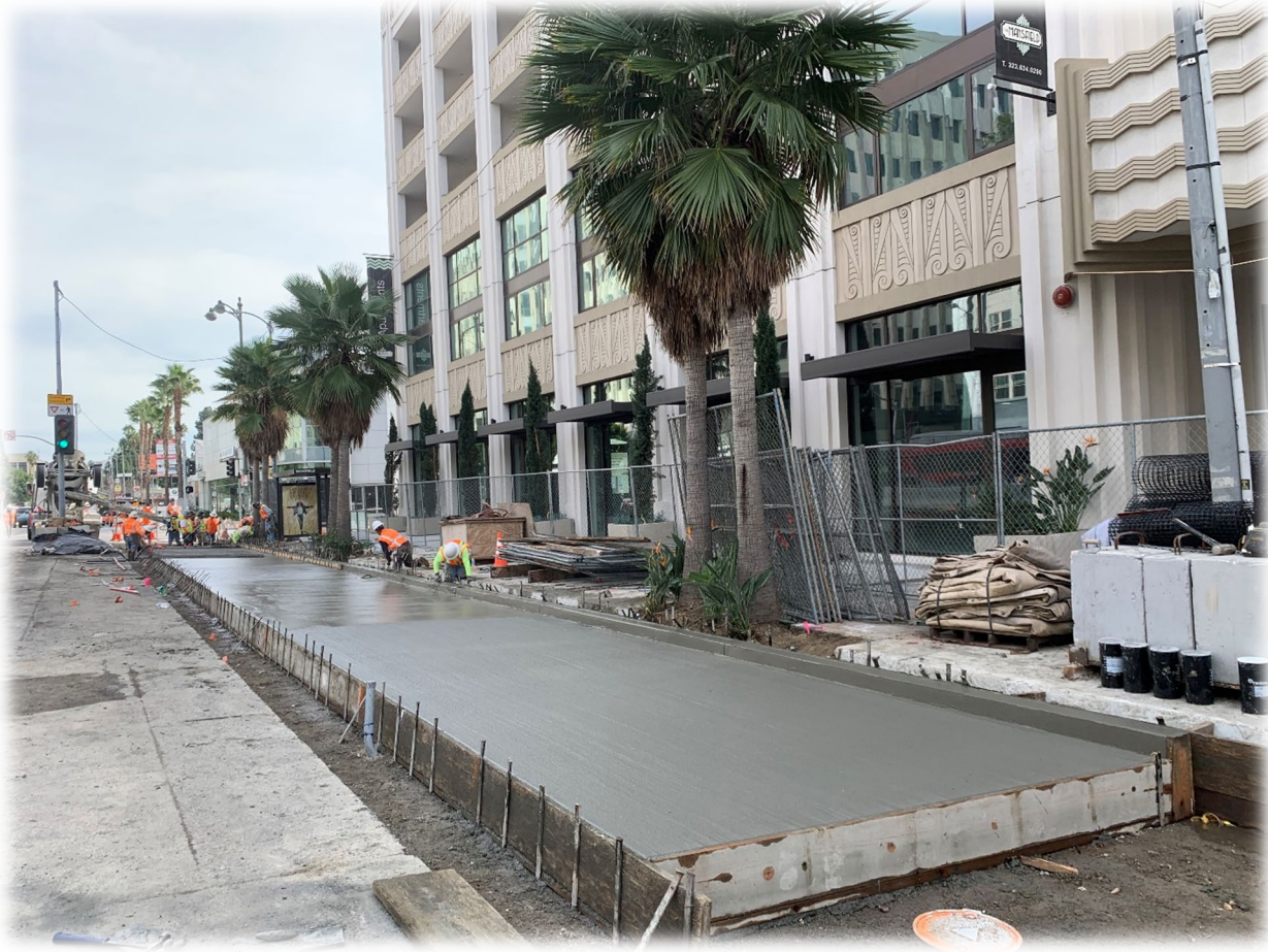
Poured Bus Pad Section between Mansfield Av and Orange Dr
