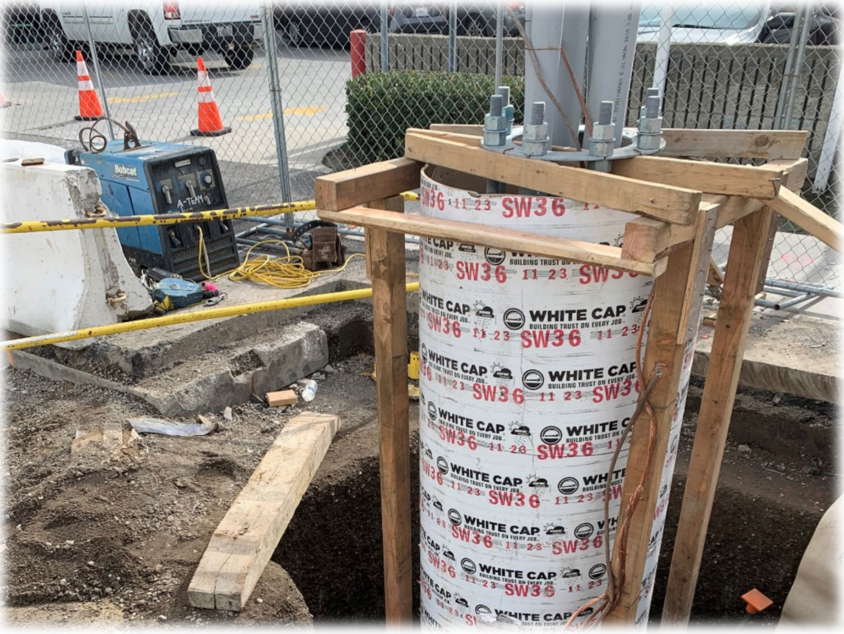
Foundation for the radio antenna at Wilshire/Sycamore
