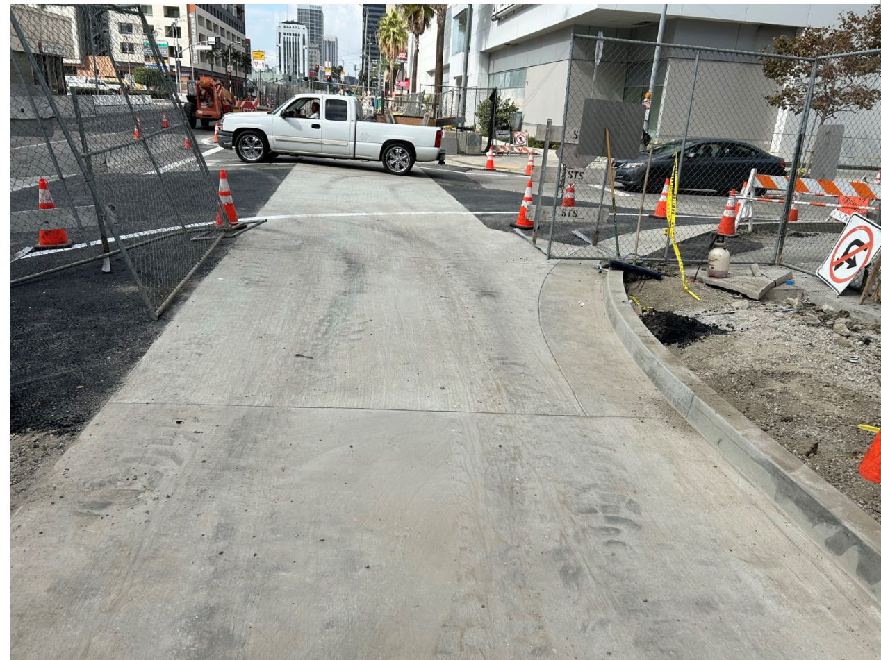
Finished Bus Pad and Curb at Wilshire/Orange
