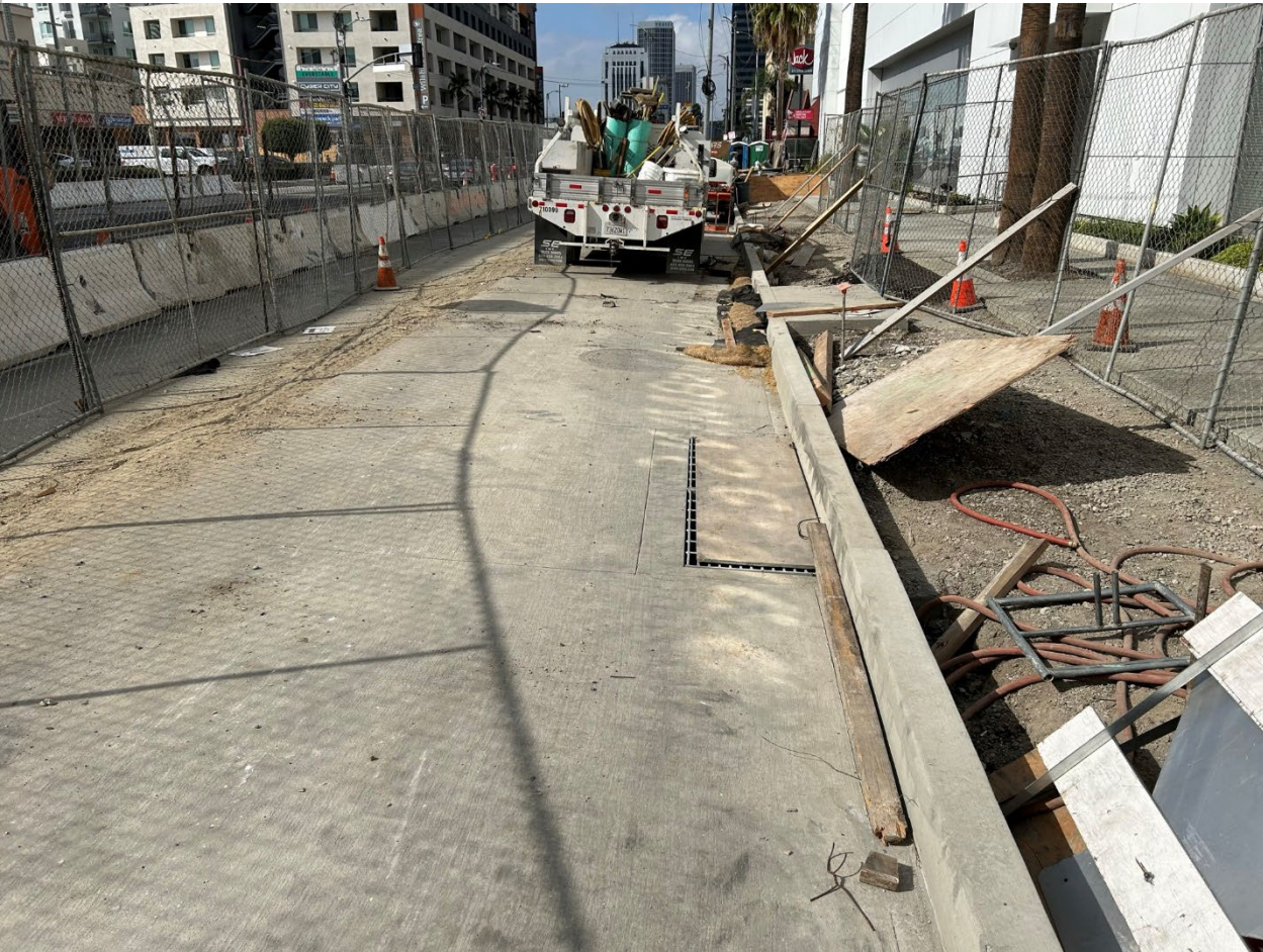
Finished Bus Pad and Curb on Wilshire – between Orange Dr and Sycamore Av
