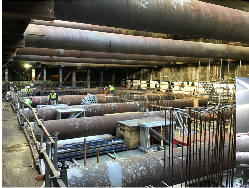
Left two photos – Progress work on Concourse Level (Falsework & Rebar)
