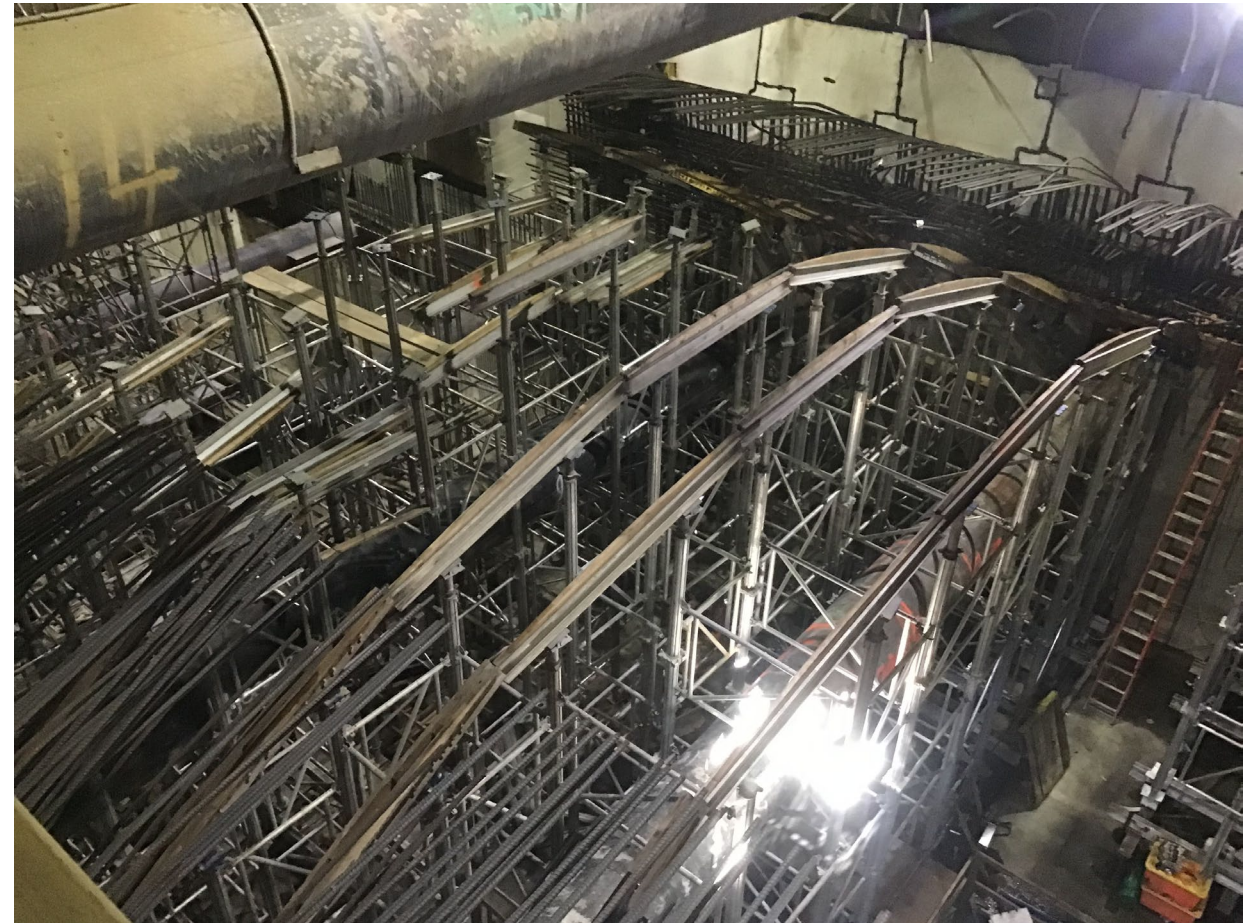
Concourse Roof Falsework Installation Progress
