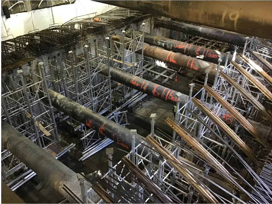
Station roof falsework
