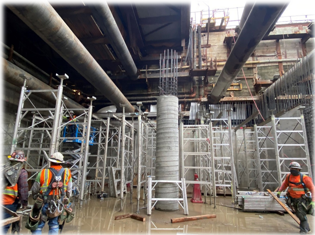
M Metro Entrance Structure
