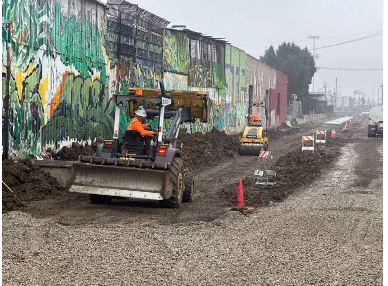
Grading gravel and spreading CMB for compaction
