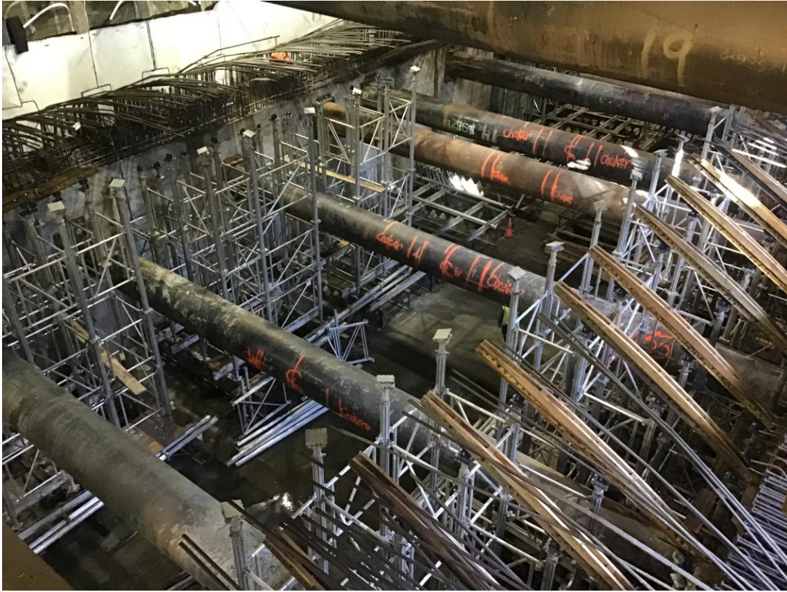
Station roof falsework
