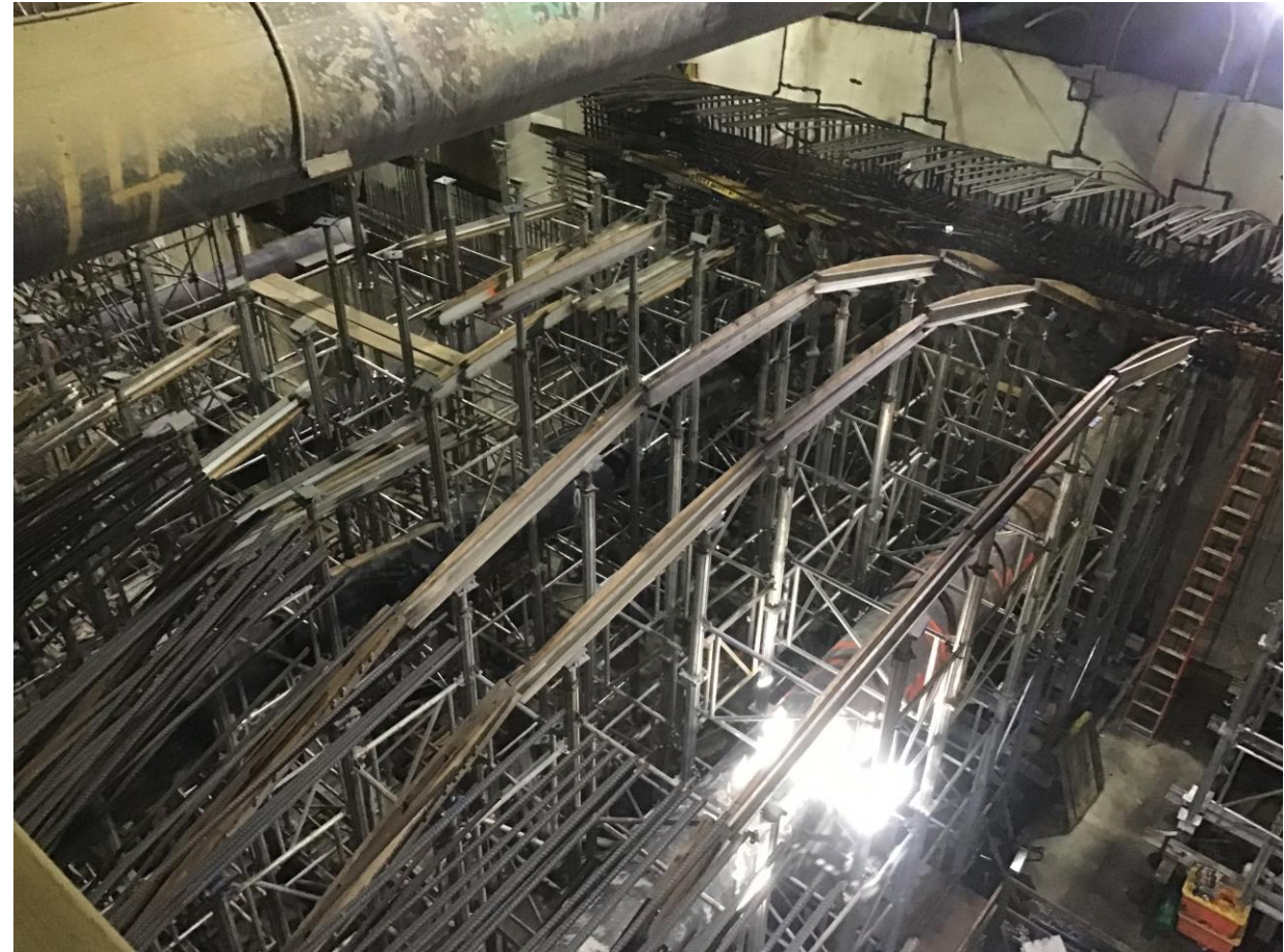
Concourse Roof Falsework Installation Progress
