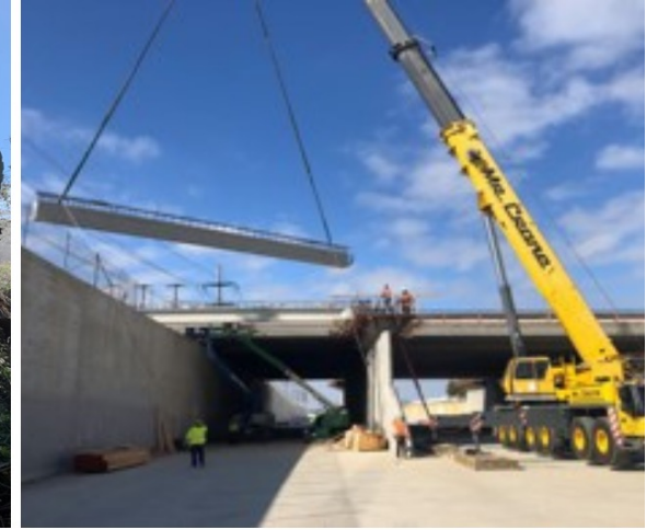
Above: Ongoing excavation at existing Rye Canyon Undercrossing Bridge; Example of girder installation
