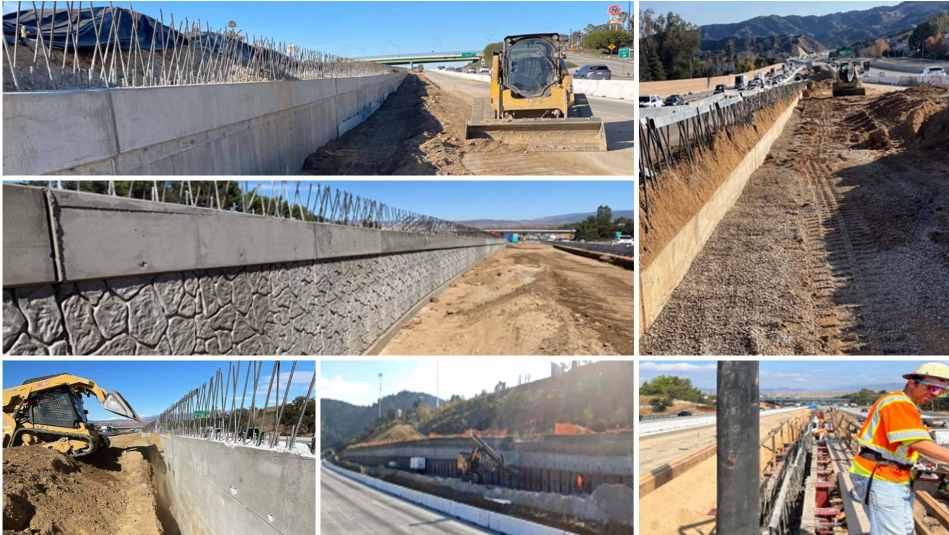
Center median construction activities including excavation, rebar, concrete, and backfill work.
