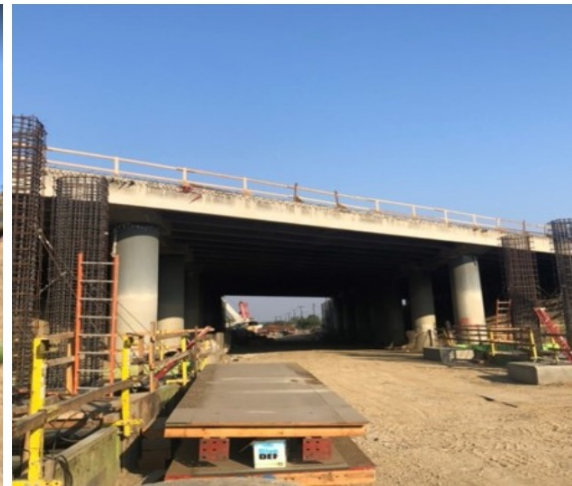
Above: Calgrove Bl Undercrossing bridge; Examples of column and falsework construction
