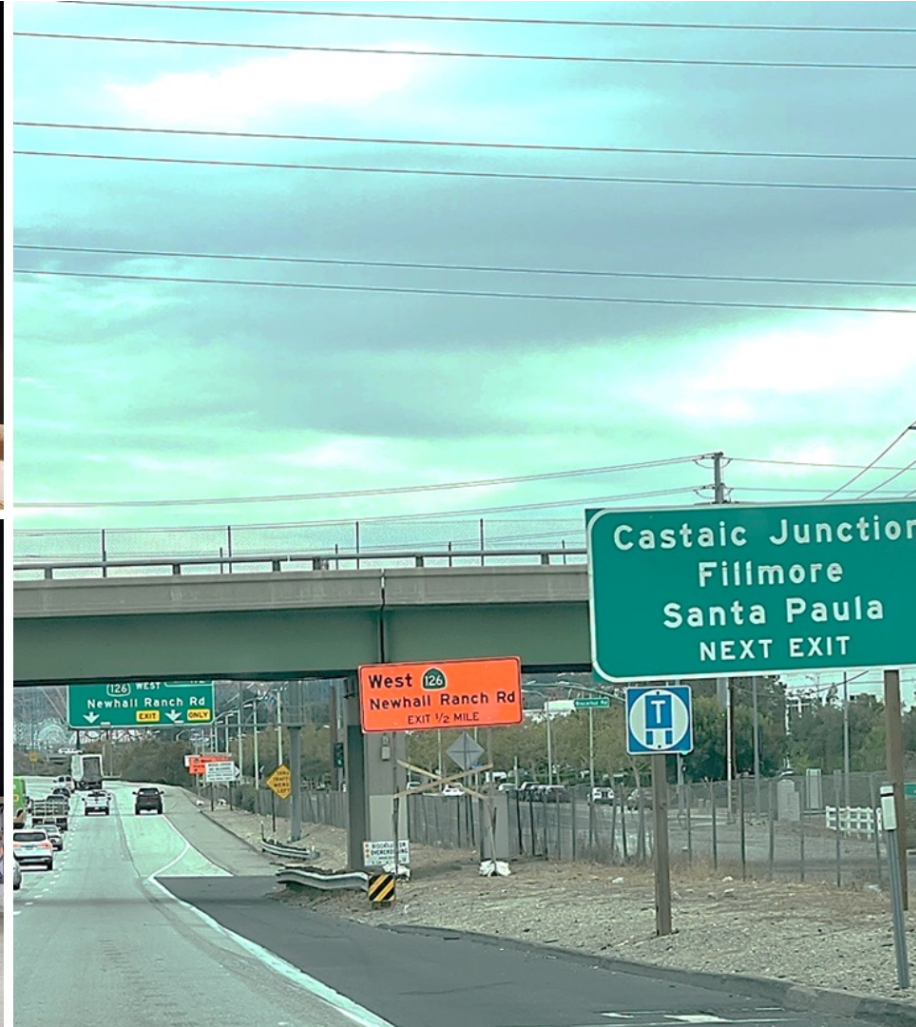
Temporary signage at Southbound I-5 outside shoulders
