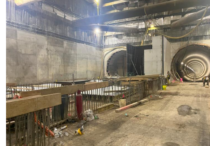
Track level looking east
