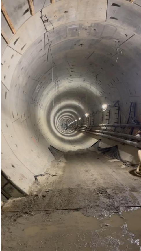
Tunnel Eye looking west
