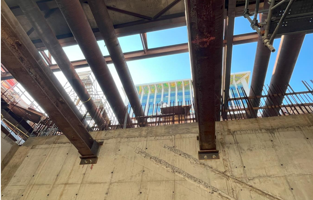
Station Entrance (future location of entrance escalator)
