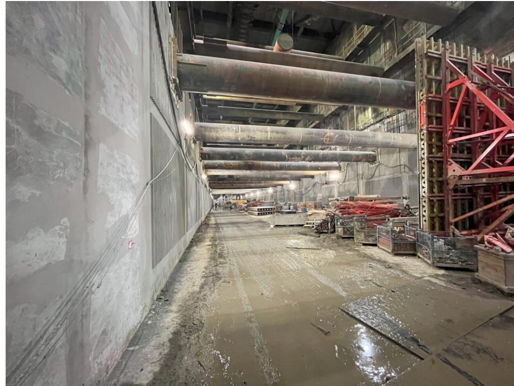
Track level looking west
