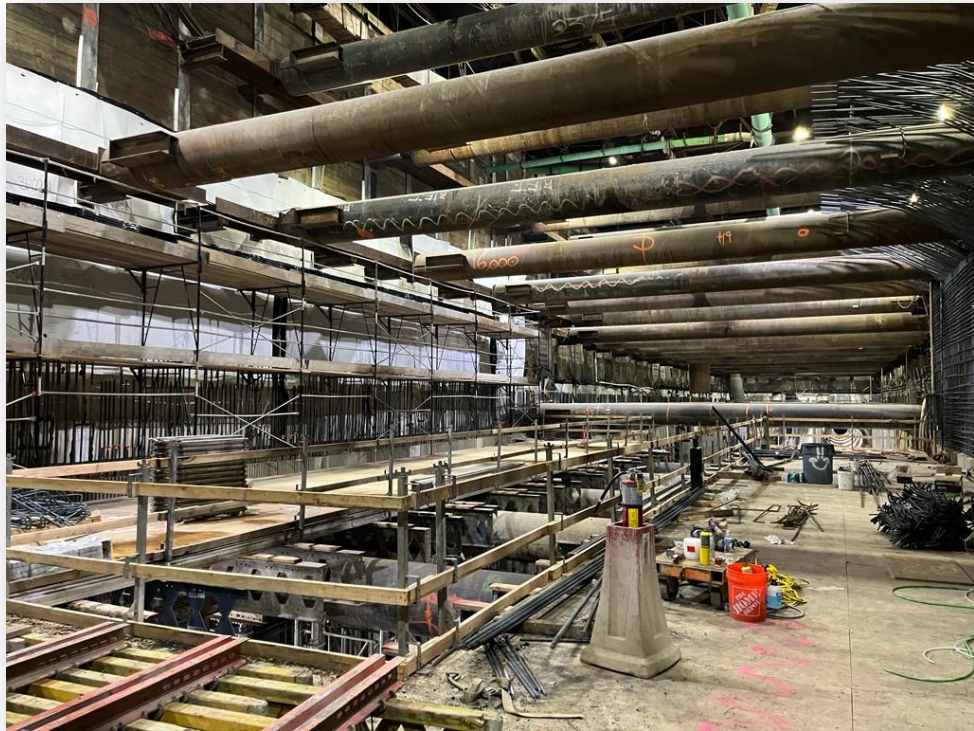
Concourse Level looking west
