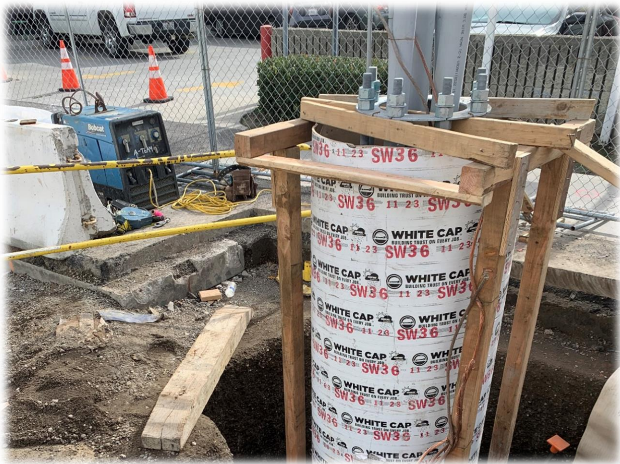
Foundation for the radio antenna at Wilshire/Sycamore
