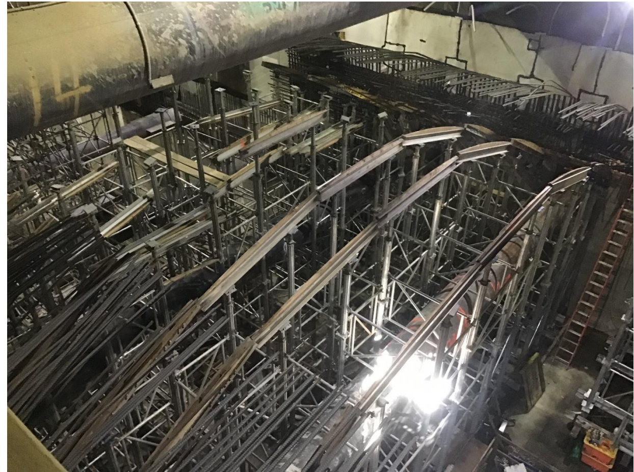
Concourse Roof Falsework Installation Progress
