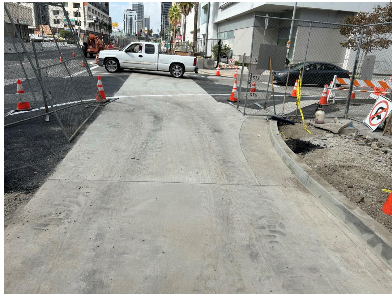
Finished Bus Pad and Curb at Wilshire/Orange
