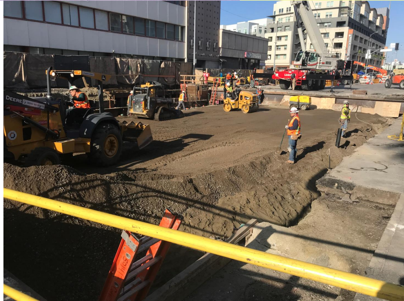
Backfilling operations at Wilshire Bl and Orange Dr, within the City of Los Angeles
