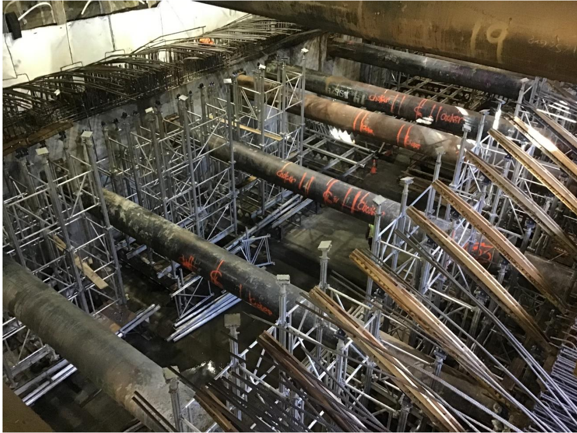
Station roof falsework
