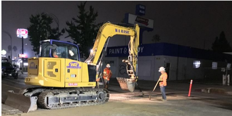
Lateral work activity near Van Nuys Bl and Hartland St.
