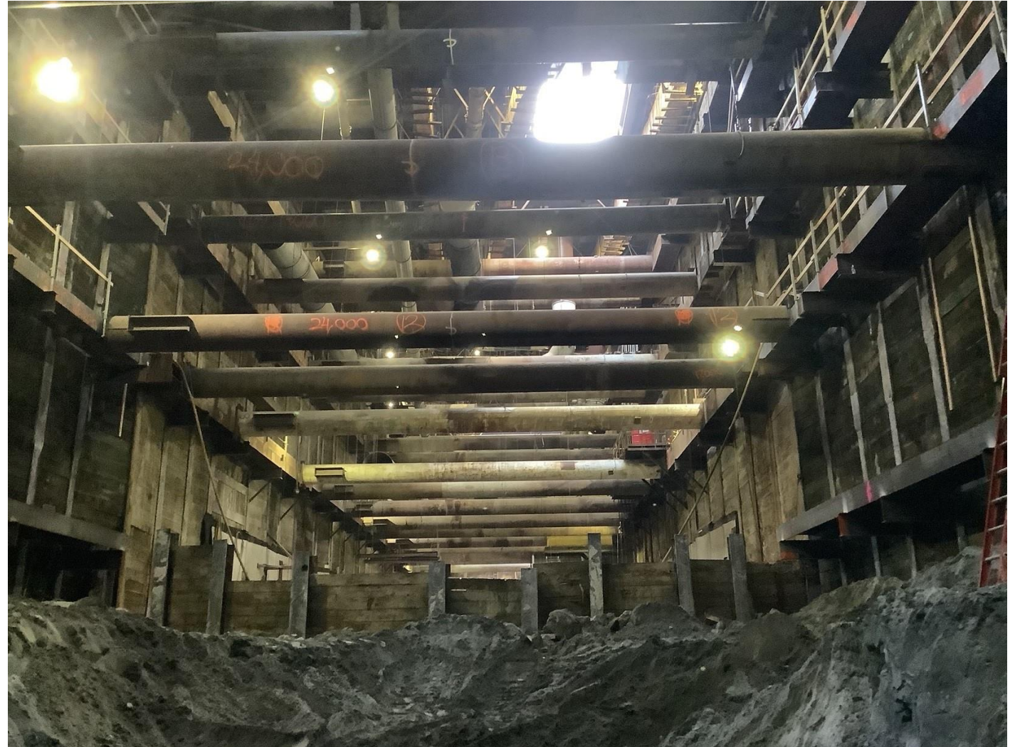
Station looking East
