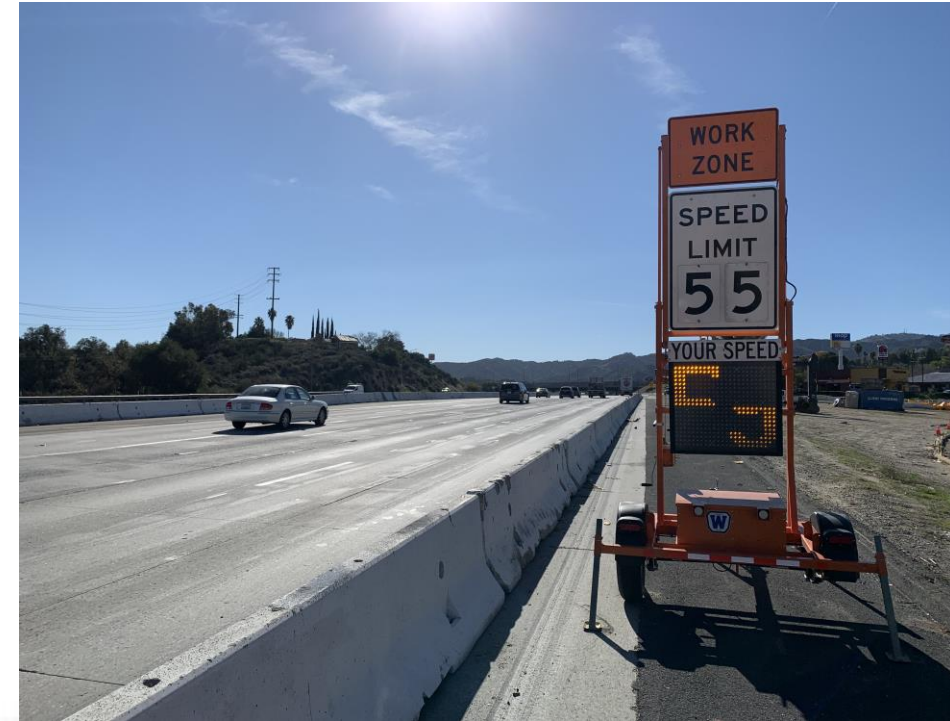
Work zone speed limit signage
