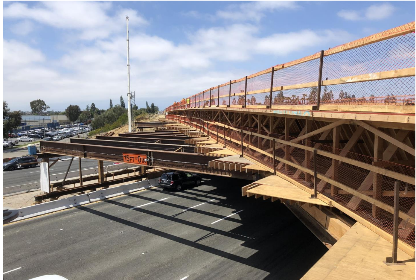
Example of bridge falsework – I-405 Improvement Project, Orange County
