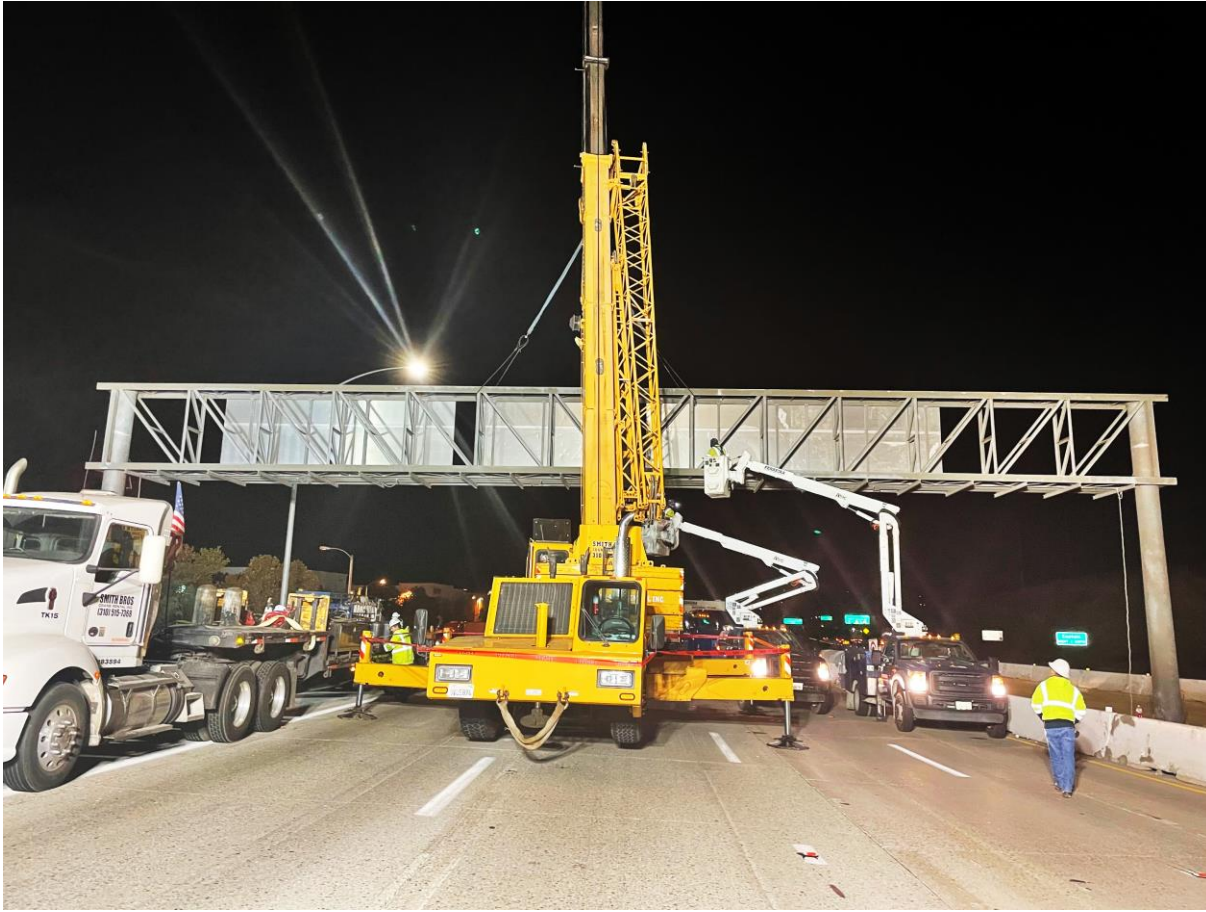
Crews preparing to remove existing overhead signage with crane
