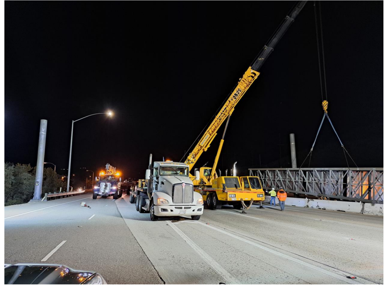
Overhead signage removed and placed in center median
