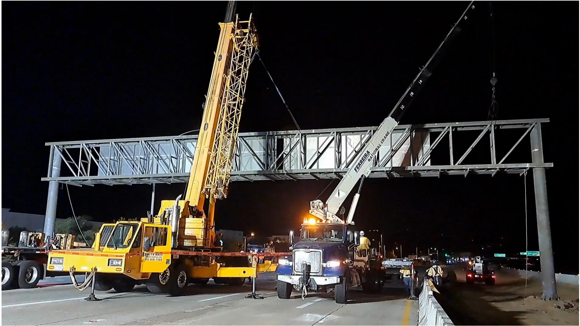
Video footage of Southbound overhead sign being removed
