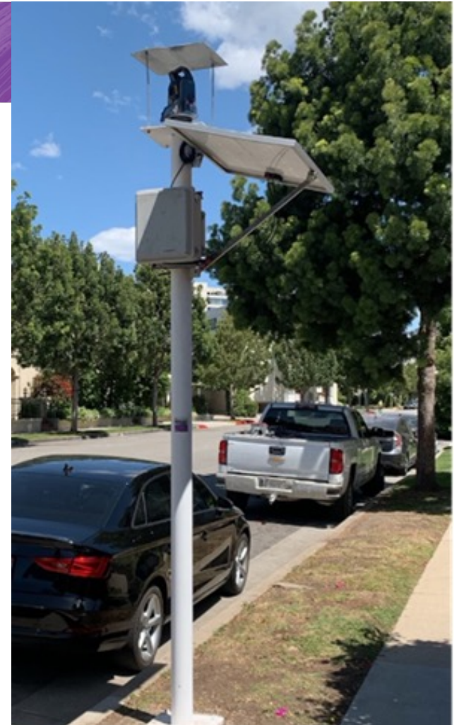
Example of 10-foot geotechnical instrumentation pole.
