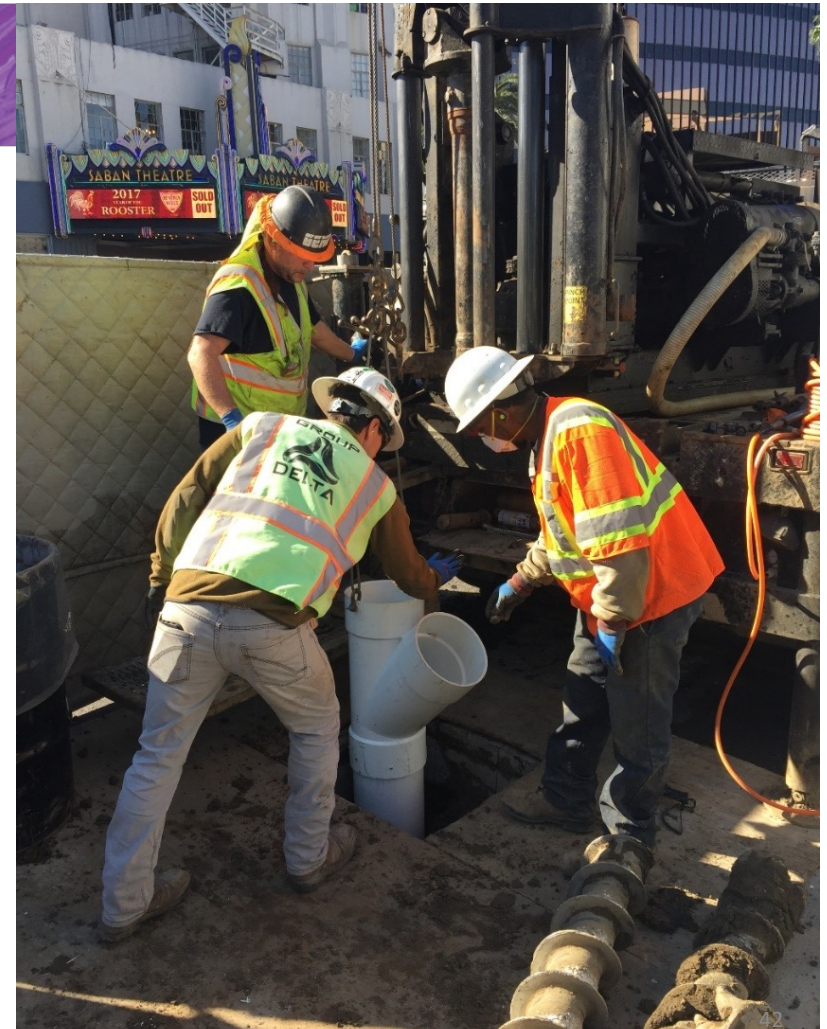
Example of instrumentation drilling
