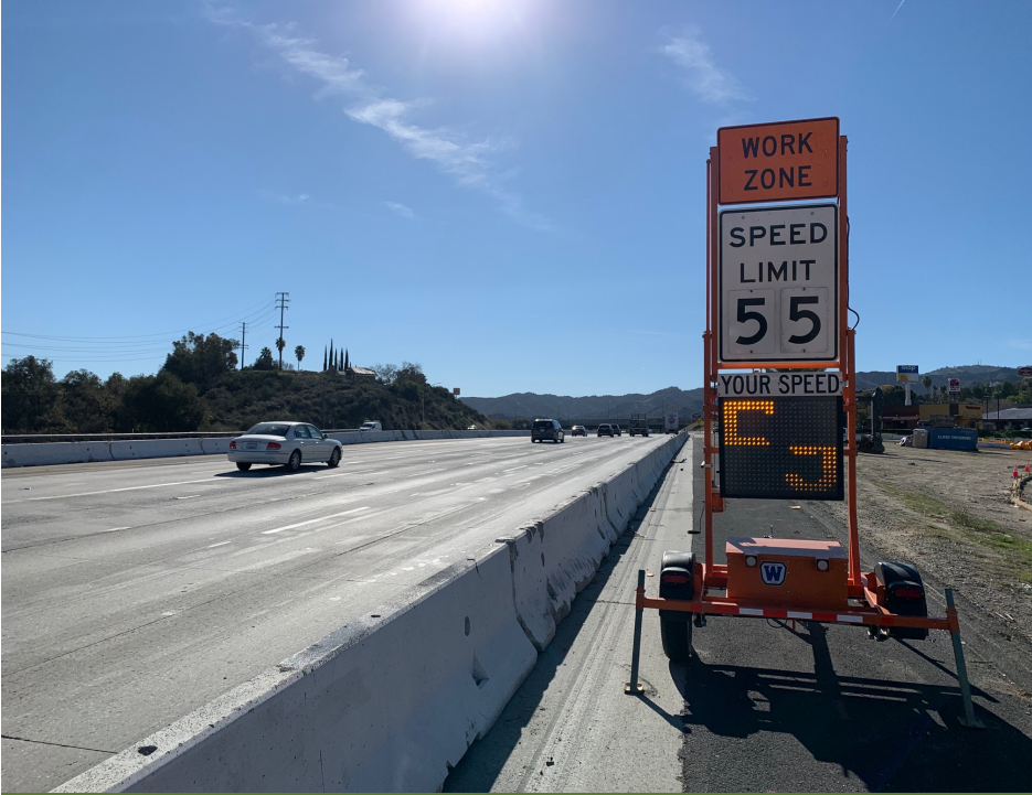
Work zone speed limit signage
