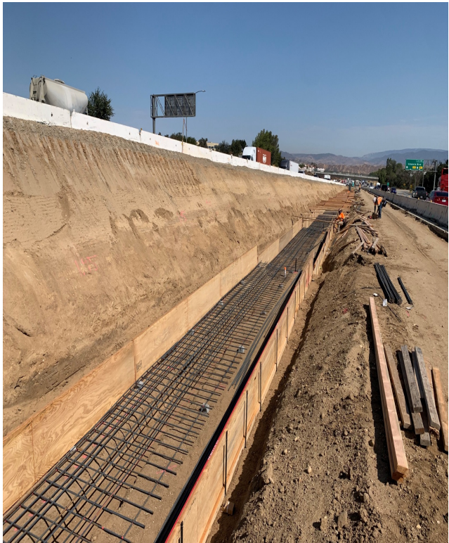
Project-wide center median construction: activities include drainage installation, retaining wall work, sign structure, pavement and concrete work
