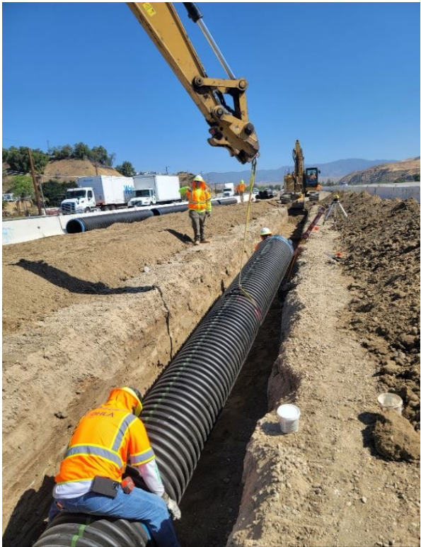
Project-wide center median construction: activities include drainage installation, retaining wall work, sign structure, pavement and concrete work
