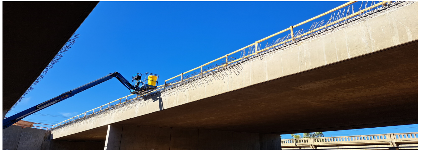
Castaic Creek Bridge progress photos as of August 2022
