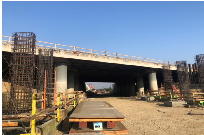
Examples of column and girder construction from the I-405 Improvement Project
