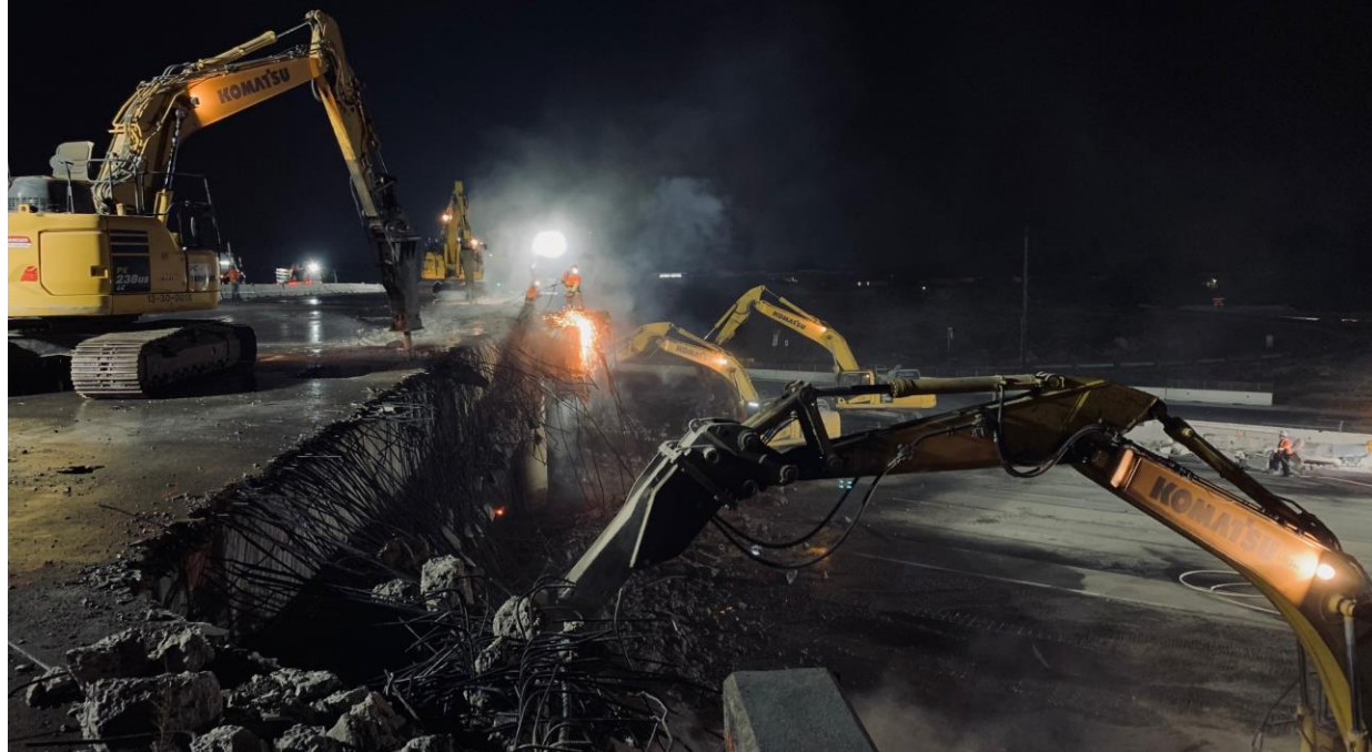
Controlled bridge demolition using excavators with hydraulic breaker extensions
