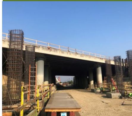
Example of column construction
