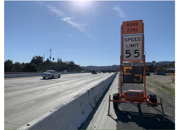
Work zone speed limit signage
