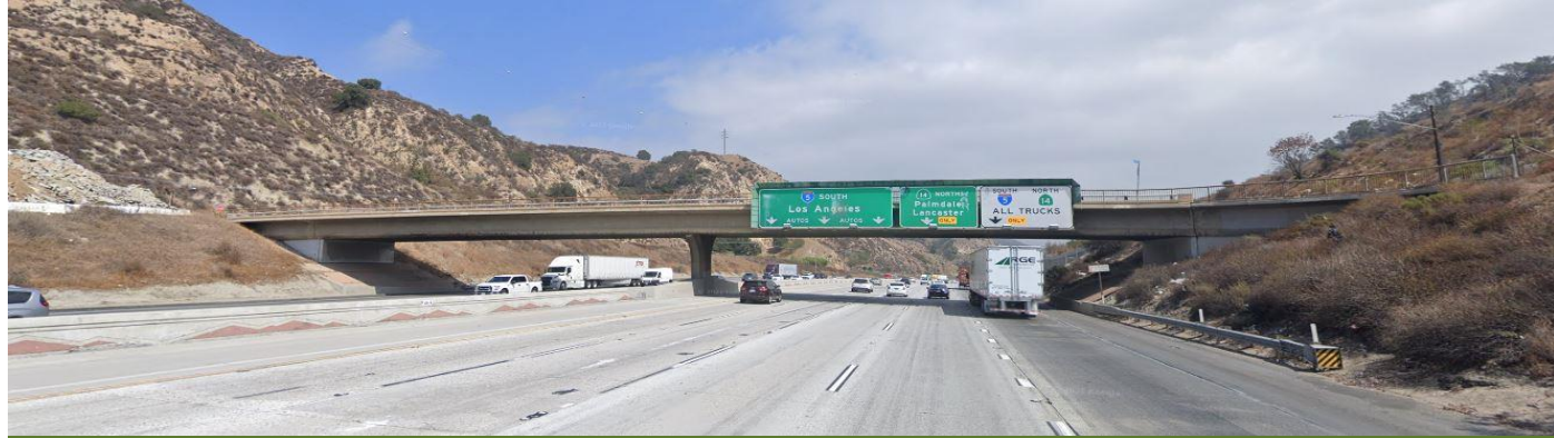
Existing Weldon Canyon Overcrossing bridge
