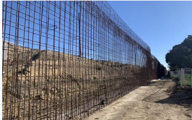
Example of rebar construction
