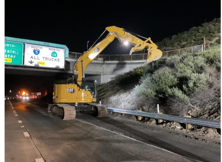
Performing vegetation removal at SR-14 & I-5 split
