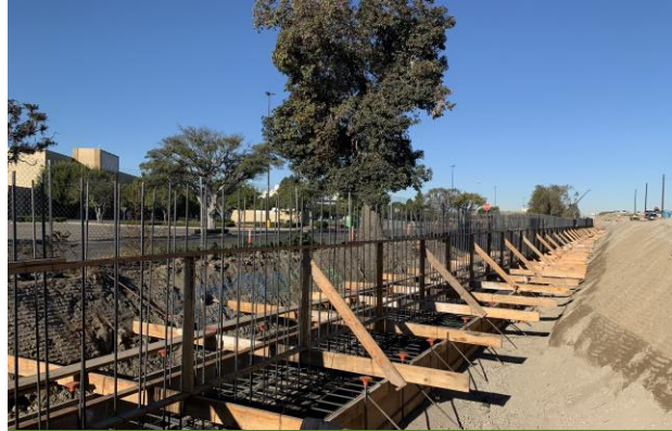
Example of retaining wall footing construction
