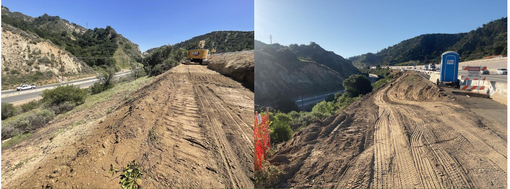
Completed vegetation removal between SR-14 and Calgrove Bl
