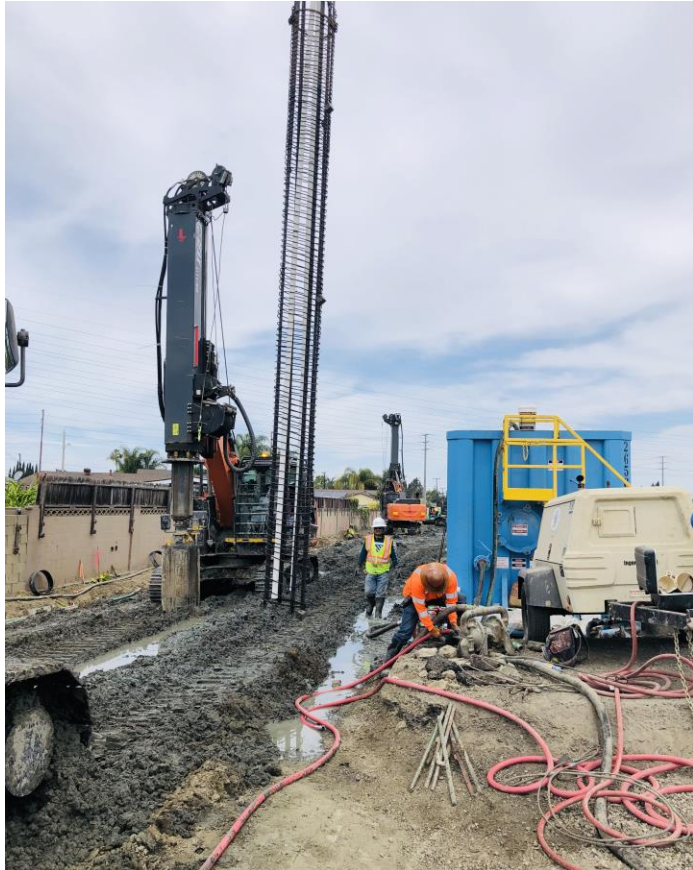
Steel pile driving
