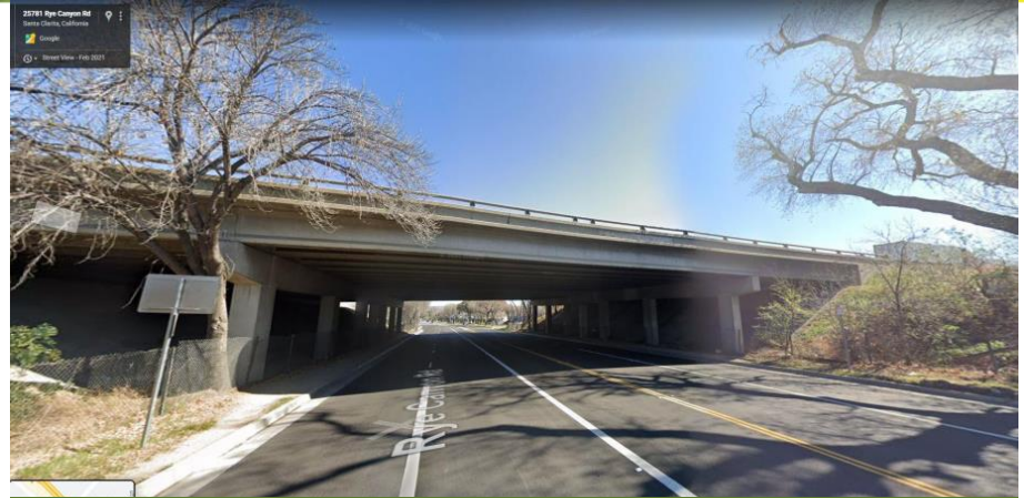
Existing Rye Canyon Undercrossing Bridge
