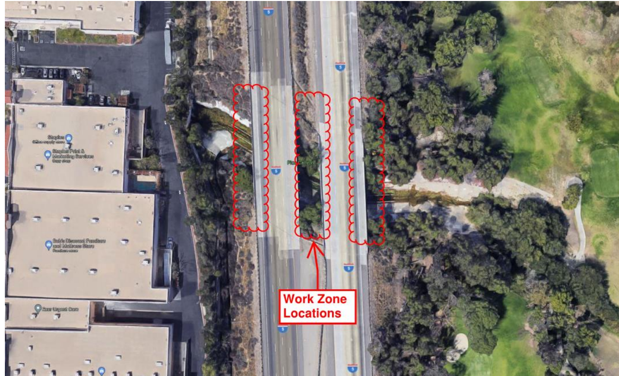
Work zone at Butte Canyon Bridge
