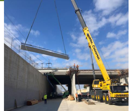
Example of girder installation
