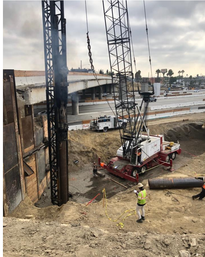
Concrete in drilled hole (CIDH) pile installation
