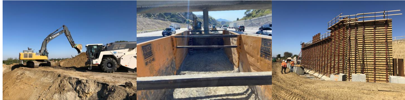
Examples of shoring, excavation, and abutment form construction activities
