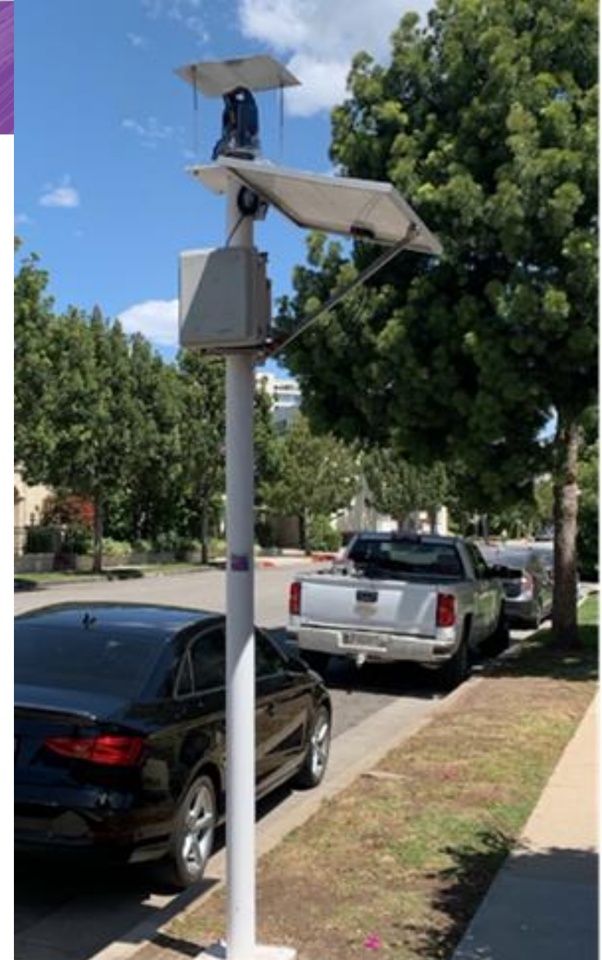
Example of 10-foot geotechnical instrumentation pole.
