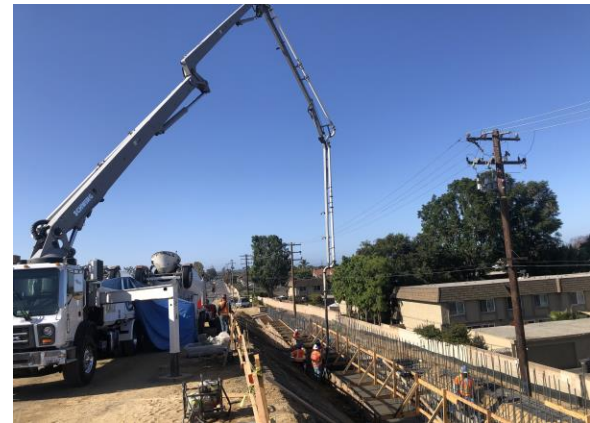
Sample photos: Typical freeway grading and concrete work
