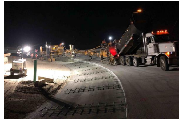
Sample photos: City street and ramp asphalt/concrete paving.
