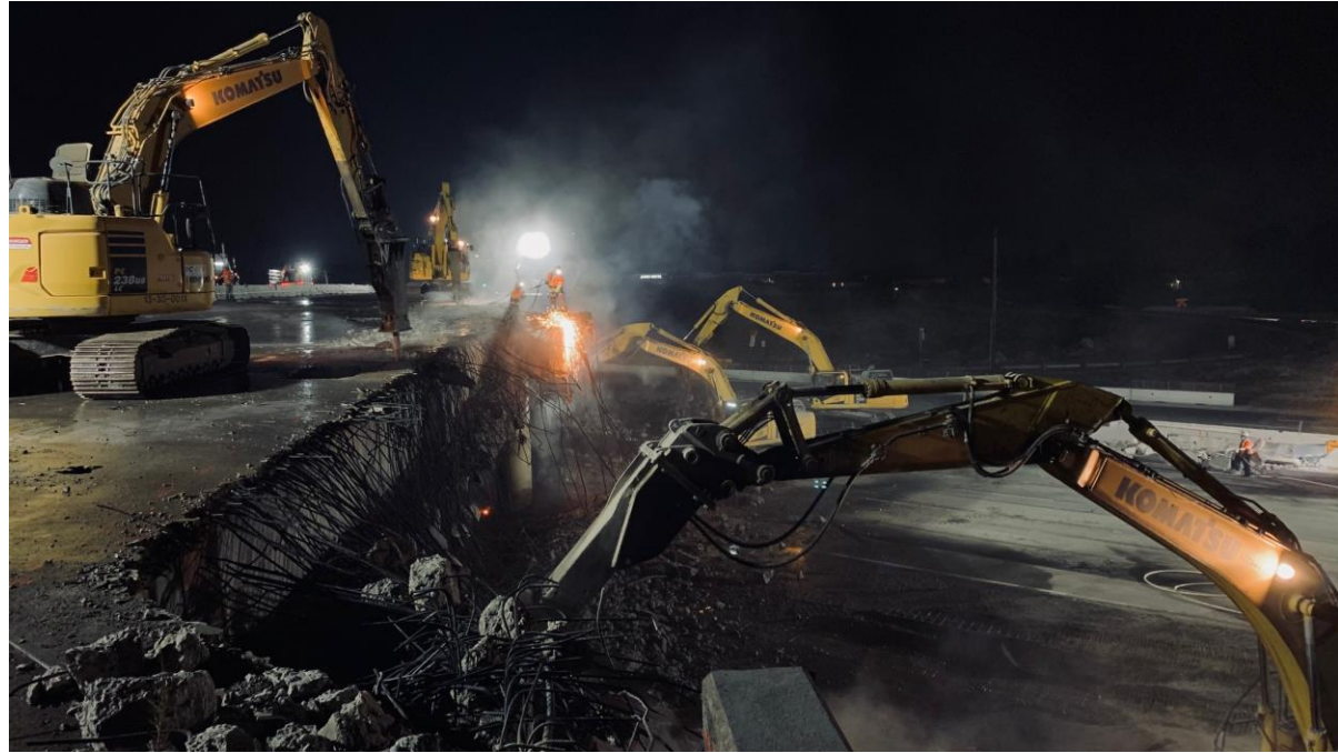
Sample photo: Controlled bridge demolition using excavators with hydraulic breaker extensions.
