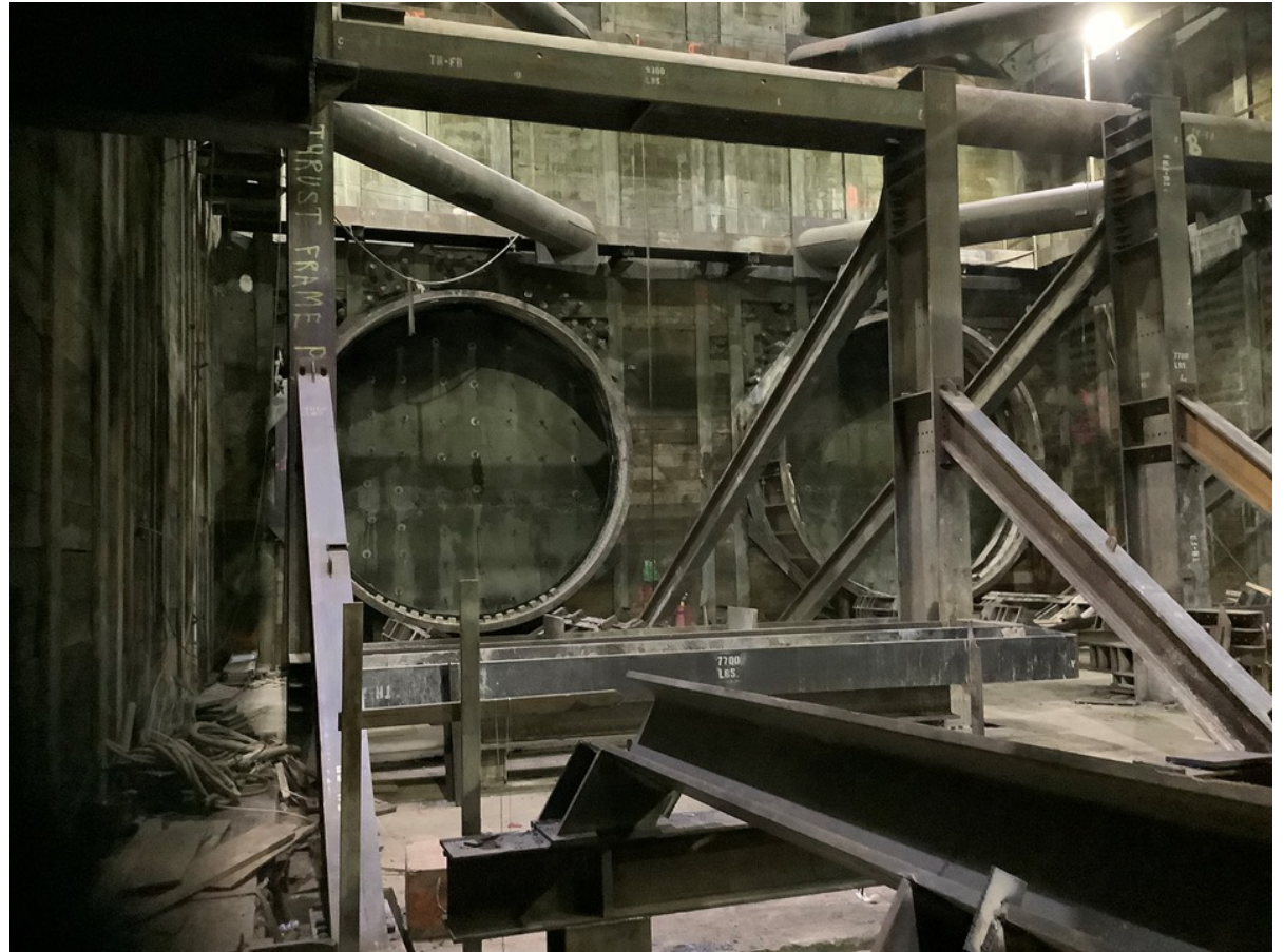
Progress of exterior wall installation.
