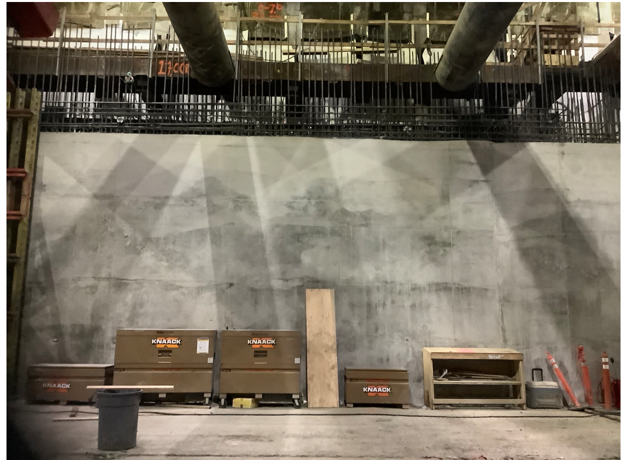
Progress of installing exterior walls.
