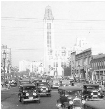
Wilshire and Vermont Avenue, 1934
