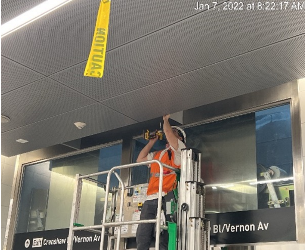
Adjusting ceiling panels above elevators
