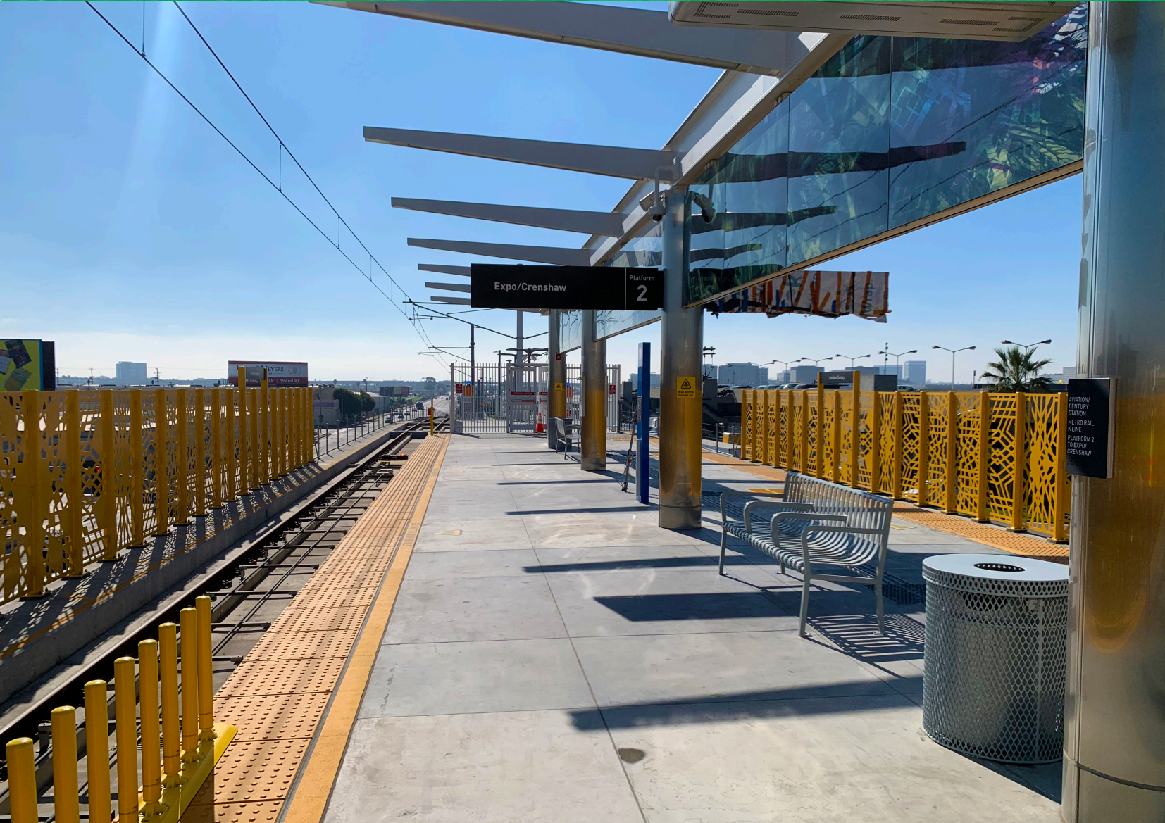
Station platform, signage, and benches
