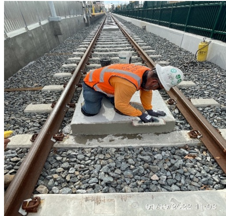
Sacking and patching rail vehicle pads along southbound track
