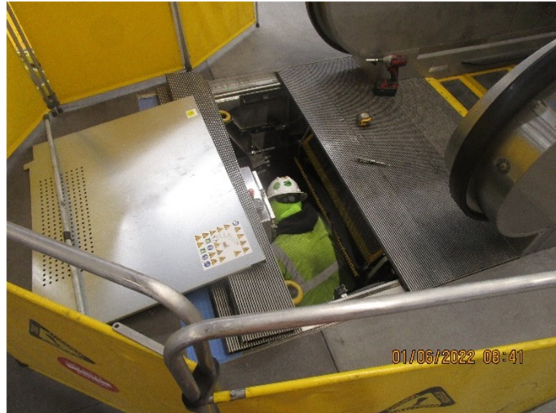
Adjustment of roller, belts and chain at pit of escalator
