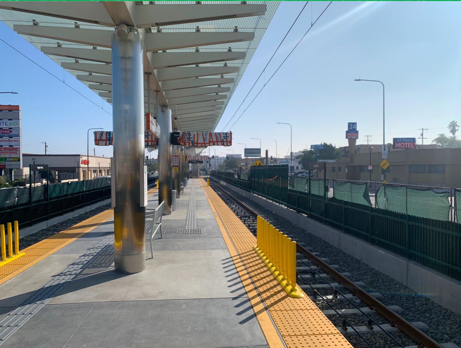
Station platform and tactile pavers
