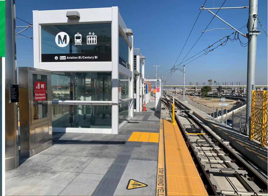
Elevator at platform level and railway track
