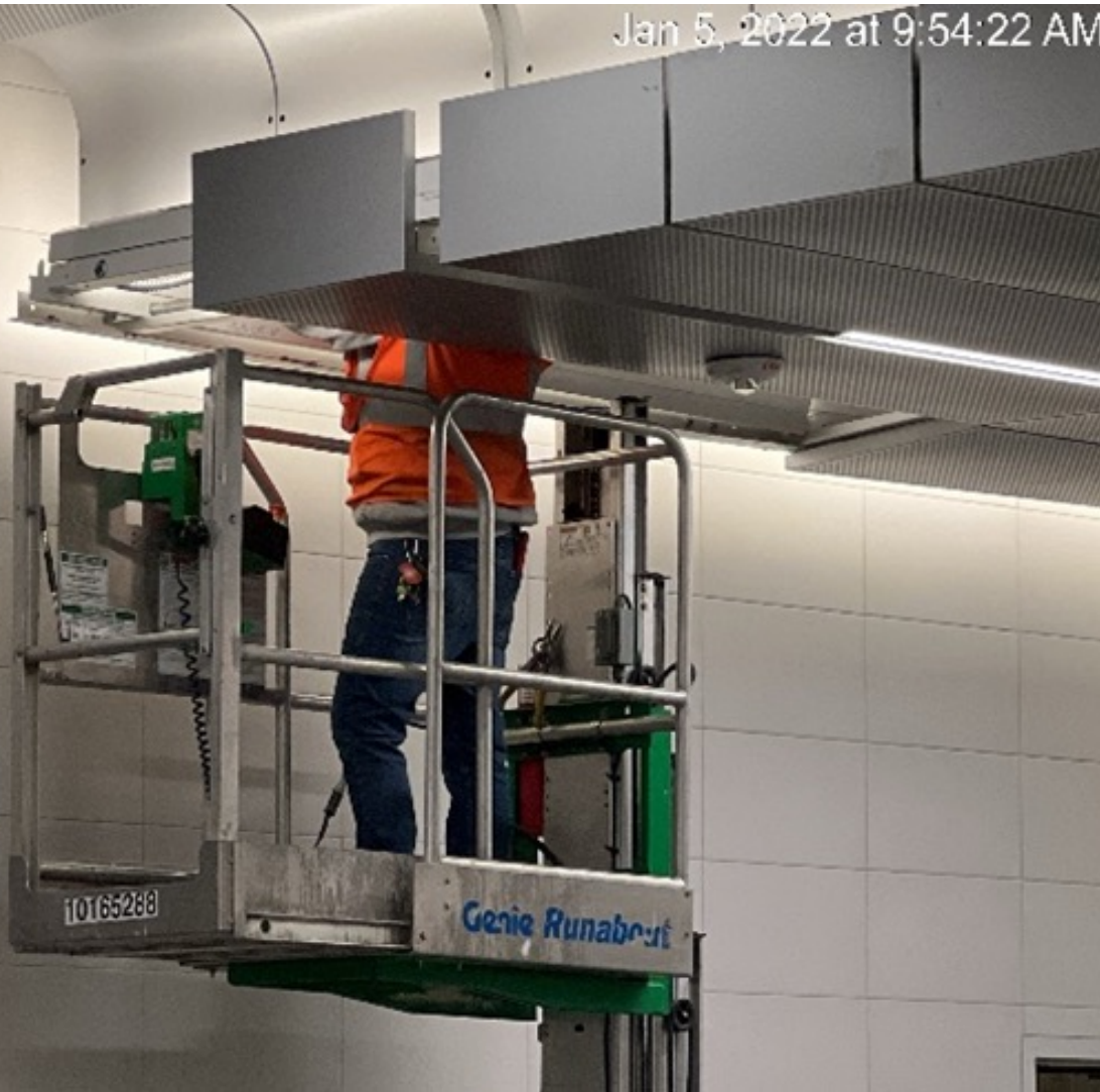
Adjustment of light cove ceiling at concourse area
