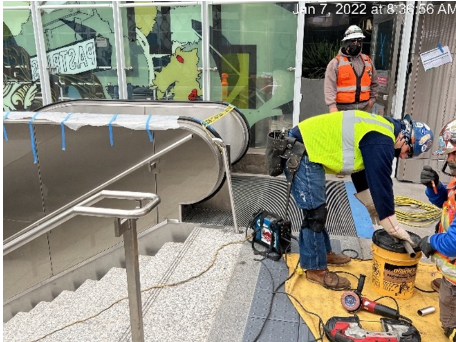
Welding handrails along exterior sides of escalators at main entrance
