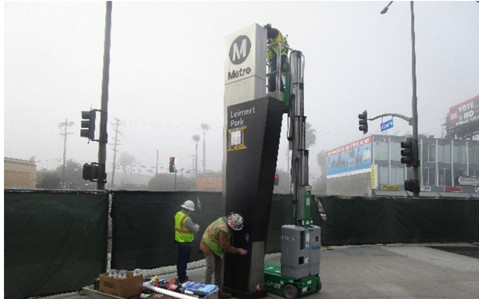
Cleaning and polishing the grand pylon sign at the Leimert Park Station plaza
