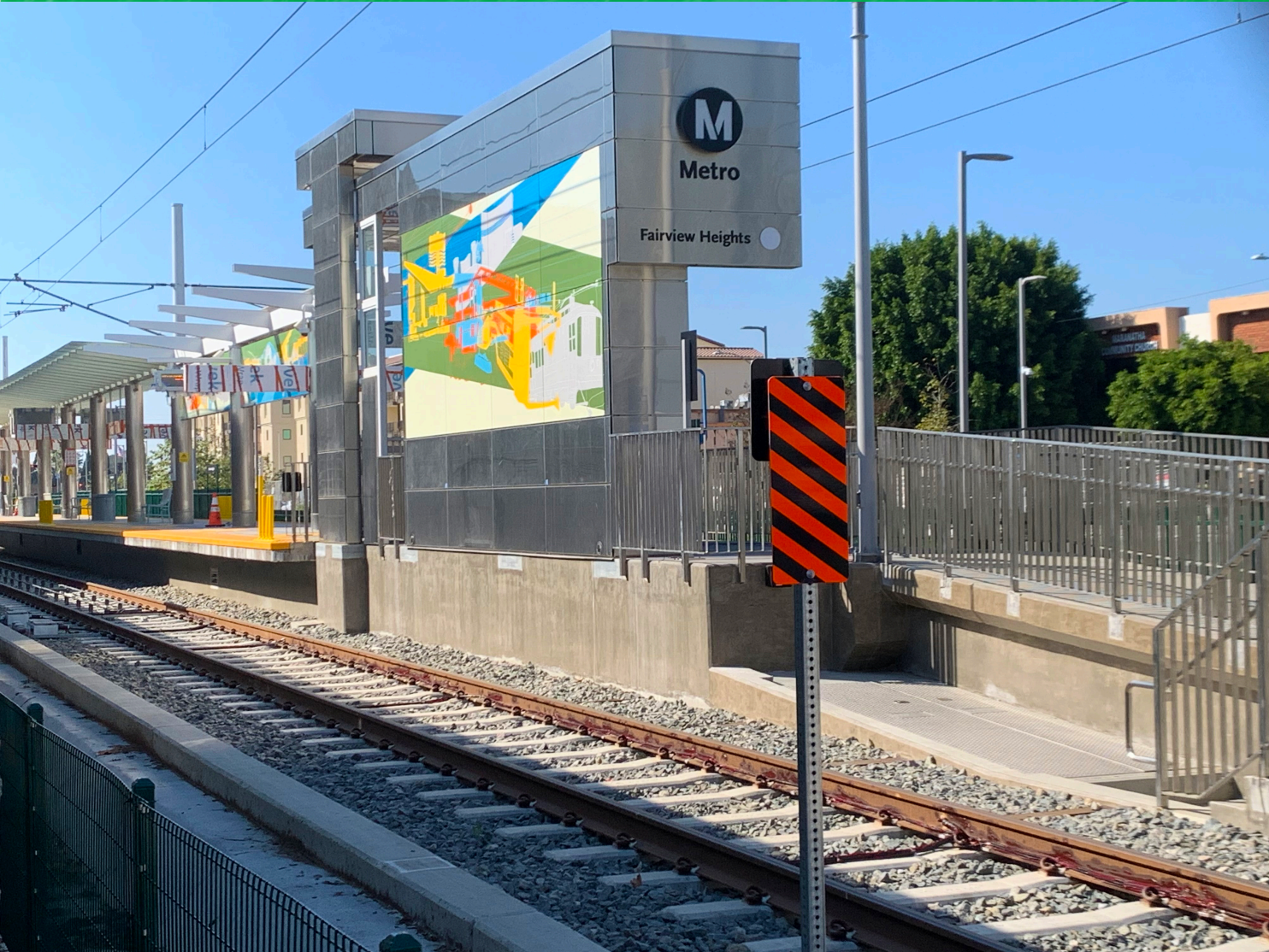
TVM canopy, railway track, station plaza, and installed porcelain enamel artwork
