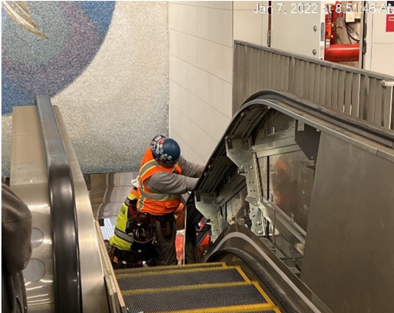
Installing cladding trim to escalator between concourse and platform
