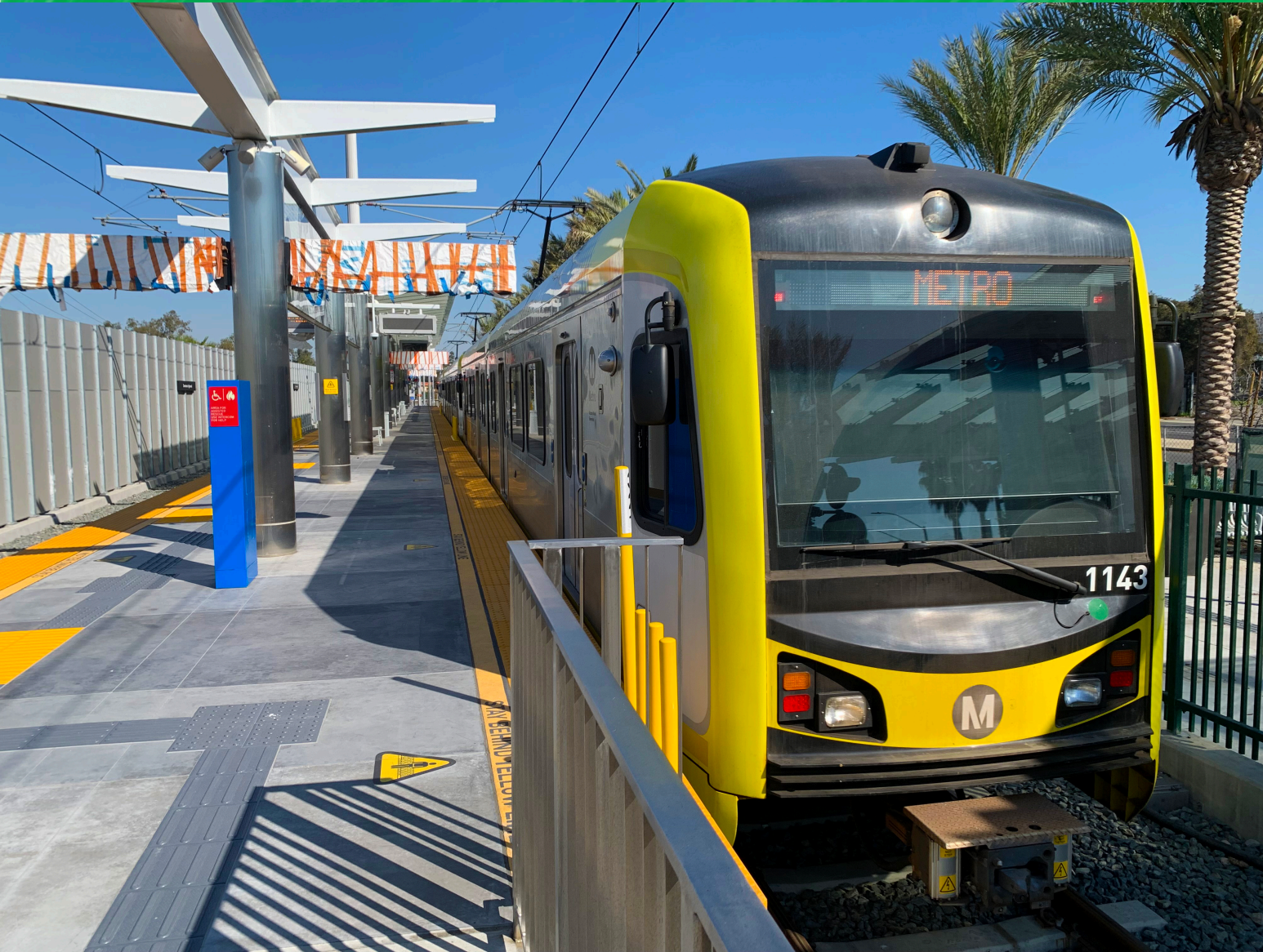
Station platform and installed signage
