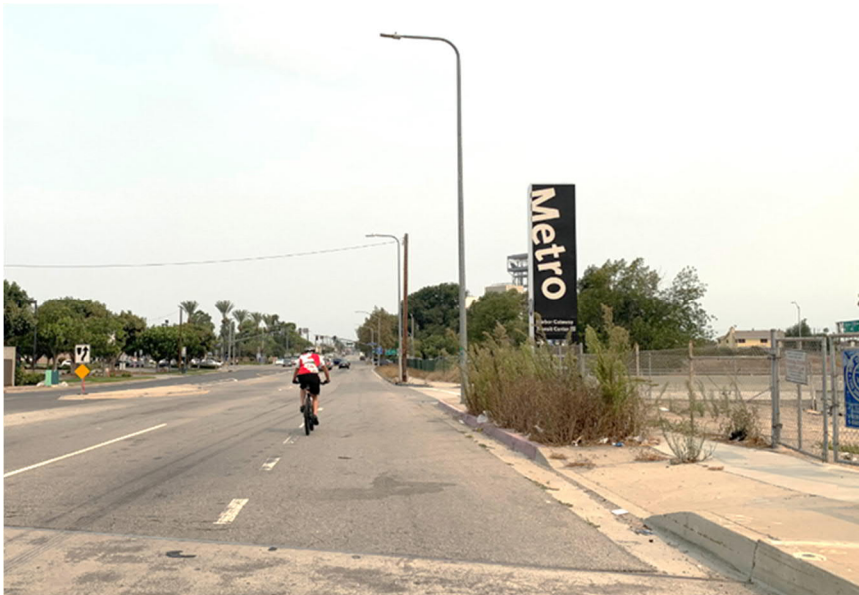
Figure ES.7: Gap in the Bike Lane on Vermont Avenue near the Harbor Gateway Transit Center
