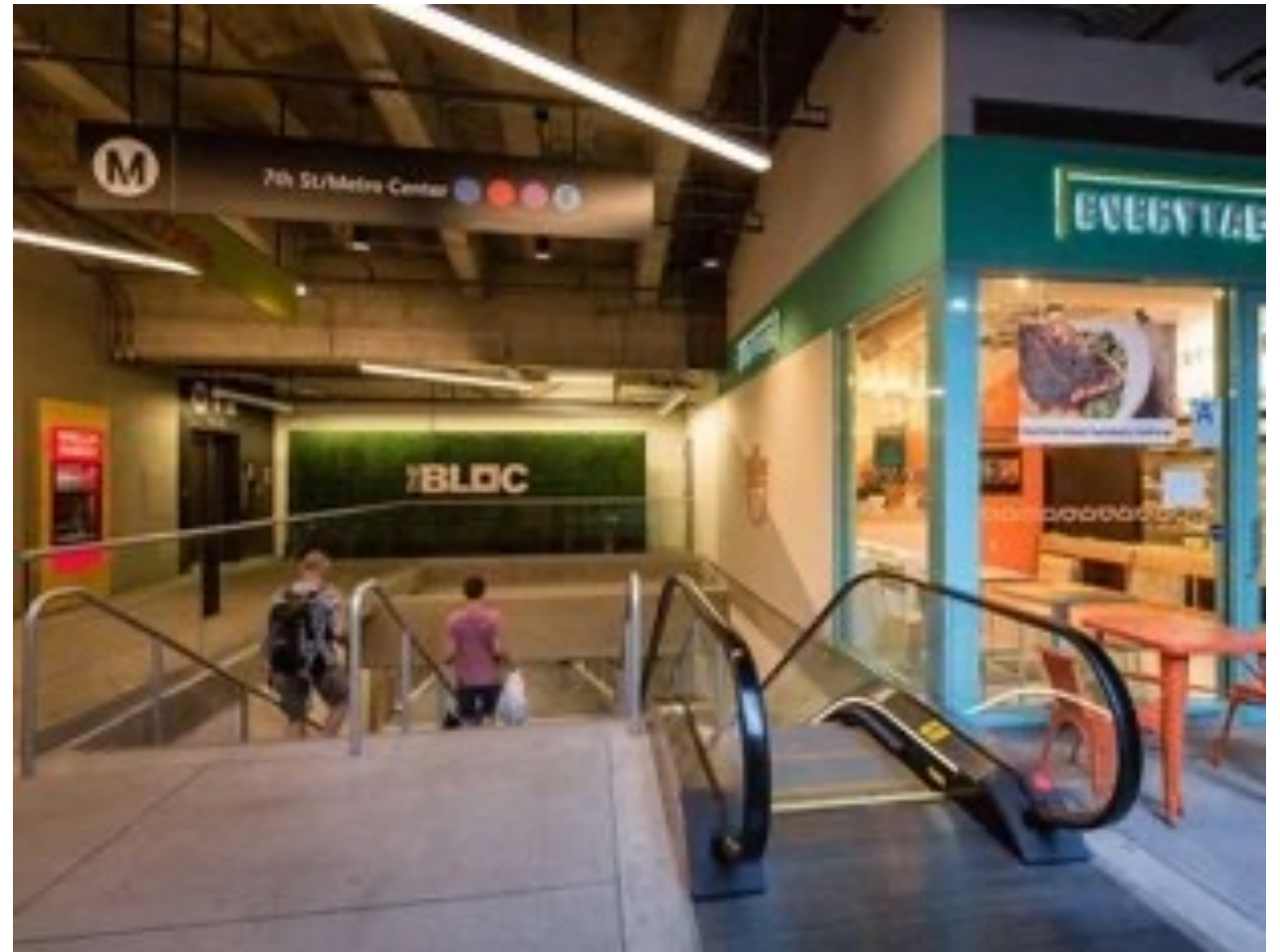
New station entrance at 7th Street/Metro Center Station using knock-out-panel (KOP) 24
