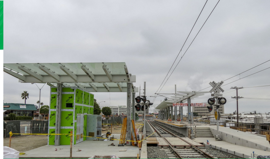
TVM canopy under construction
