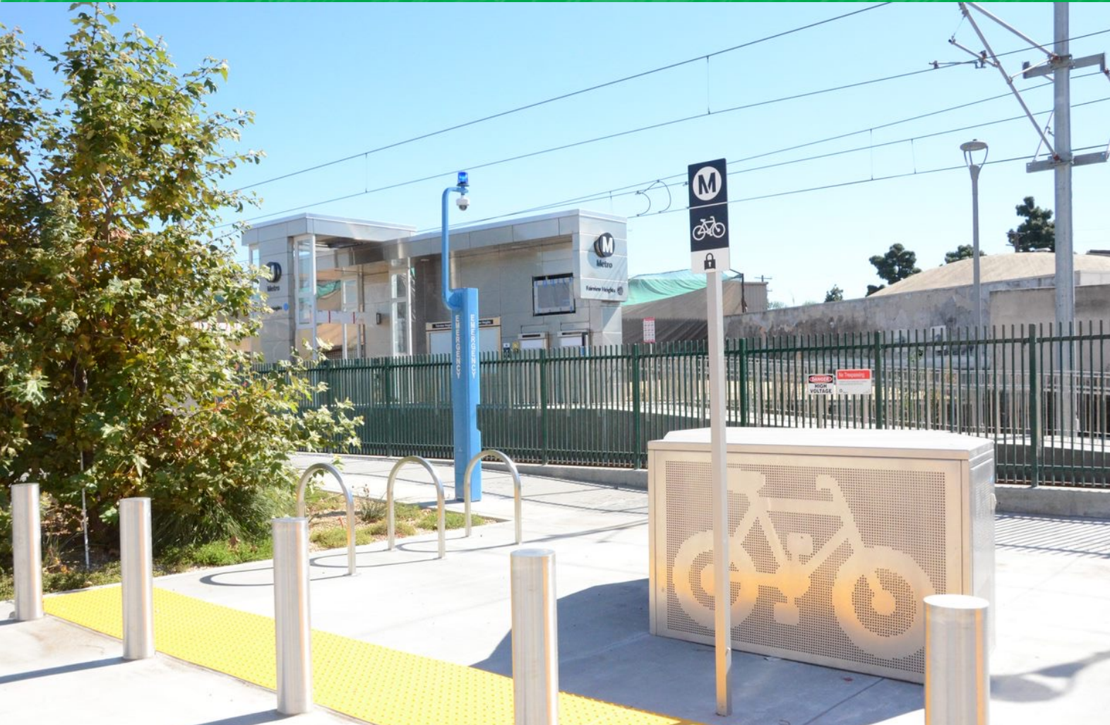
Ticket Vending Machine Canopy and bike locker
