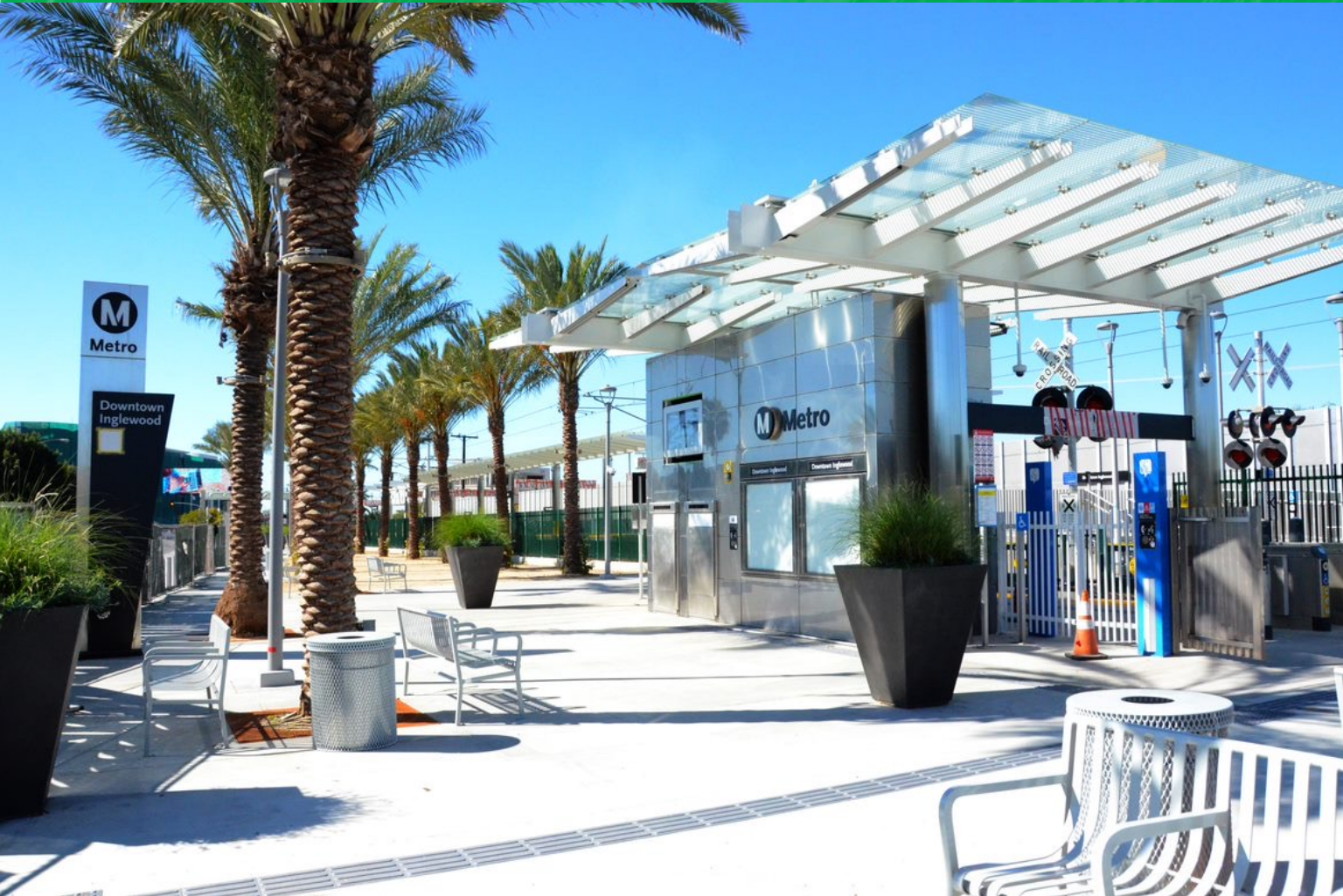
Station pylon, TVM canopy, and plaza
