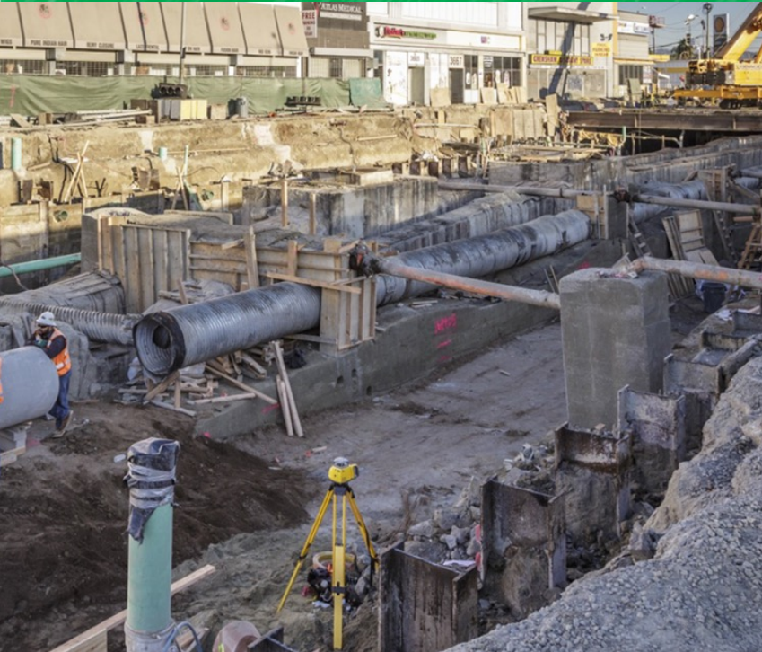
Station backfill and decking removal operation
