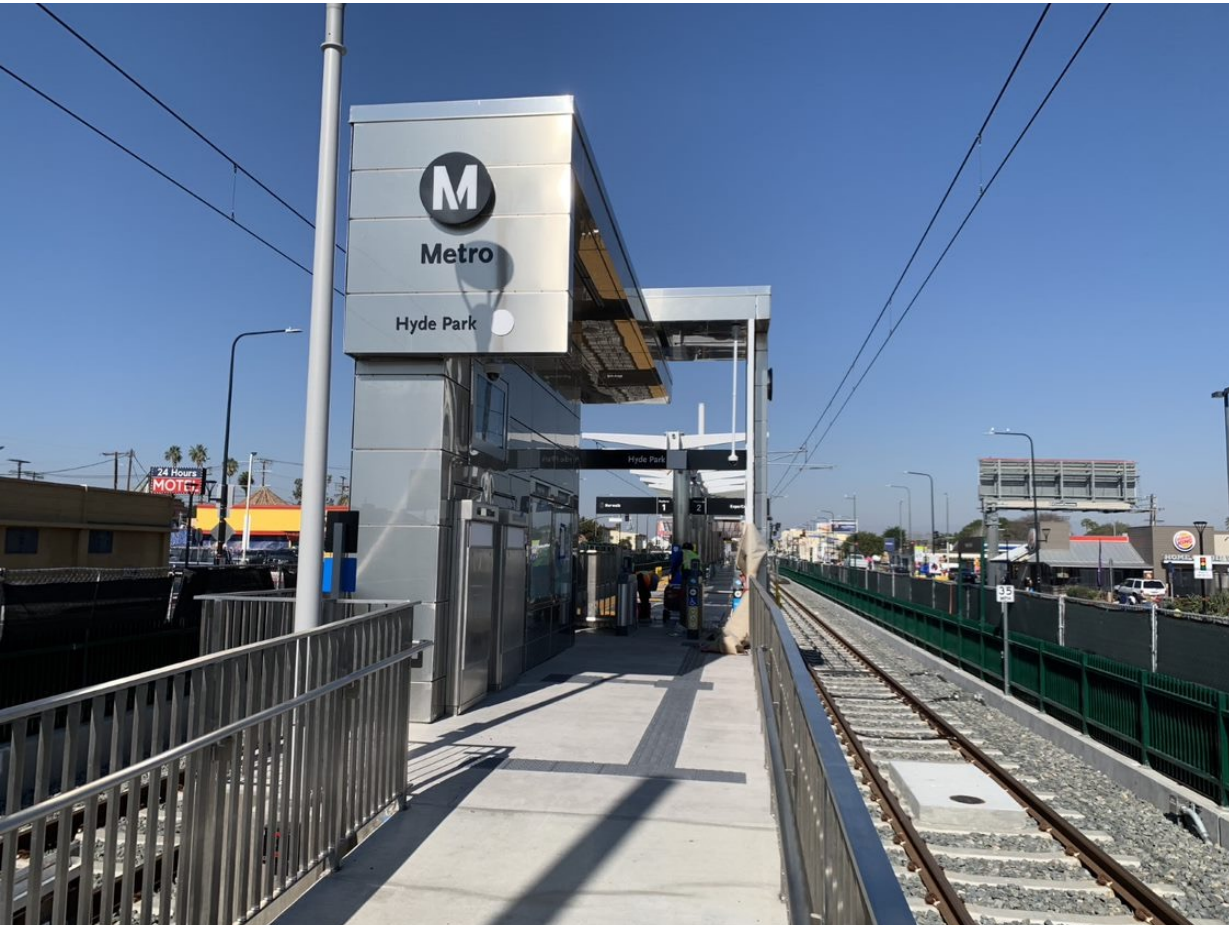
Station platform at Crenshaw Bl near 58th St
