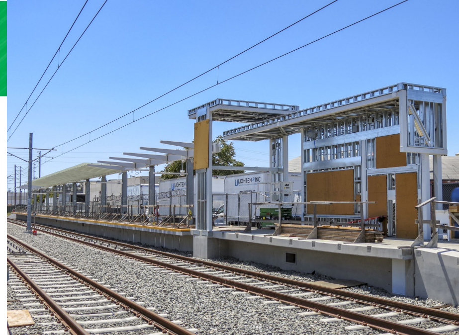
TVM canopy under construction
