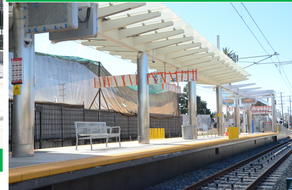
Station platform, benches, and bollards
