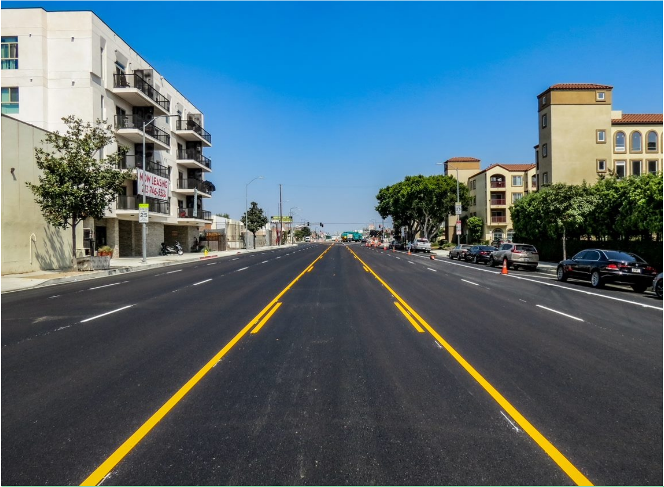
Completed Crenshaw street restoration
