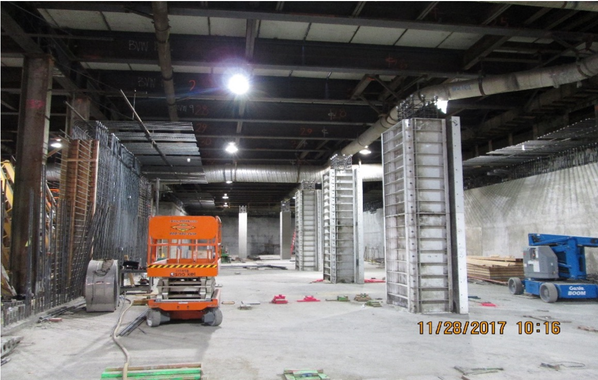
Concourse level frame and rebar installation
