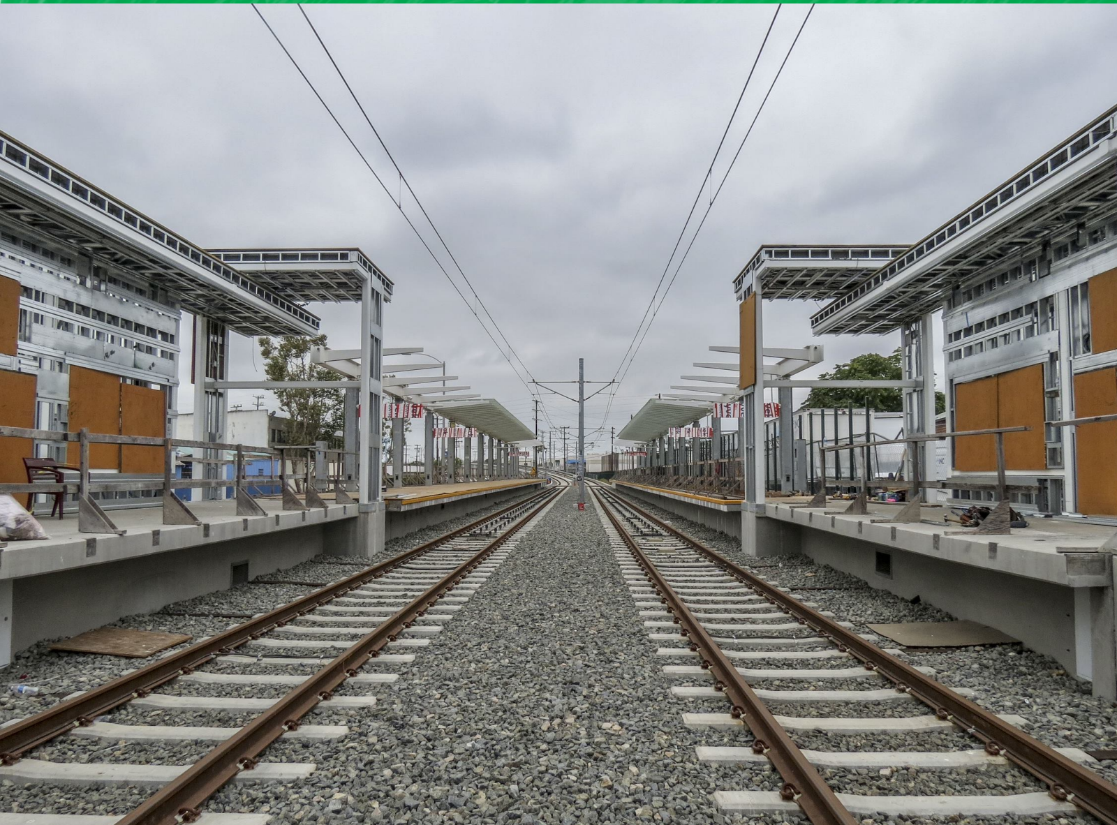
Split-platform station under construction
