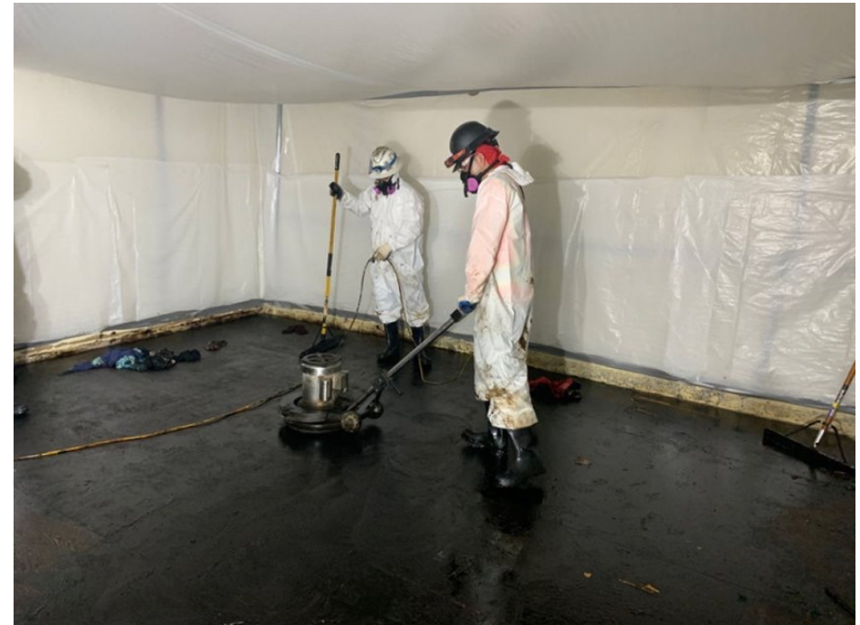
Workers removing glue that held flooring
