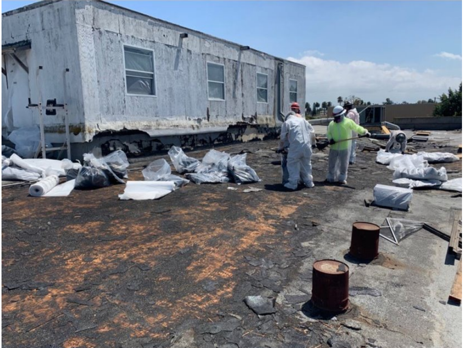
Abatement of roofing material
