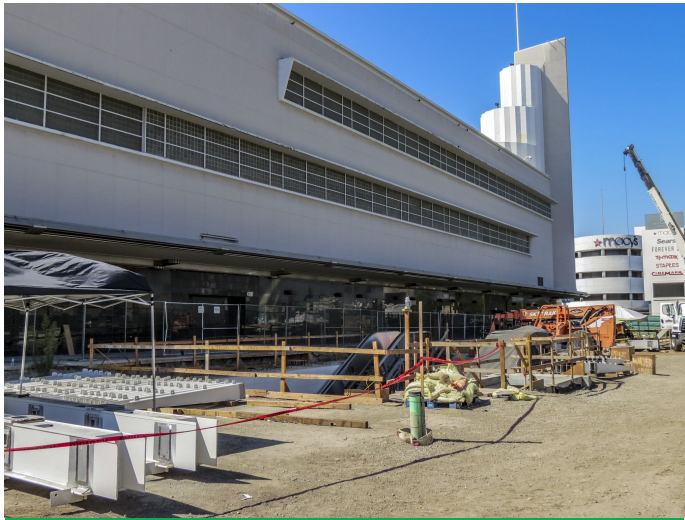
Station plaza construction
