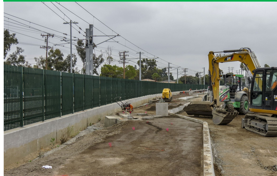
Bus Transfer Facility under construction
