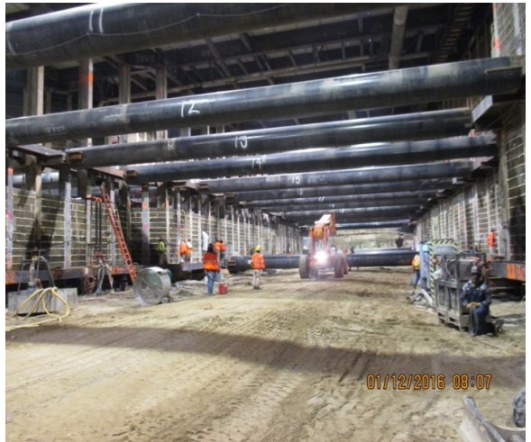
Tier level 2 bracing
