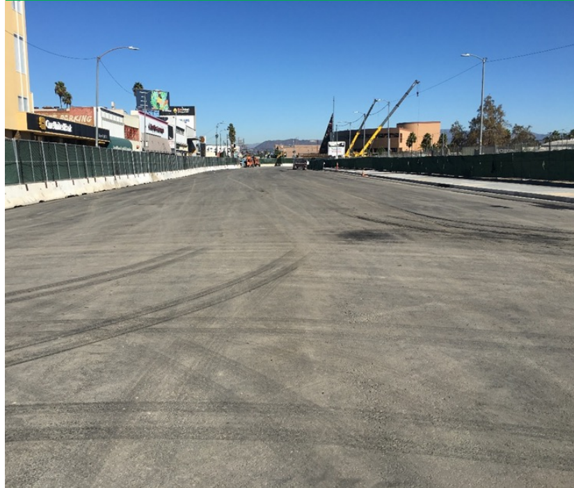
Street restoration of Crenshaw Bl
