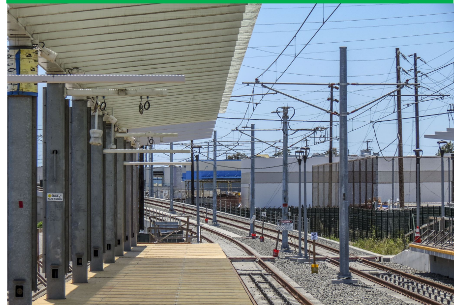
Station platform under construction
