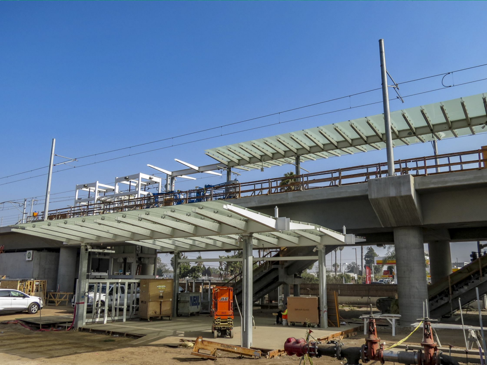
Station canopy and station plaza under construction
