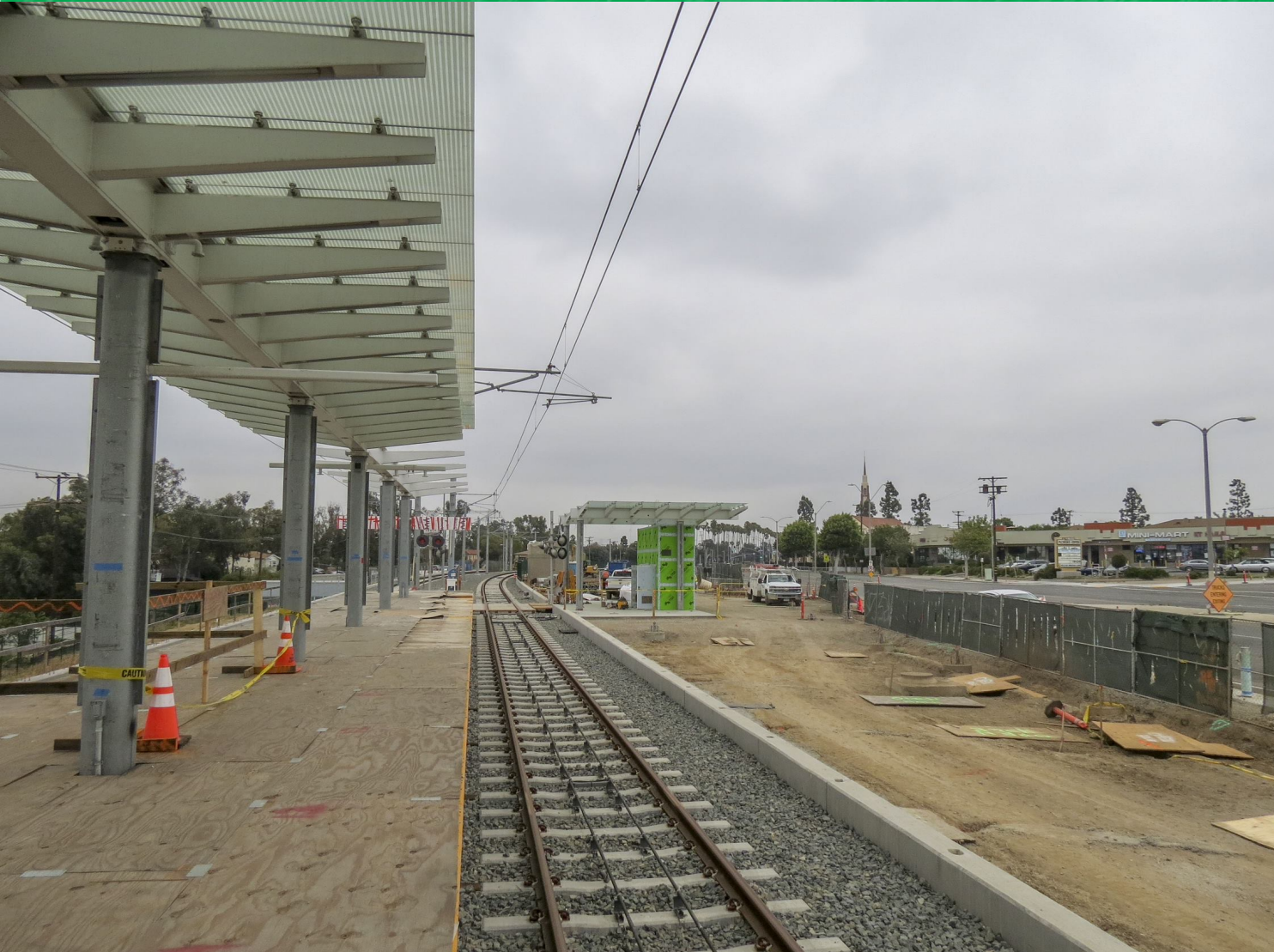
Station platform and plaza under construction
