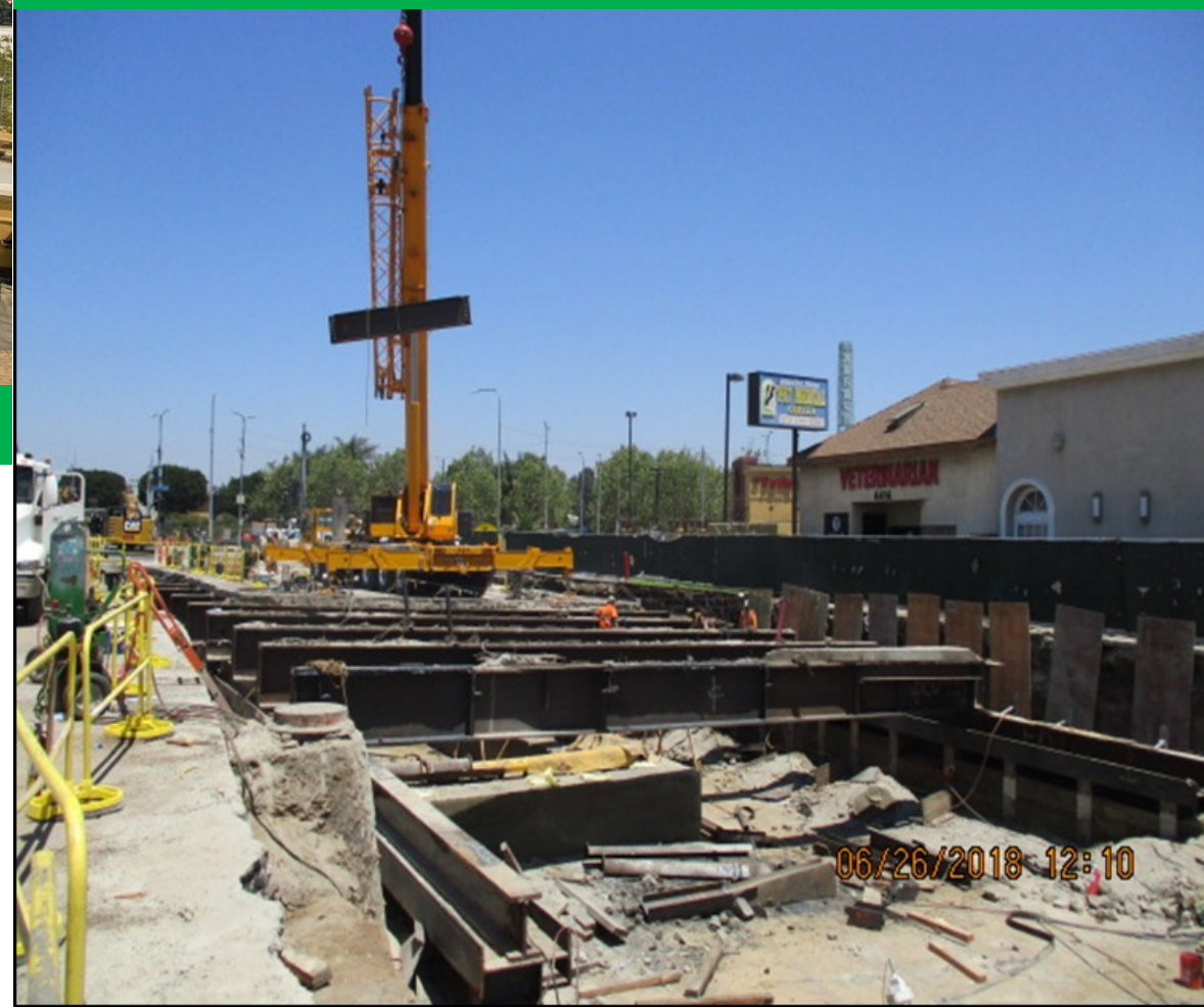
Removal of steel beams during backfilling operation
