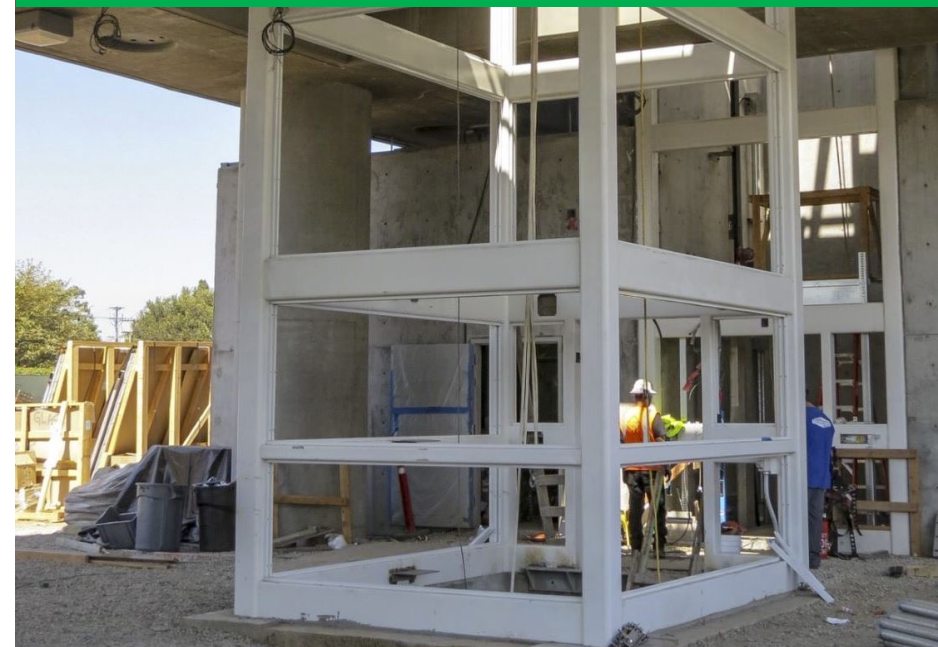
Elevator under construction
