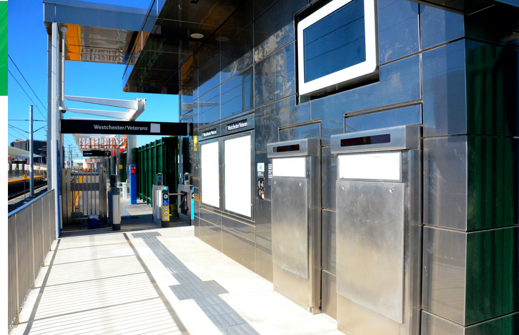
Platform entrance and Ticket Vending Machine
