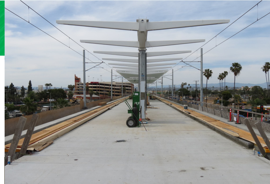
Station platform under construction
