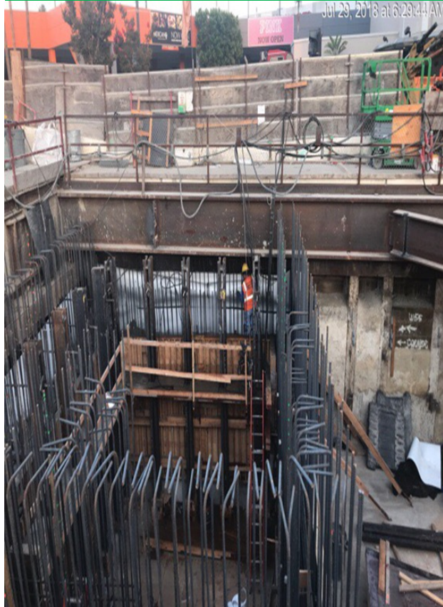
Rebar installation for elevator shaft
