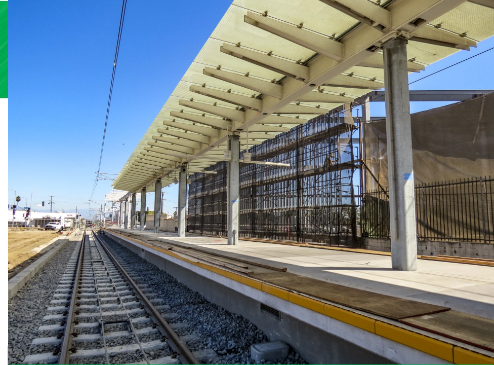
Station platform under construction
