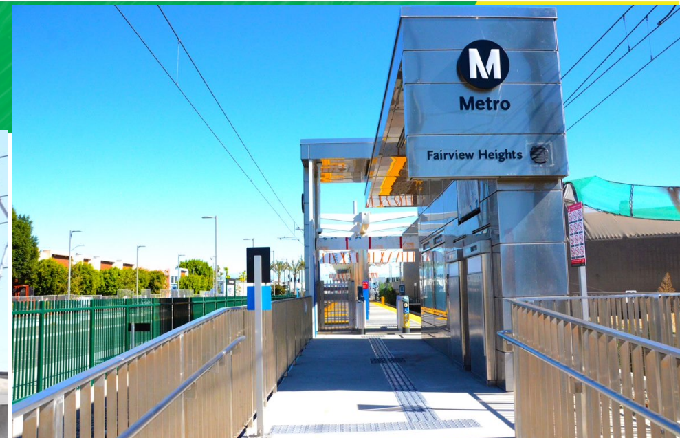
TVM canopy at western end of station
