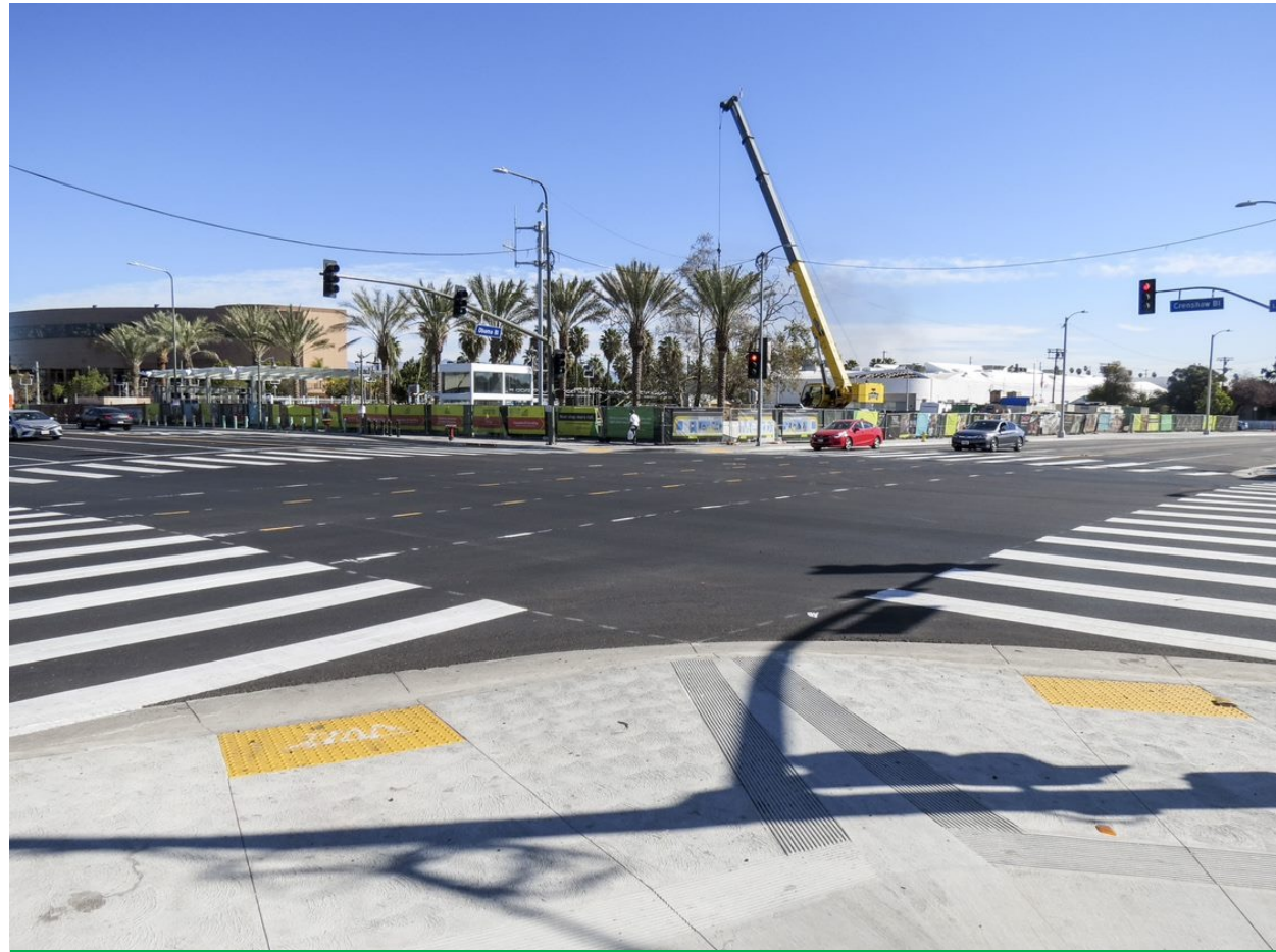
Street restoration at Crenshaw Bl and Obama Bl
