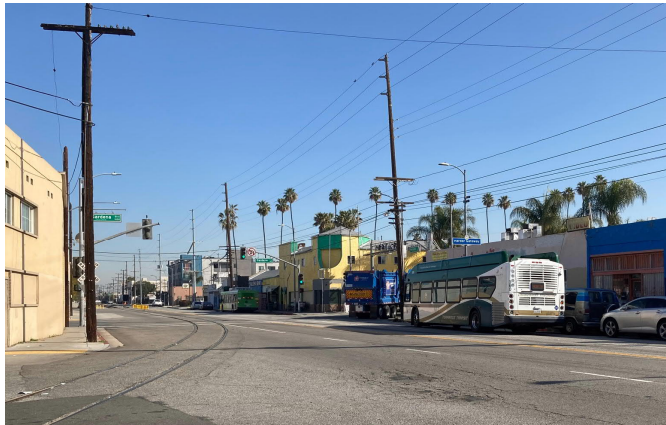
Gardena Blvd & UPRR Track Narrowest roadway width
