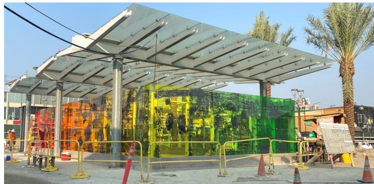
Pavilion art glass panels at station plaza
