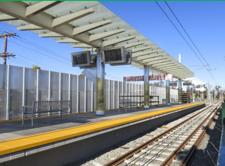
Station platform and tactile pavers
