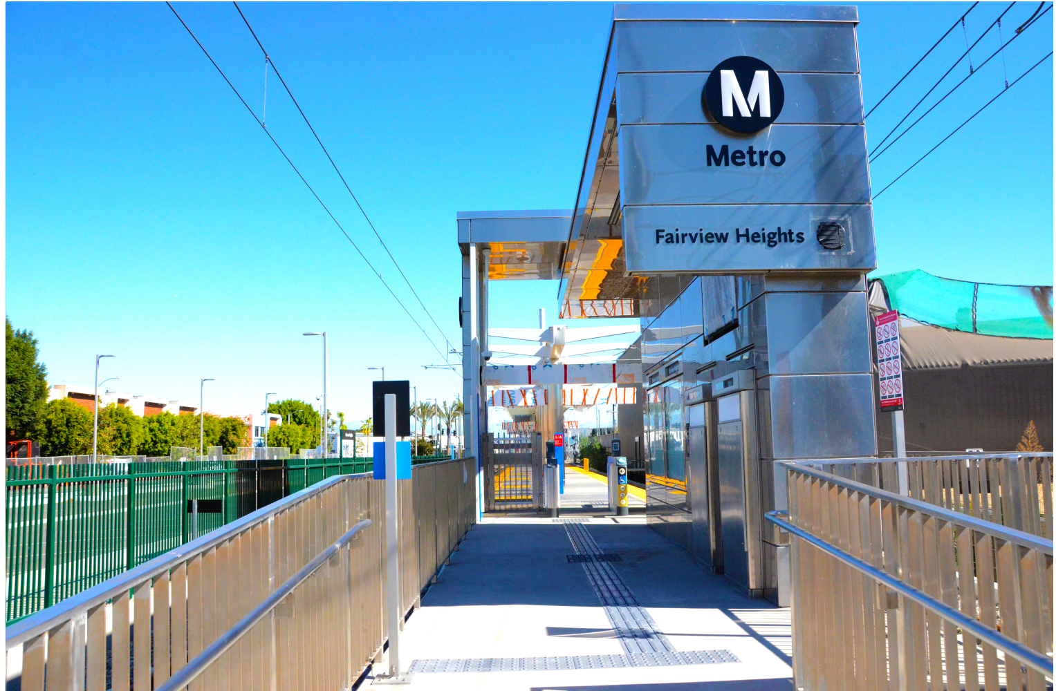
Platform entrance and Ticket Vending Machine canopy
