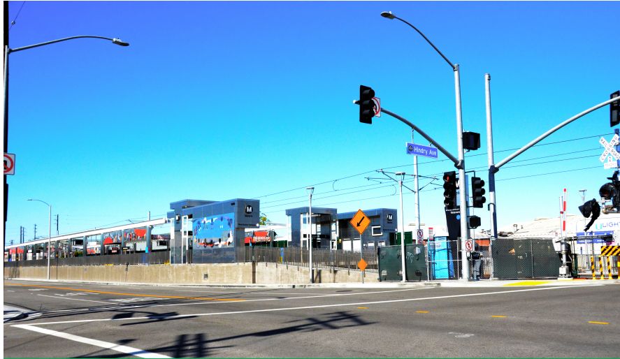
Station view from street
