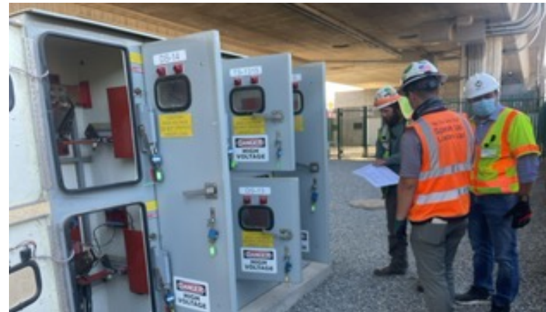
Remaining items walk for Traction Power Substations
