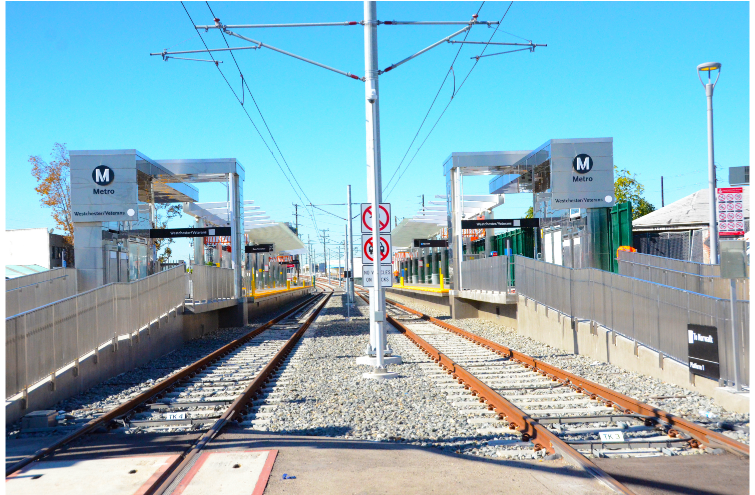
Entrances, OCS, and railway track
