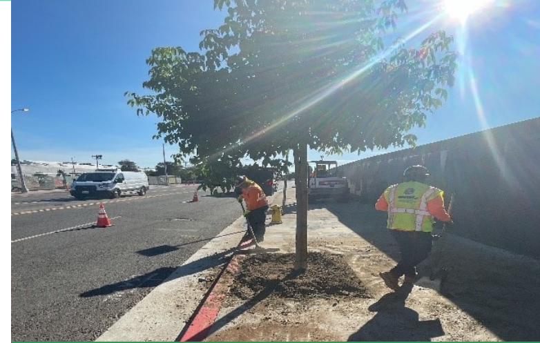
Unloading and planting trees along eastbound Obama Bl and Crenshaw Bl
