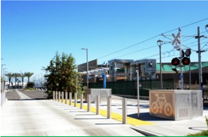
Walkway, bike locker, and tactile pavers
