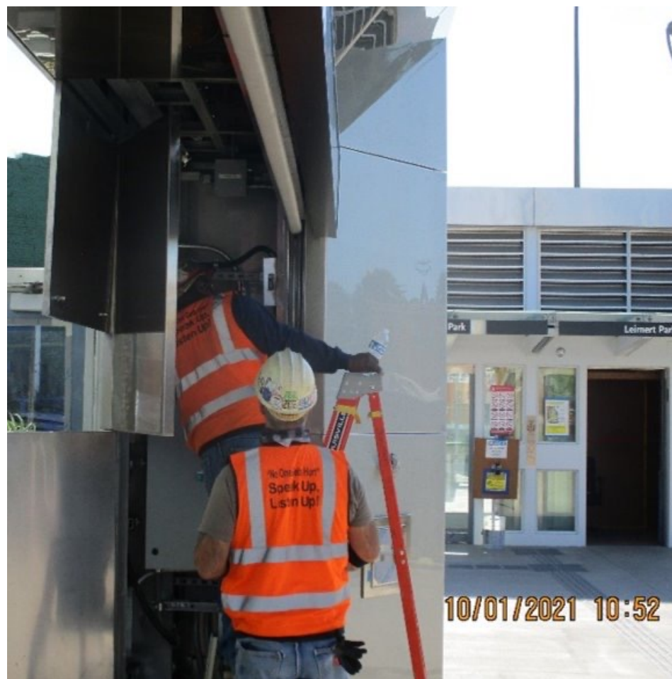
Installation of sensor mounts to the main entrance roll-up door at the station plaza
