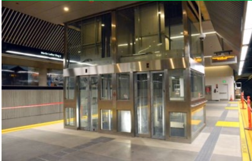
Underground station elevator
