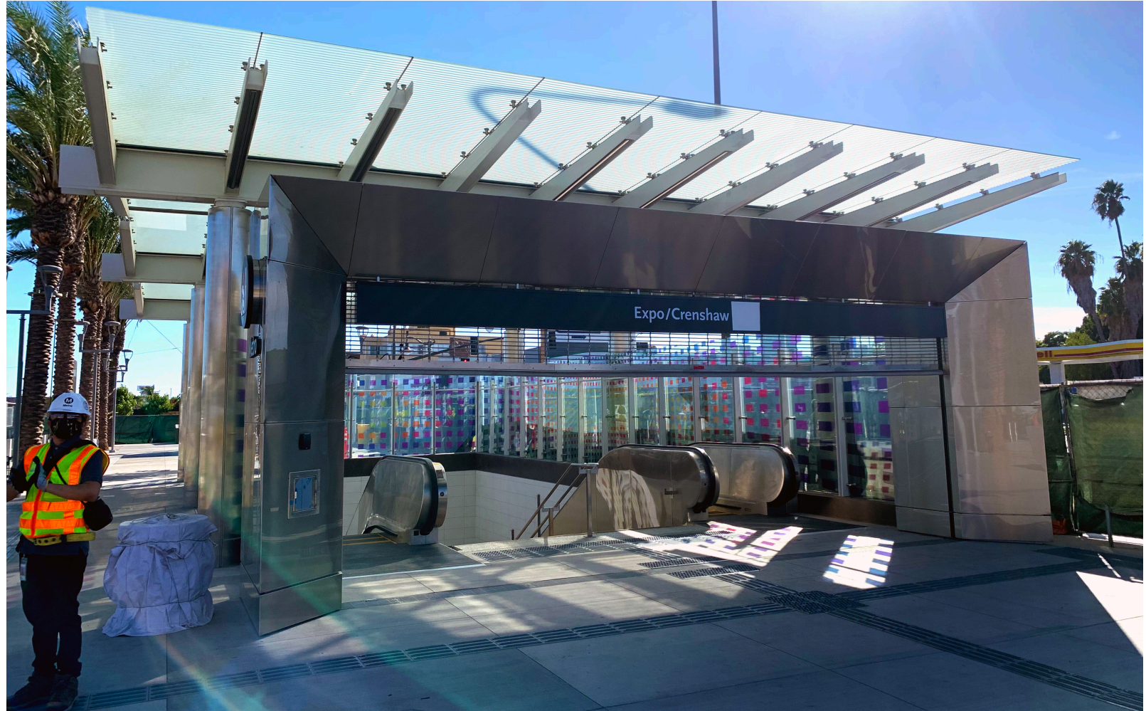
Station entrance stairs and escalators
