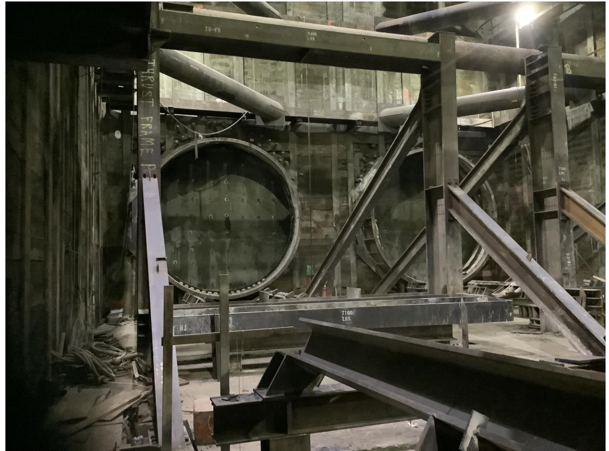
Progress of installing exterior walls.
