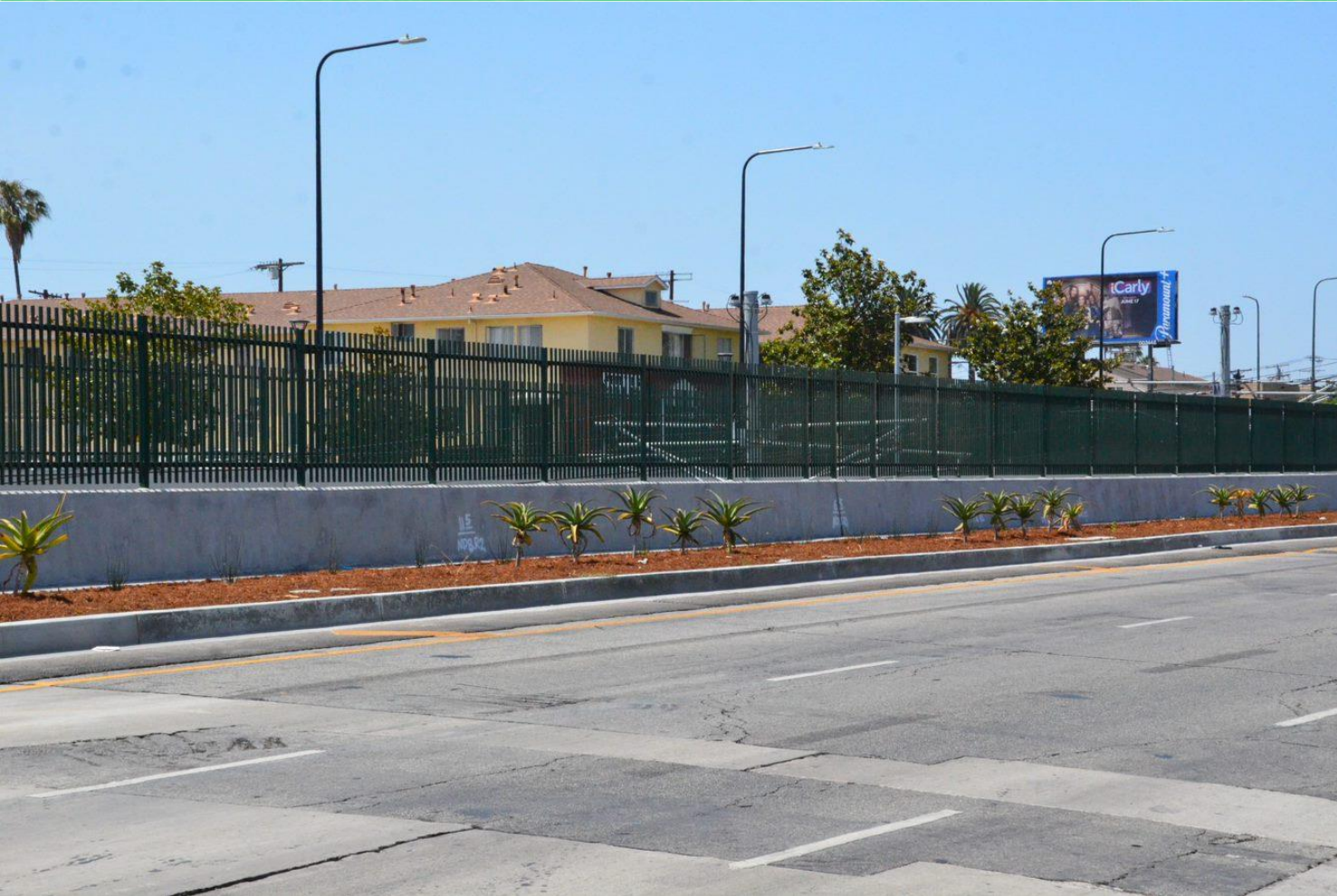
Landscaping at train portal along northbound Crenshaw Bl near 60th St
