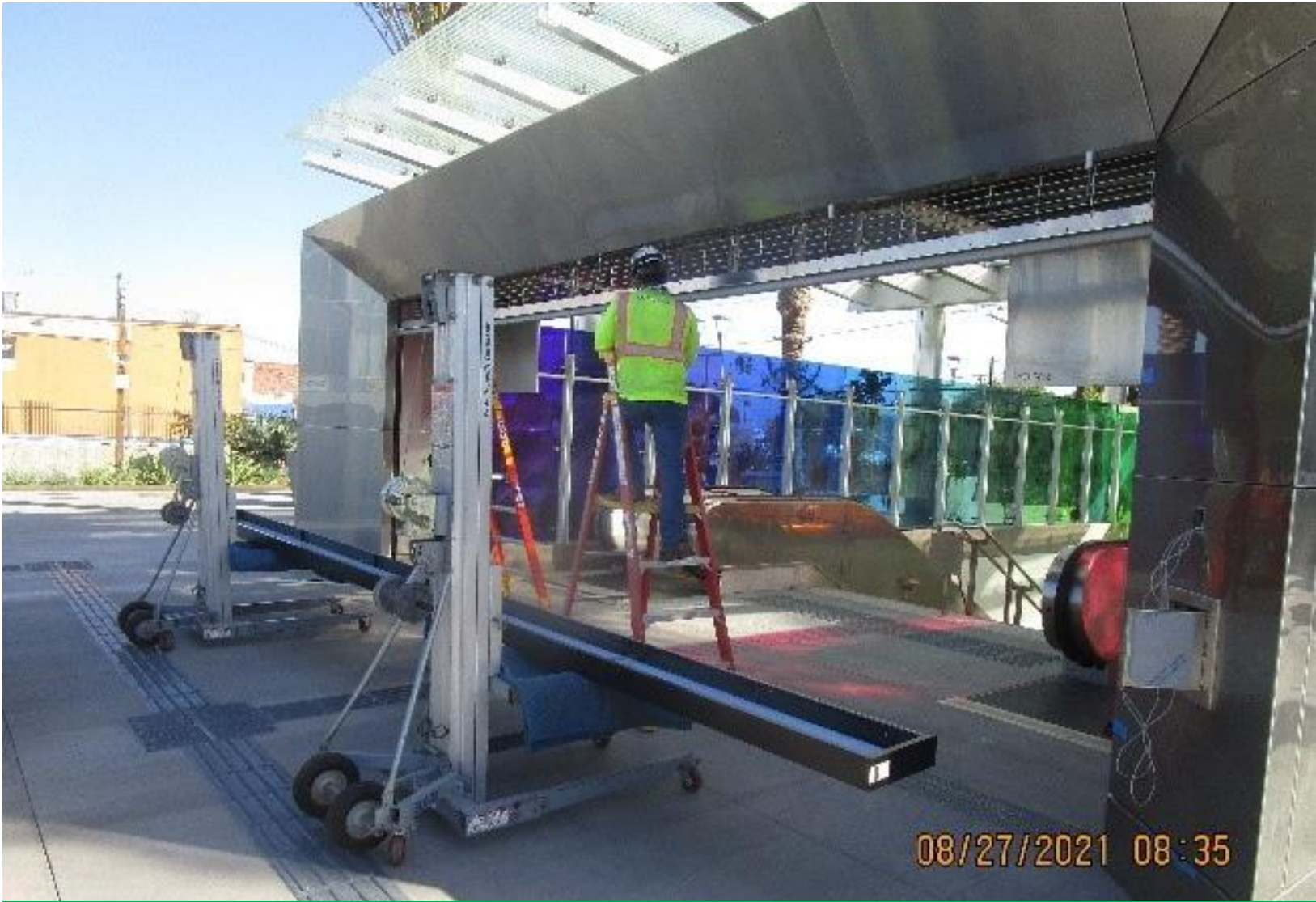
LEIMERT PARK STATION – Preparing for signal band installation above the main entrance coiling door at the plaza
