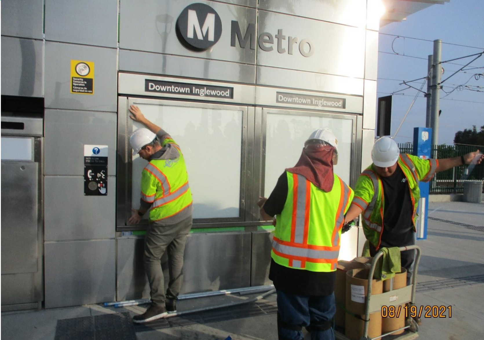
Applying the anti-graffiti coating to the edges of the map cases at the La Brea Station
