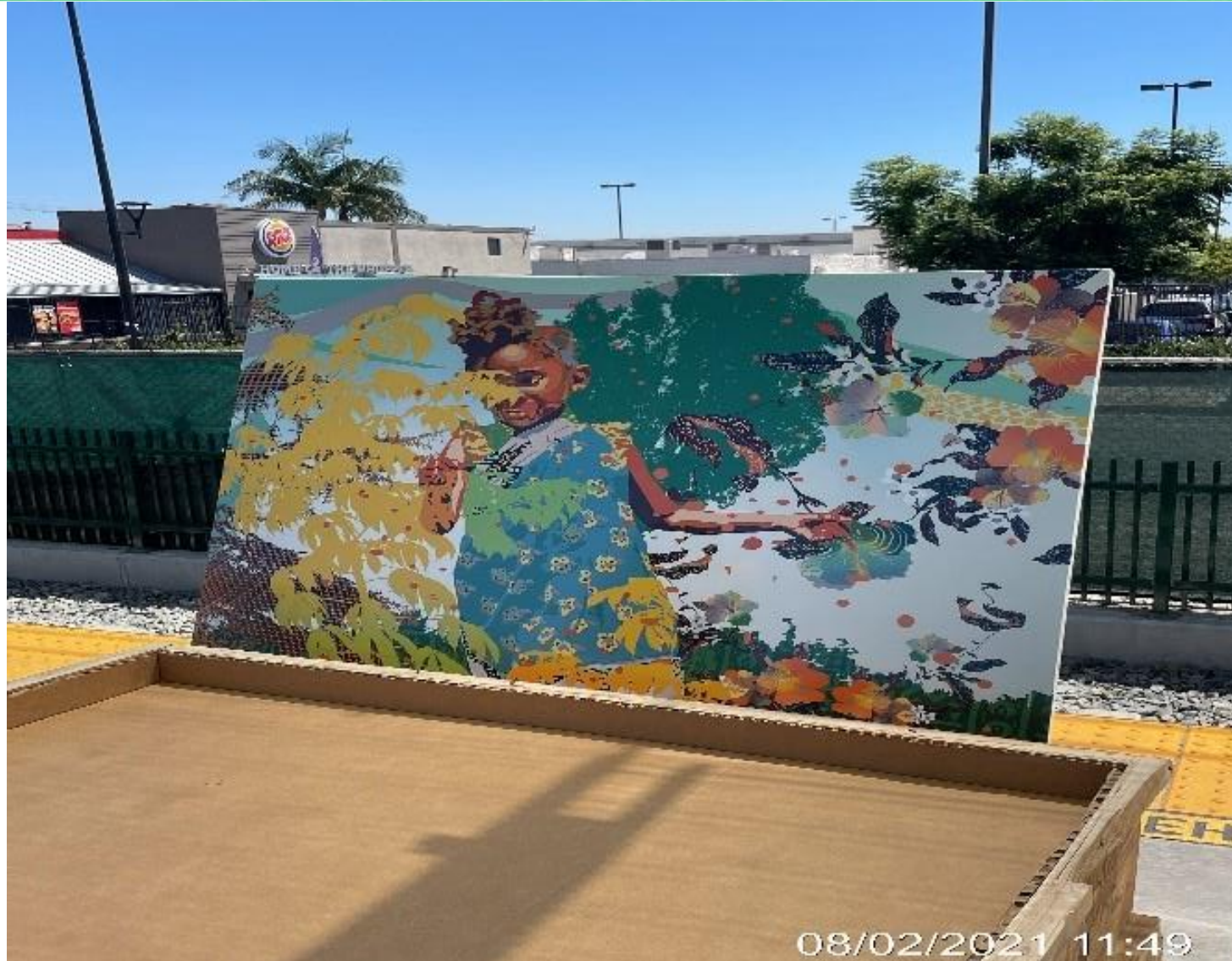
HYDE PARK STATION – Porcelain enamel steel art panel being prepared for installation
