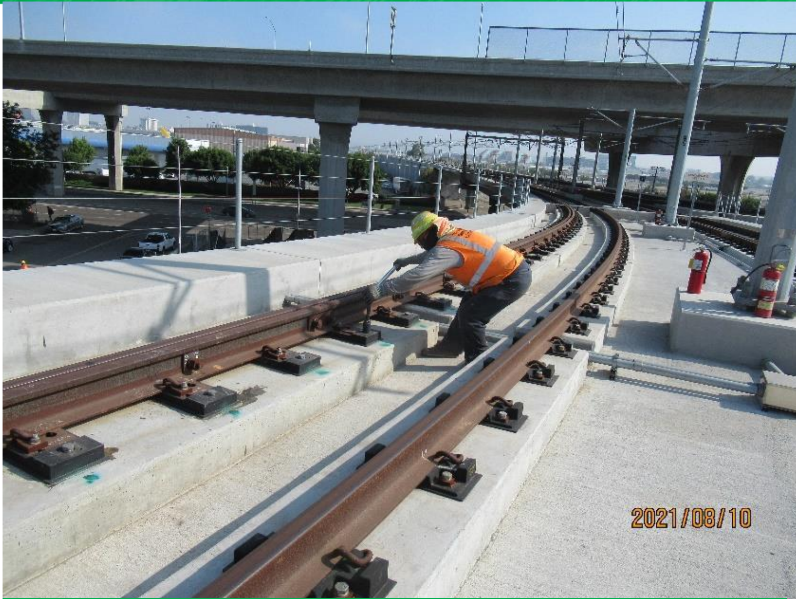
Green Line Bridge Checking Fastener Bolt Torque
