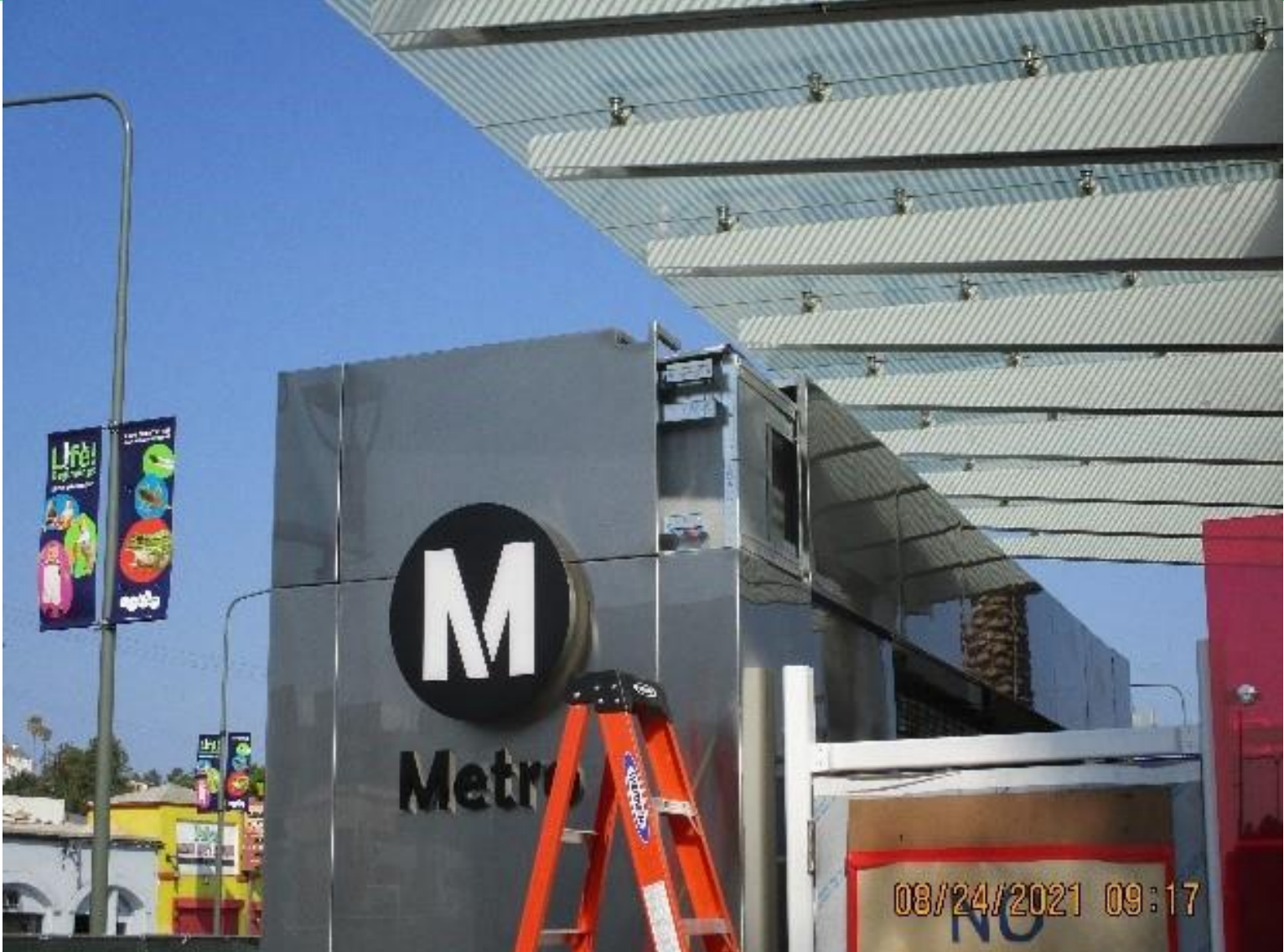
LEIMERT PARK STATION – Resume stainless steel cladding panel installation at the main entrance plaza roll-up door
