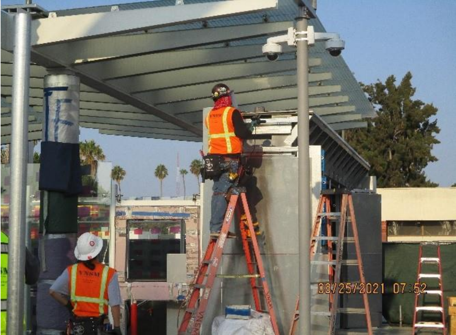
EXPO STATION – Continue stainless steel cladding panel installation to the main entrance plaza roll-up door
