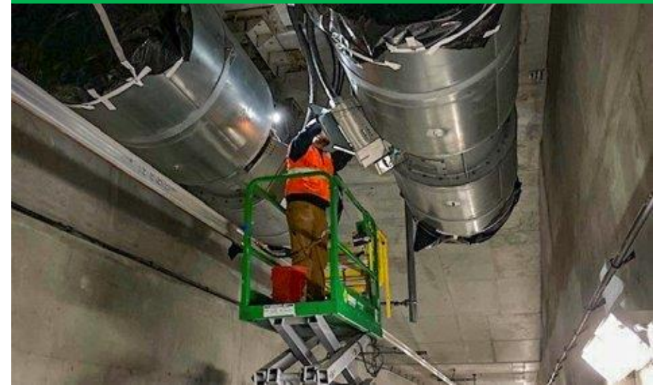
Installation of fans
