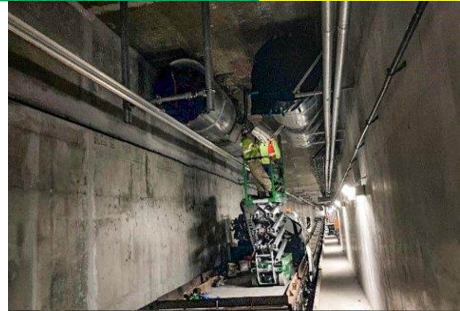
Installation of fans
