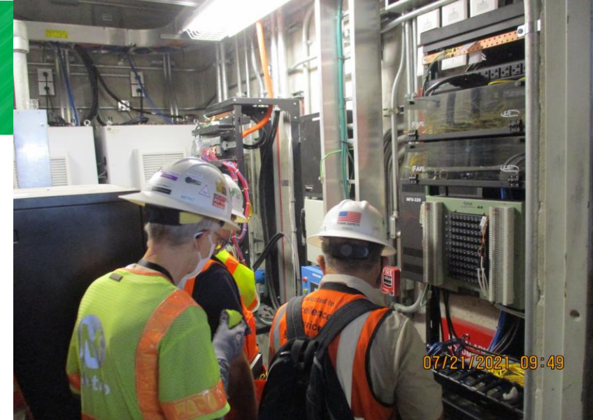
Crews performing system integration testing
