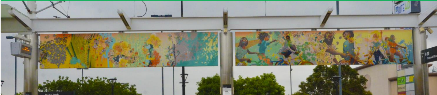
Installed porcelain enamel steel art panels
