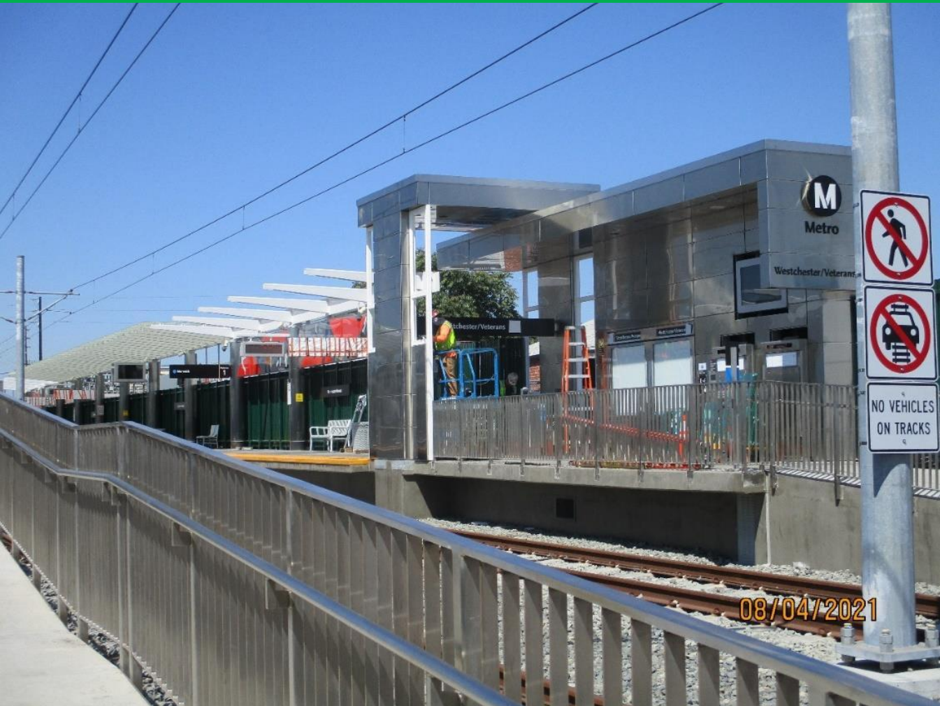
Westchester/Veterans Station wind screen frame mounting
