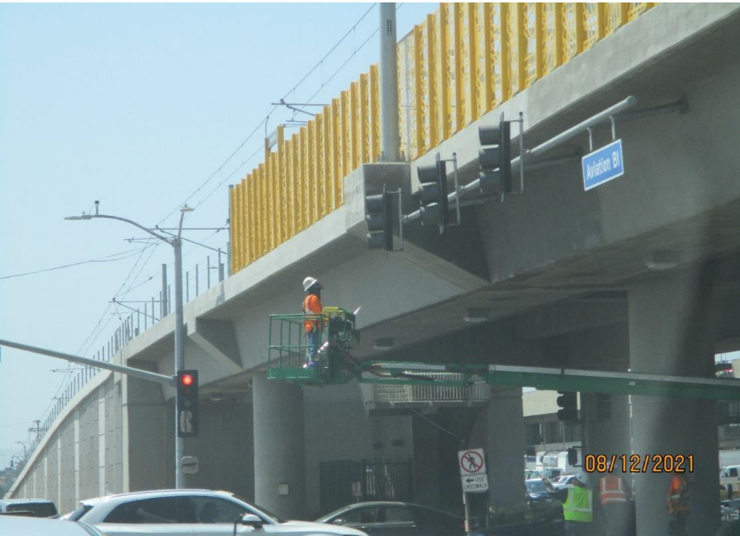
Work crews applying anti-graffiti coating to the Century Bridge
