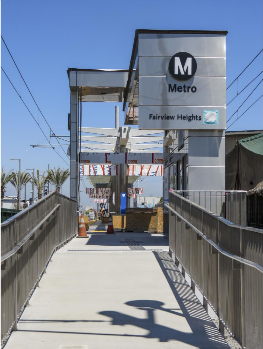
Pedestrian crosswalk, steel bollards, Ticket Vending Machine canopy structure
