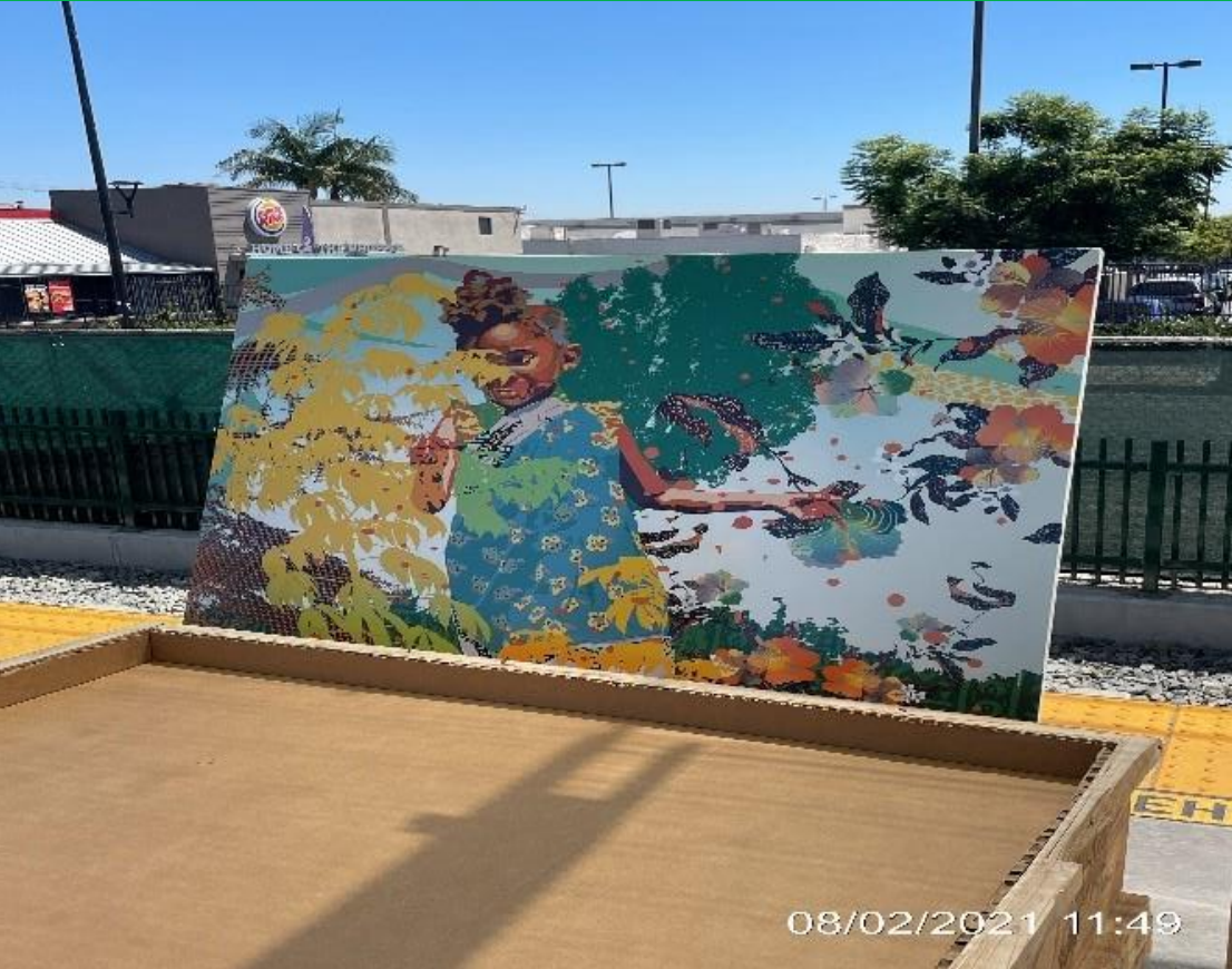
Porcelain enamel steel art panel being prepared for installation
