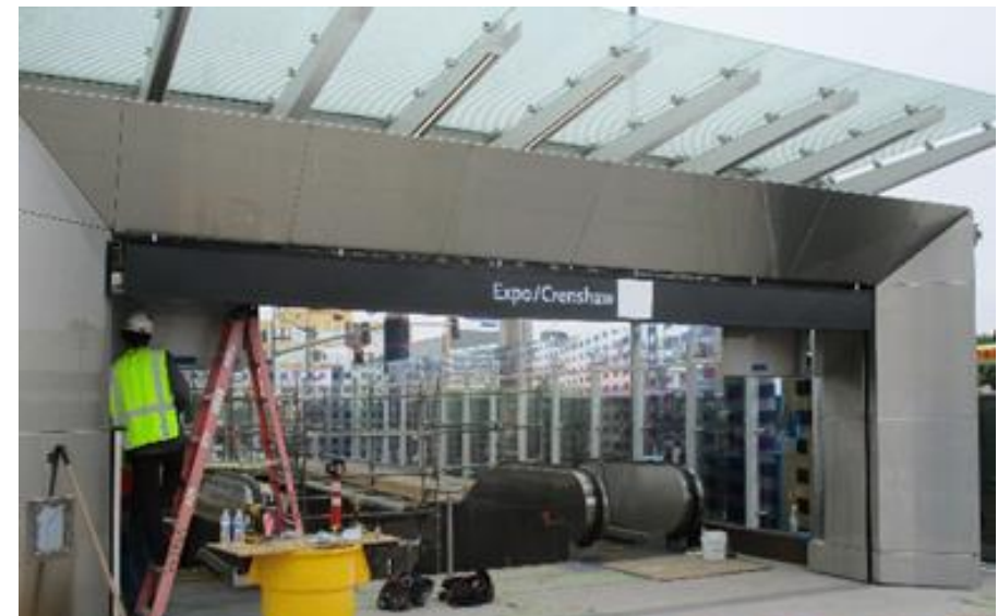
Stainless steel cladding installation for main entrance roll-up door
