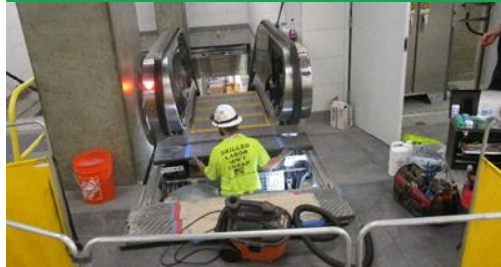
Performing function test on escalators between concourse and platform levels
