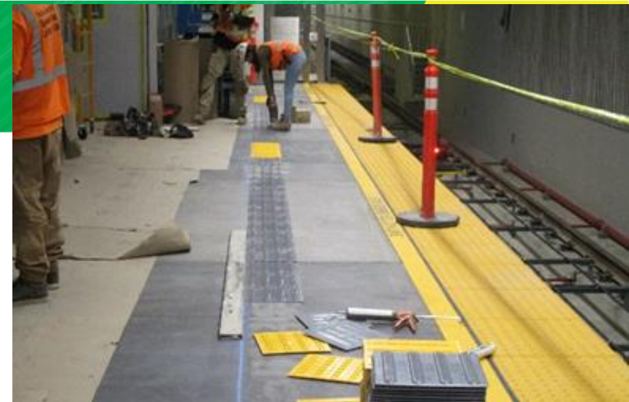
Installing directional tactile pavers throughout the platform
