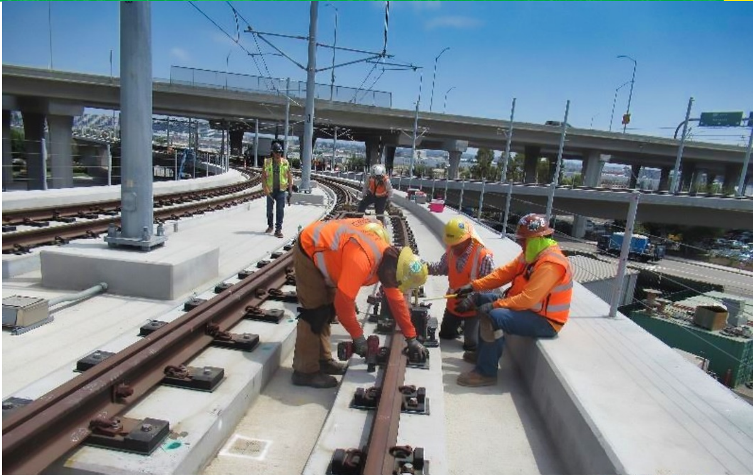
Workers at the C Line/Crenshaw/LAX Wye track adding galvanized shim plates
