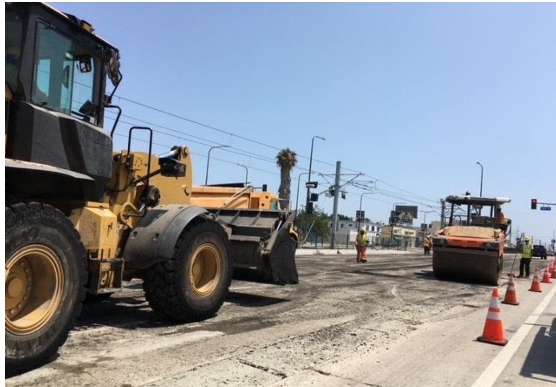
Park Mesa Heights roadway reconstruction along Crenshaw Bl
