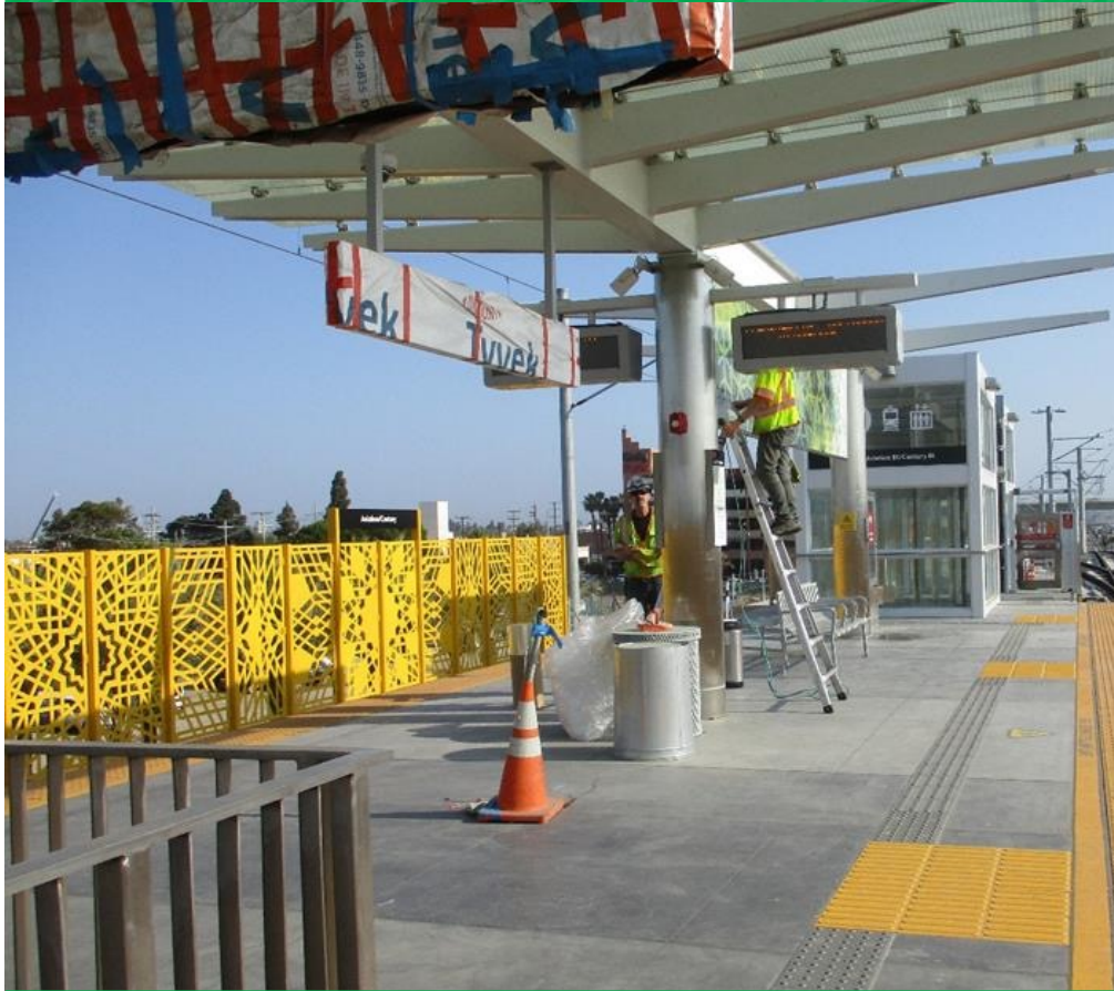
Workers applying the anti-graffiti covering to the Aviation Station Platform columns
